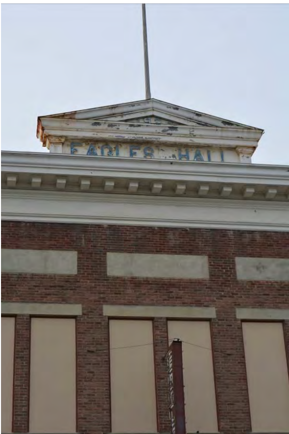
5 of 21. Eagles' Hall, Cornice detail, April 2019
