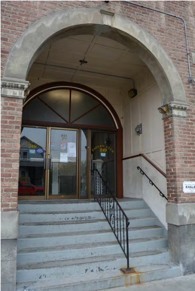
6 of 21. Eagles' Hall, Main entry detail, April 2019
