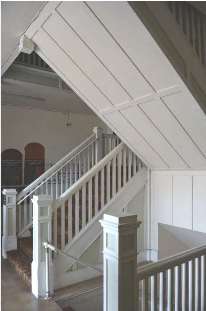
8 of 21. Eagles' Hall, Main entry stair detail, April 2019
