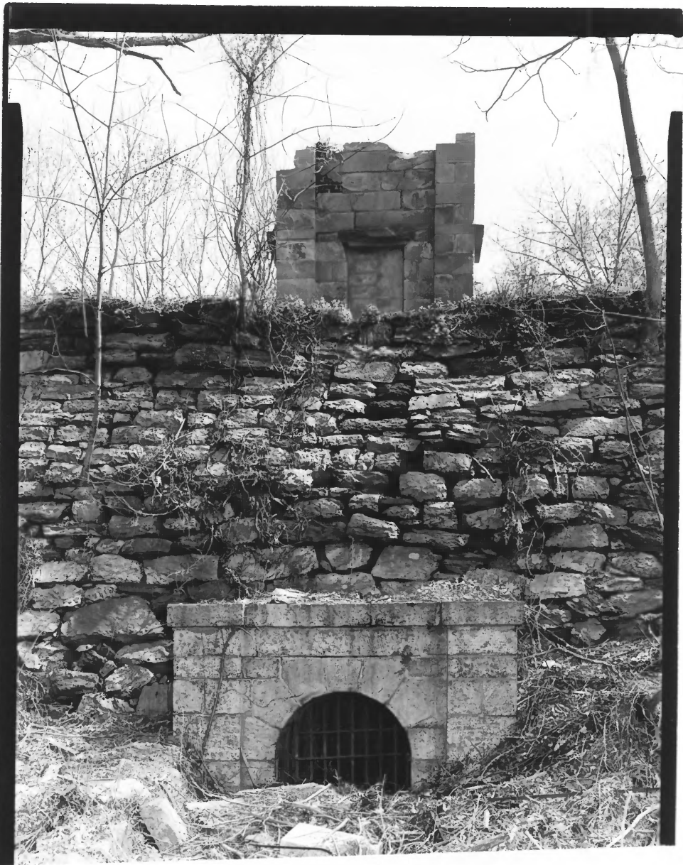
PHOTOGRAPH #9 Croton Aqueduct Ossining, New York Western elevation of the waste weir atop the Aqueduct and its discharge conduit at Snowden Avenue and Van Wyck Street in Ossining. Jack Boucher, 1978, HAER Photo No. NY-109-4.
