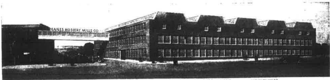
Rendering, Finishing Mill (Building 7), 1938
