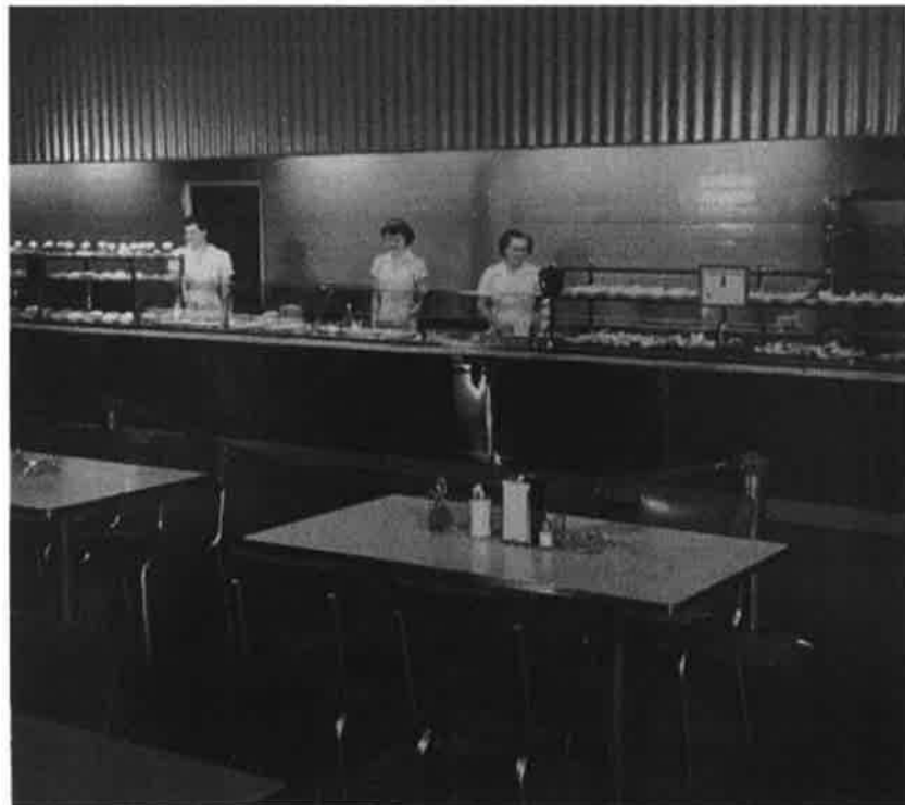
Cafeteria, Possibly Basement of Building 4, Hanes Hosiery Mill, c. 1954 Image courtesy of Frank Hinman, Gateway Holdings
