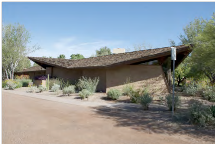
Figure 4. View of O'Connor House facing north. Source: E. Vondy, 2018.
