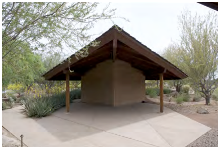
Figure 8. View of O'Connor House facing southeast of the northwest prow roof. Source: E. Vondy, 2018.
