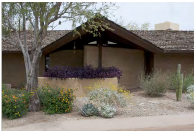
Figure 5. View of O'Connor House facing east towards sheltered entry. Source: E. Vondy, 2018.
