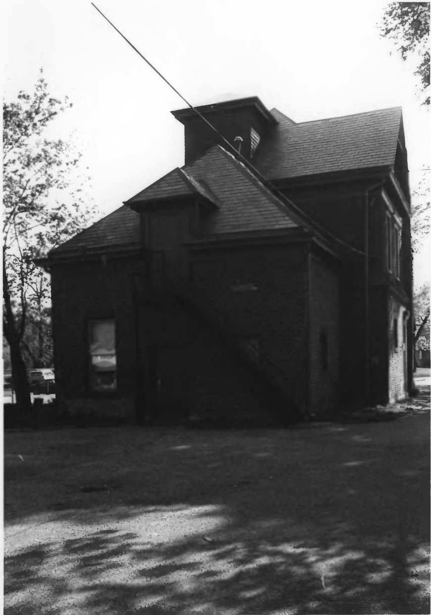
© FIREHOUSE No. 7, E. BANK, IN, SO. BEND, IN PHOTO No. 6C
