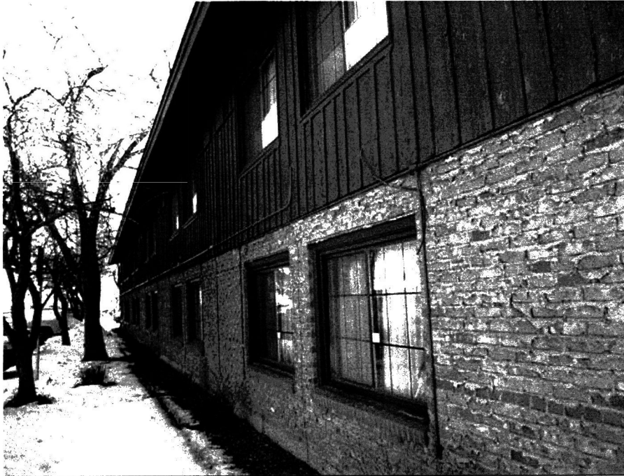
Photo 0011. North elevation of north wing of Dude Rancher Lodge. View to the east.
