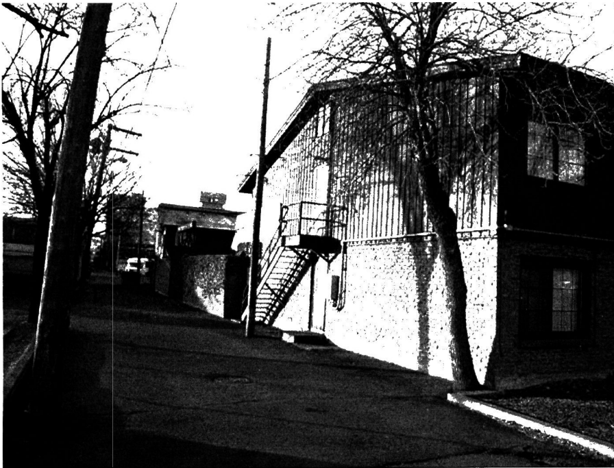
Photo 0009. Rear façade of north wing at Dude Rancher Lodge. View to the south.
