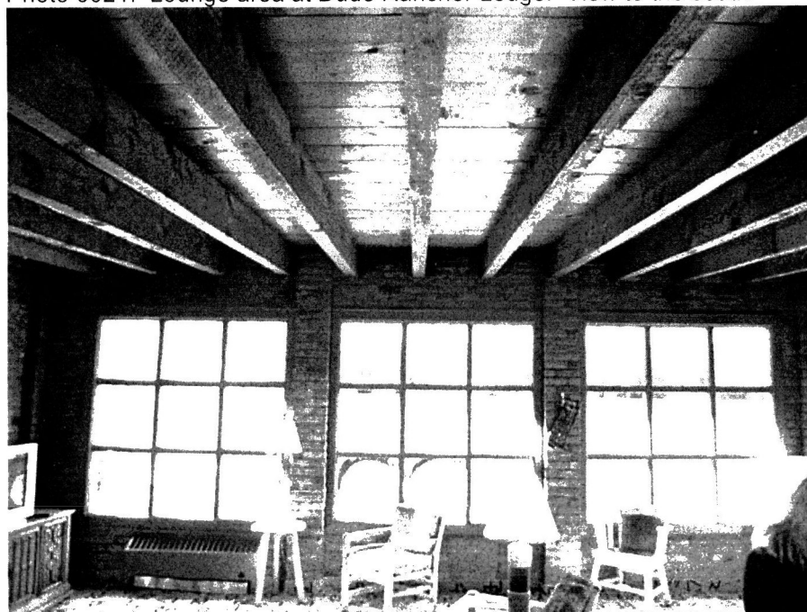
Photo 0022. Lounge area at Dude Rancher Lodge. View to the west.
