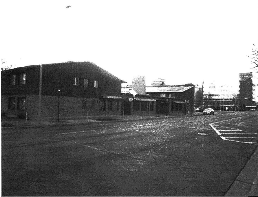
Photo 0001. Overview of Dude Rancher Lodge. View to the southeast.
