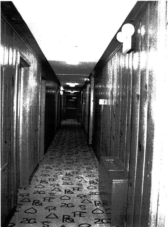
Photo 0026. Second floor hallway in south wing of Dude Rancher Lodge. View to the east.
