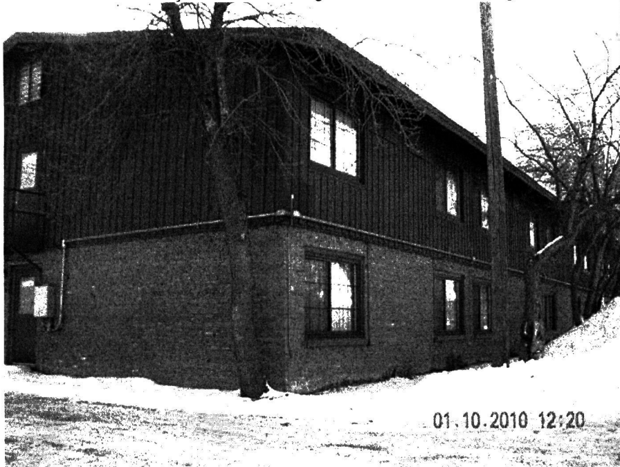
Photo 0010. North elevation of north wing of Dude Rancher Lodge. View to the southeast.
