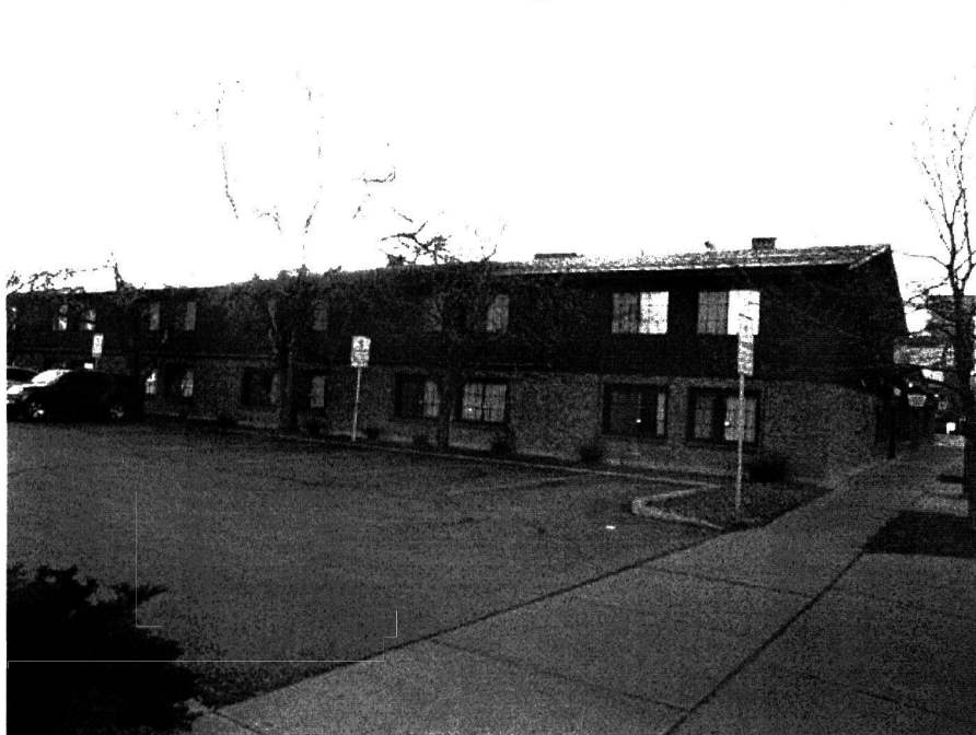
Photo 0012. North elevation of north wing of Dude Rancher Lodge. View to the south.
