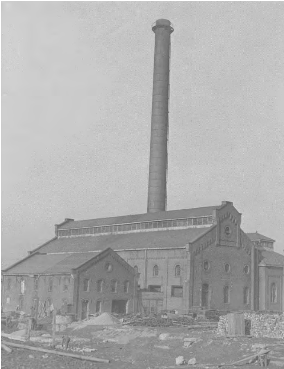
Figure 4: Original generation plant, boiler house, 1936. Columbus Metropolitan Library.
