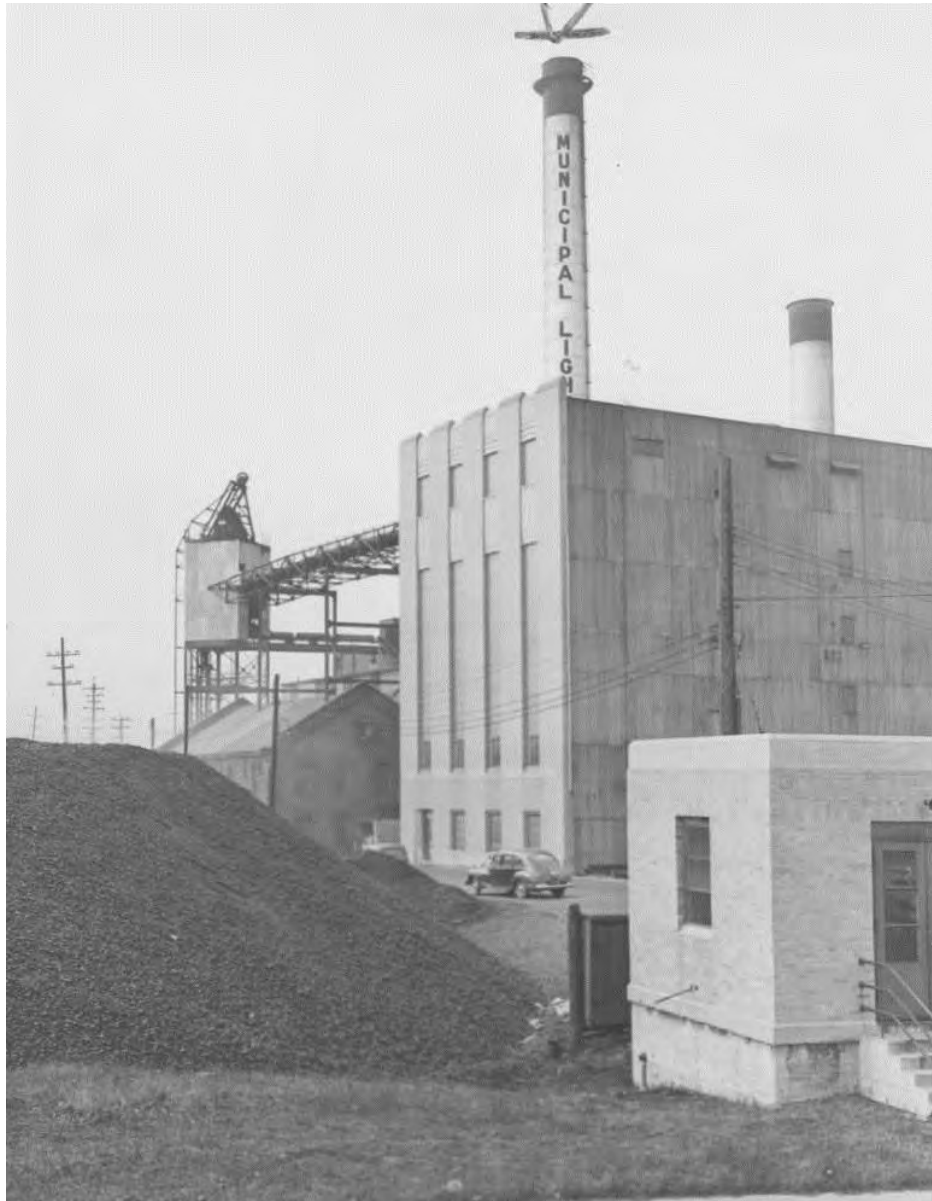
Figure 5: New generation plant, 1946. Columbus Metropolitan Library.
