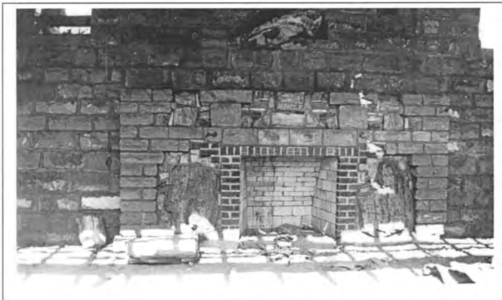
H4. Fireplace with petrified wood under construction. ca. 1936
