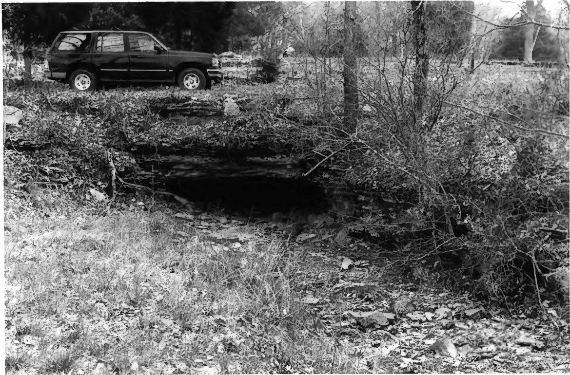
CHANDLER STONE WALL WILSON COUNTY
