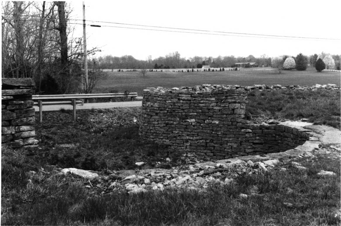
CHANDLER STONE WALL WILSON COUNTY
