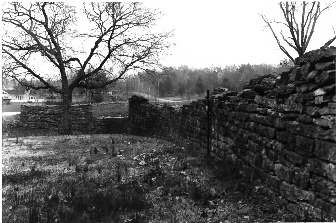
CHANDLER STONE WALL WILSON COUNTY
