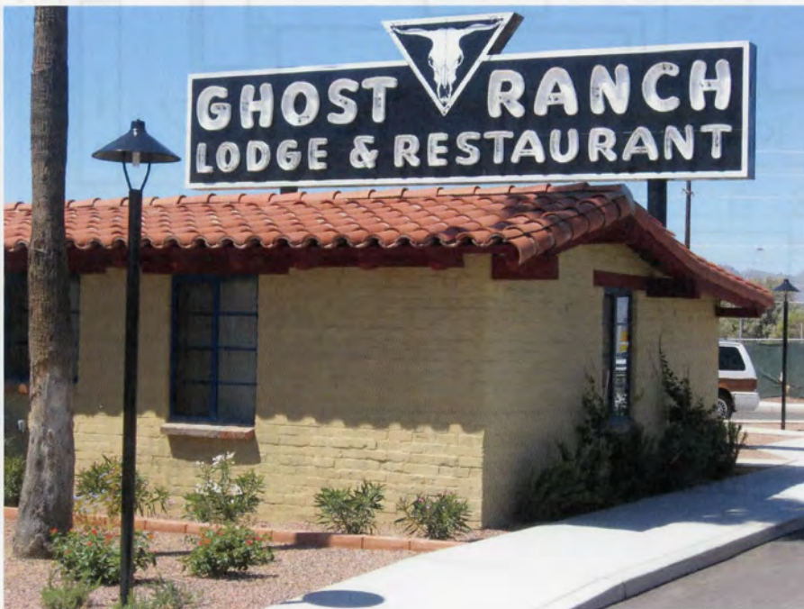
2. Original Building Group Rehabilitated sign relocated to Office Q. View to southwest. (Photo by Paul C. Sikorski of Ryden Architects, Inc., 2010)
