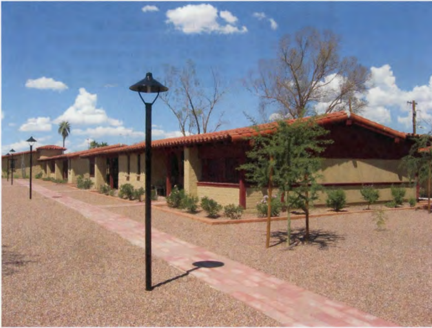
9. Original Building Group Building D and C. View to northeast. (Photo by Paul C. Sikorski of Ryden Architects, Inc., 2010)
