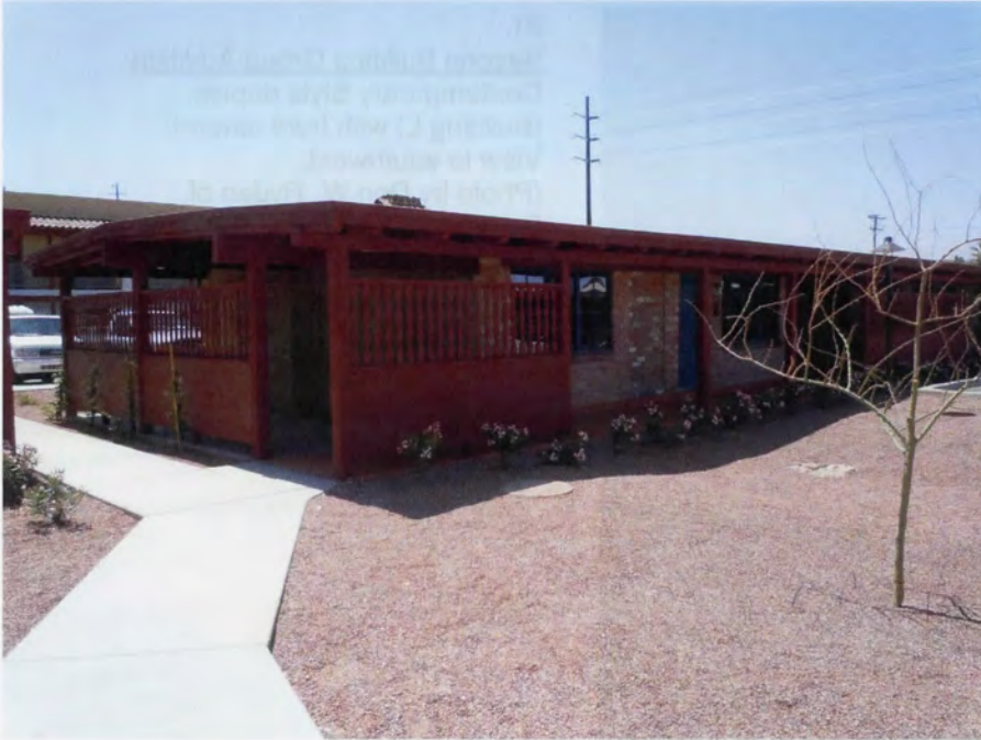
19. First Building Group Addition Spanish Colonial Ranch Style linear units (Building J) with covered walkway and end carports. View to southwest. (Photo by Don W. Ryden of Ryden Architects, Inc., 2011)
