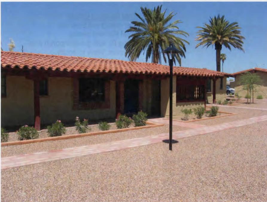
14. Original Building Group Rehabilitated Building F. View to northwest. (Photo by Don W. Ryden of Ryden Architects, Inc., 2011)
