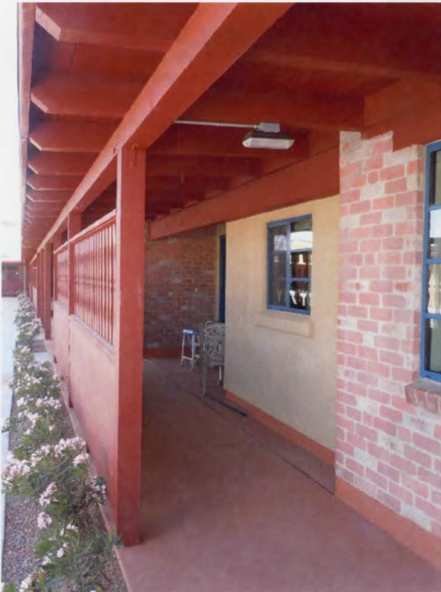
20. First Building Group Addition Building K carport infill retains sense of space and original grilles. View to south. (Photo by Don W. Ryden of Ryden Architects, Inc., 2011)
