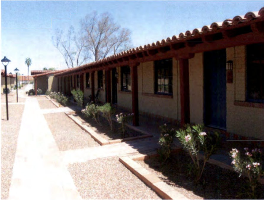
17. First Building Group Addition Spanish Colonial Ranch Style linear units (Building A) with covered walkway and no carports. View to northeast. (Photo by Paul C. Sikorski of Ryden Architects, Inc., 2010)
