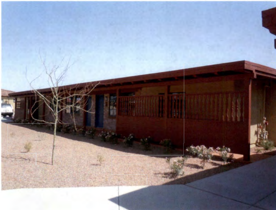
18. First Building Group Addition Spanish Colonial Ranch Style linear units (Building I) with covered walkway and end carports. View to southeast. (Photo by Don W. Ryden of Ryden Architects, Inc., 2011)
