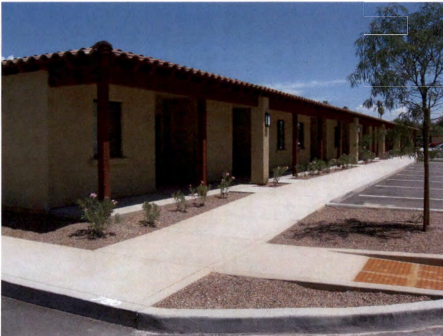
31. Fourth Building Group Addition The new, one-story Apartment (Building 4) is a simplified interpretation of the Joesler-designed duplexes. View to northeast. (Photo by Don W. Ryden of Ryden Architects, Inc., 2011)
