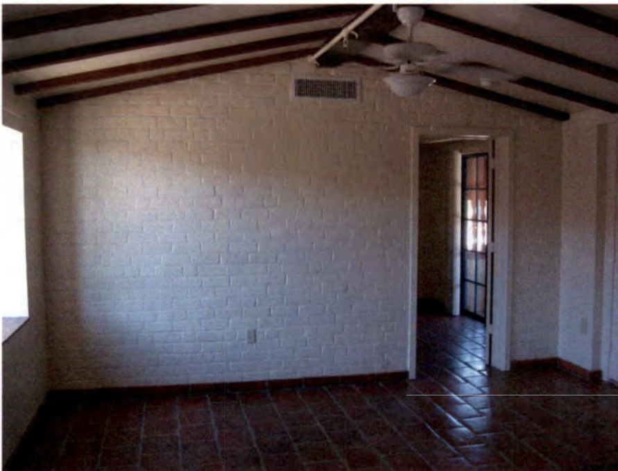
37. Original Building Group Typical livingroom looking into bedroom infill of a carport at a rehabilitated Joesler- designed duplex. Brick wall, roof beams, and tile floors are preserved. (Photo by Don W. Ryden of Ryden Architects, Inc., 2010)
