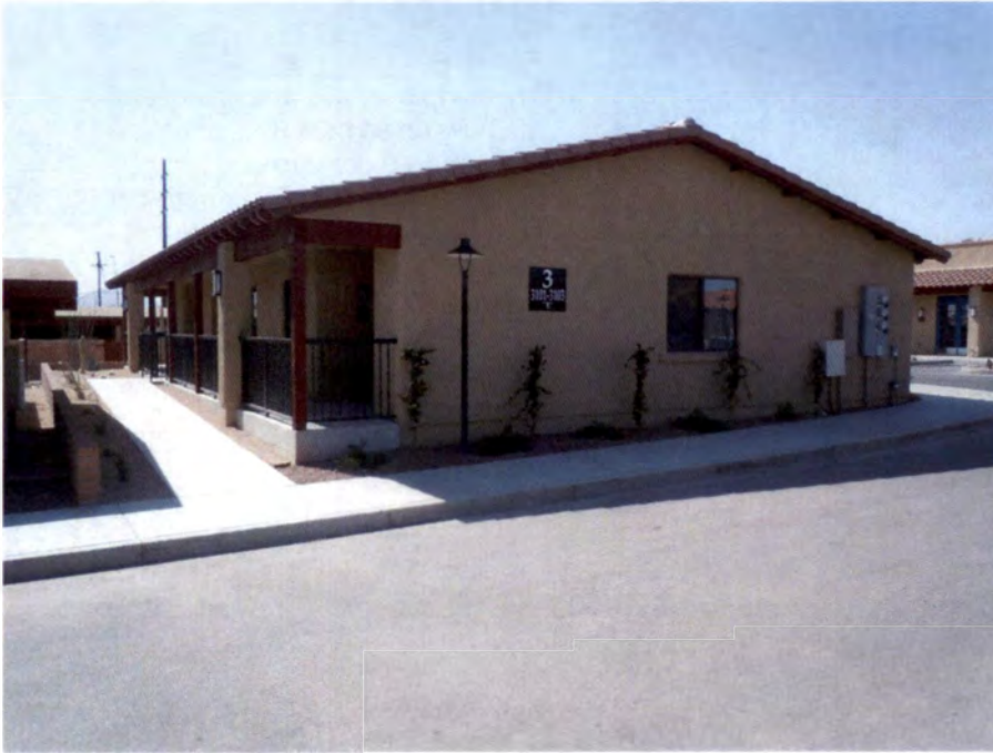
30. Fourth Building Group Addition The new, one-story Apartment (Building 3) is a simplified interpretation of the Joesler-designed duplexes. View to northwest. (Photo by Don W. Ryden of Ryden Architects, Inc., 2011)
