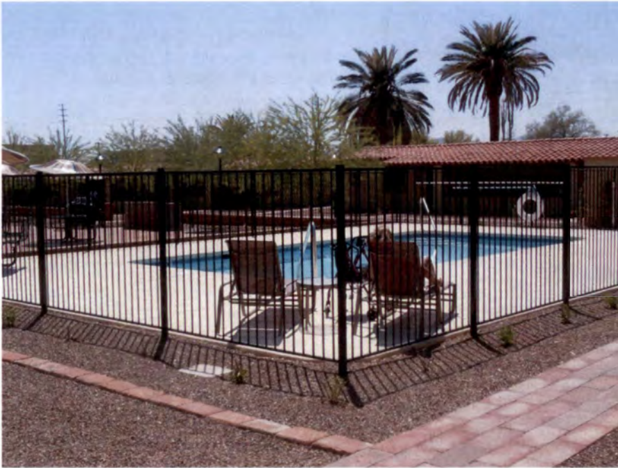
36. Fourth Building Group Addition Located at the north end of Courtyard AA, non-eligible shuffleboard courts have been replaced by a new swimming pool. View to southwest. (Photo by Don W. Ryden of Ryden Architects, Inc., 2011)
