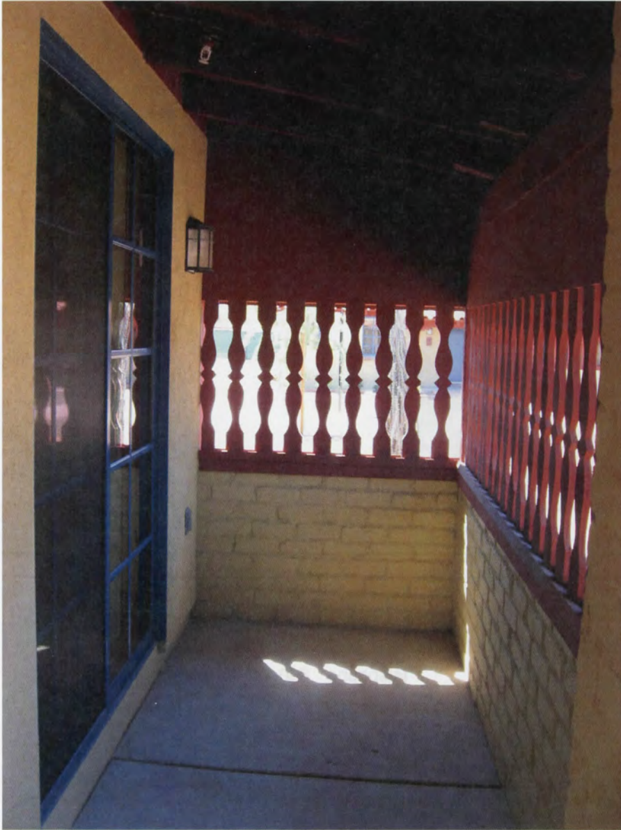
40. Original Building Group Recessed placement of the bedroom infill retains character of open carport in the form of a patio. (Photo by Don W. Ryden of Ryden Architects, Inc., 2010)
