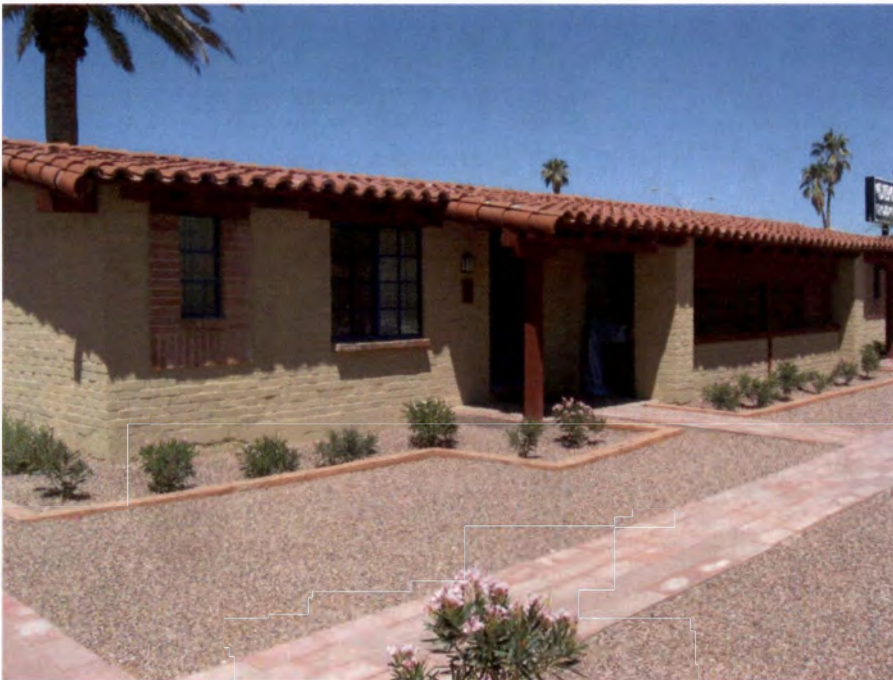
16. Original Building Group Joesler-designed Spanish Colonial Revival casita (Building E) with private porch and carport. View to northwest. (Photo by Paul C. Sikorski of Ryden Architects, Inc., 2010)
