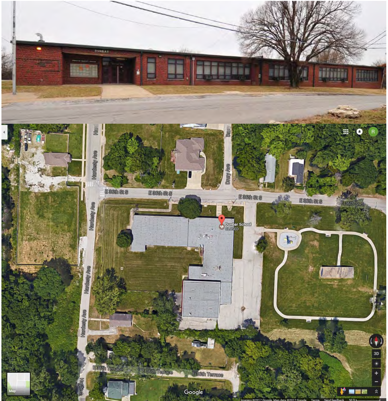
Figure 23. Dunbar School (5419 E. 36 th Street, 1956), Kansas City Public Schools, Photo and Plan. Source: Brad Finch, 2011; Google Maps, 2017.
