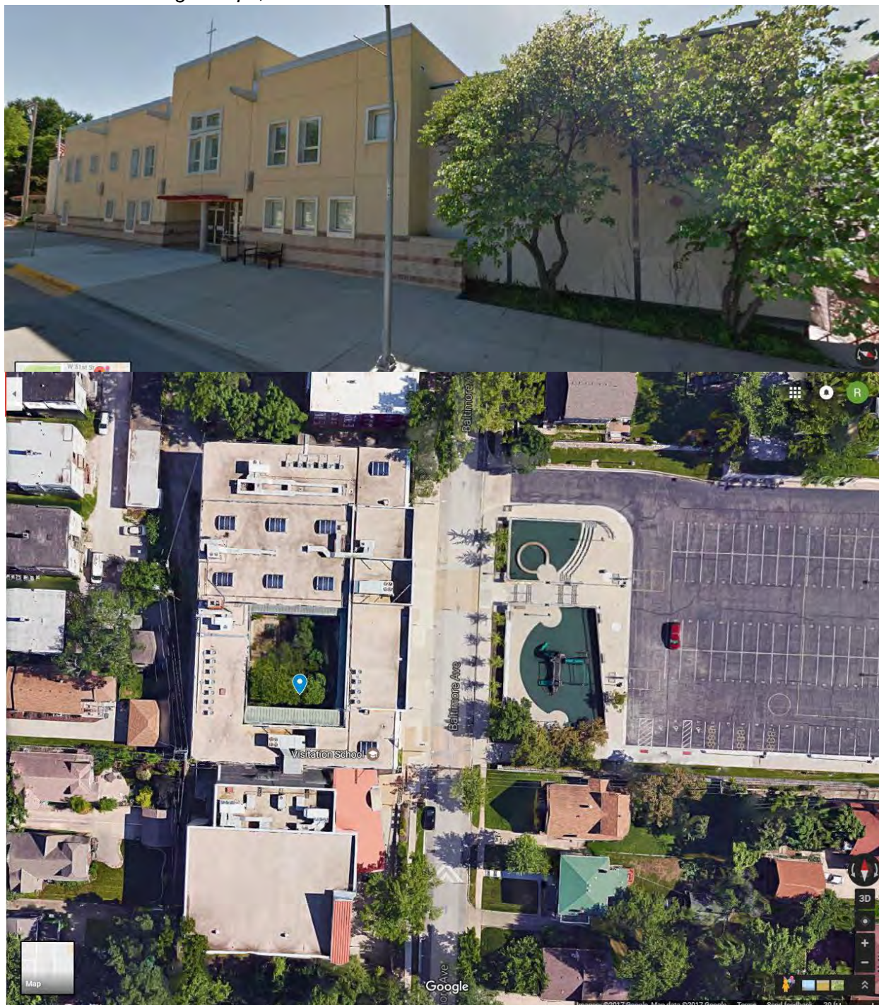
Figure 42. Visitation Parish School (5134 Baltimore Ave., 1960), Catholic School, Photo and Plan. Source: Google Maps, 2017.
