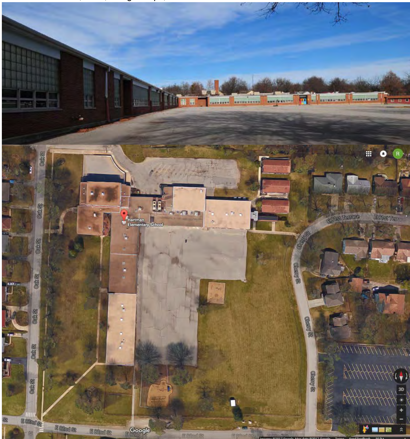
Figure 19. Hartman School (8111 Oak St., 1953), Kansas City Public Schools, Photo and Plan. Source: Brad Finch, 2011; Google Maps, 2017.
