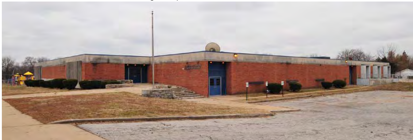
Figure 29. Franklin School (3400 Highland Ave., 1968), Kansas City Public Schools, Photo and Plan. Source: Brad Finch, 2011; Google Maps, 2017.
