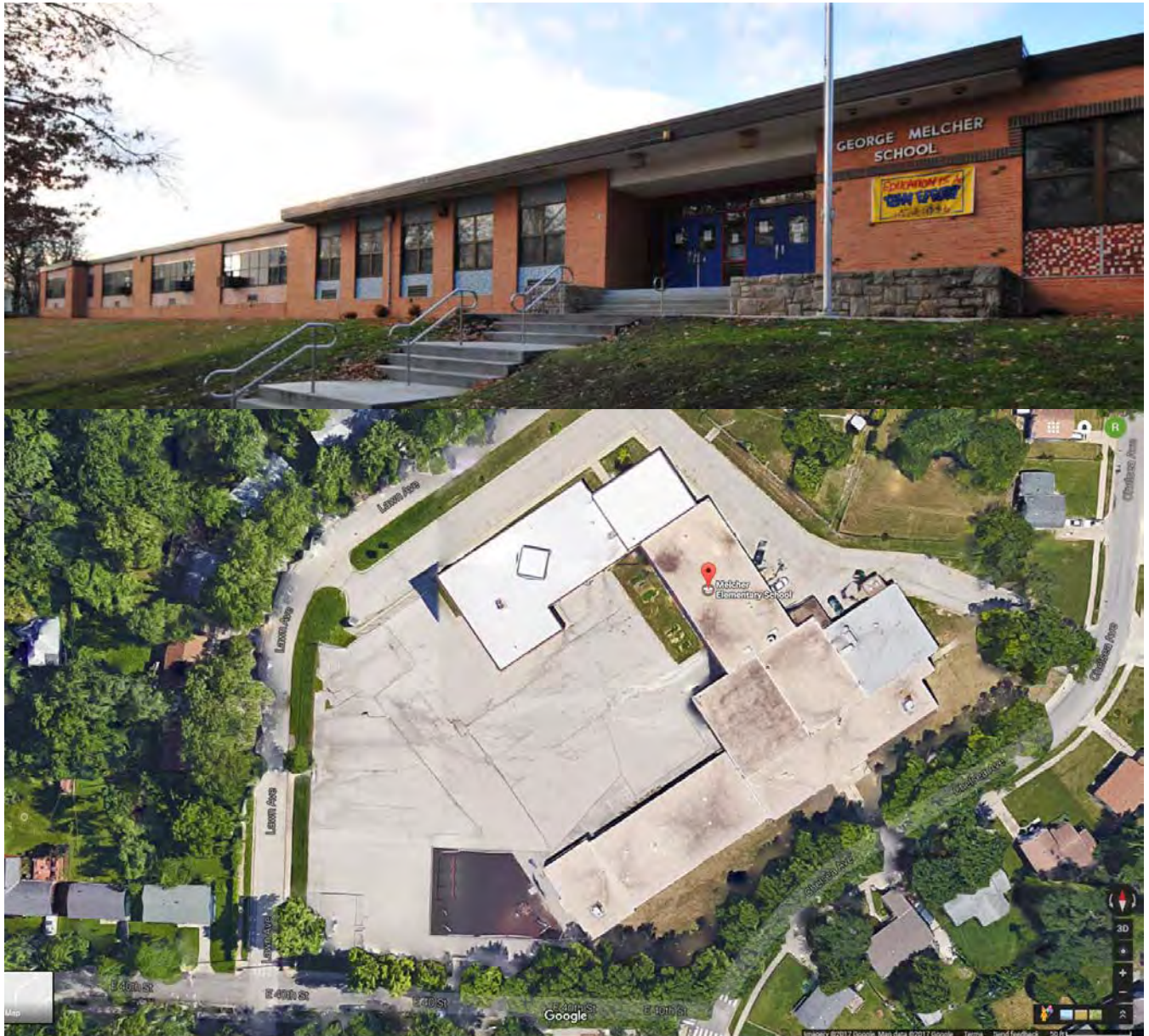
Figure 25. Melcher School (3958 Chelsea Ave., 1959), Kansas City Public Schools, Photo and Plan. Source: Brad Finch, 2011; Google Maps, 2017.
