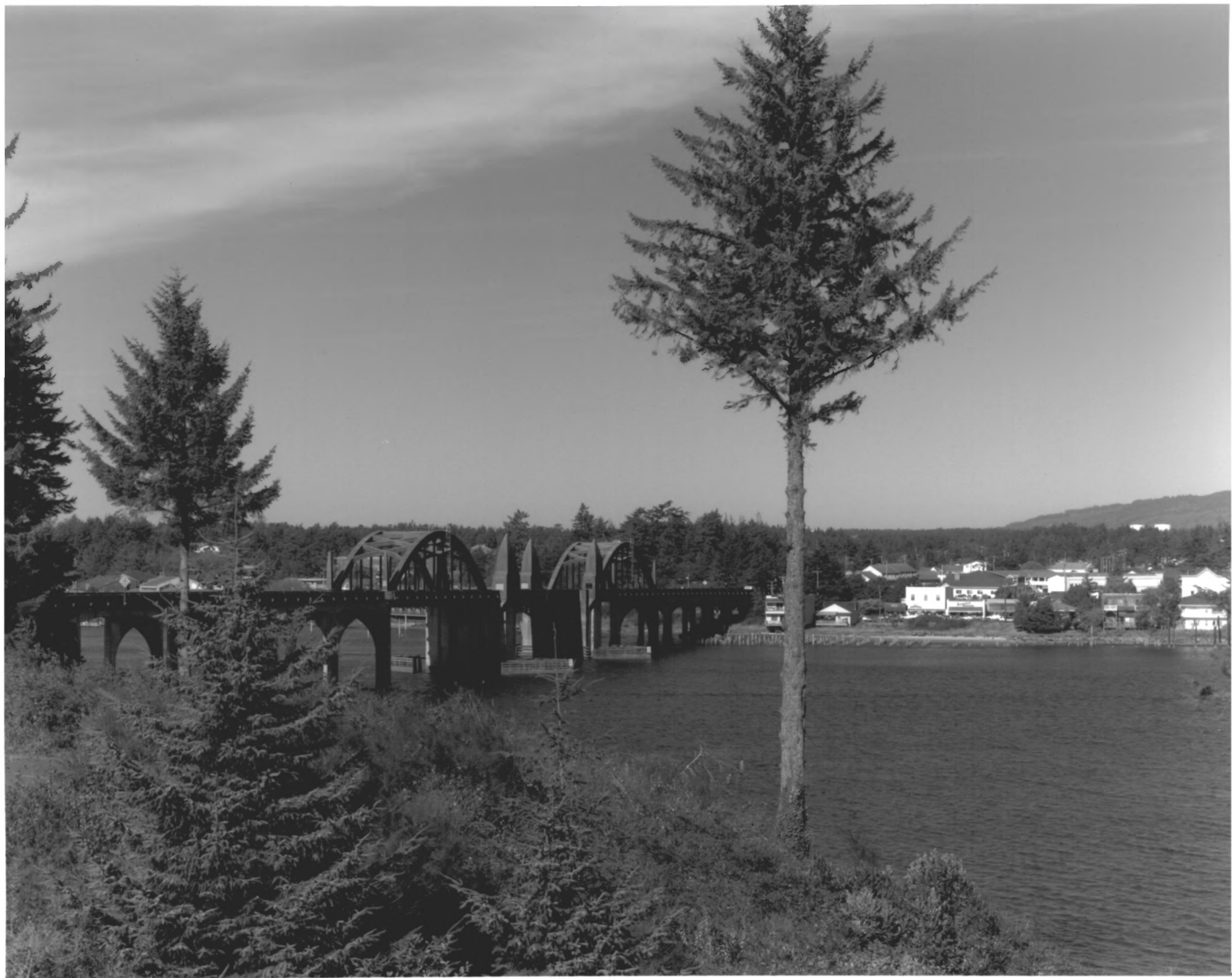
SIOUSLAW RIVER BRIDGE, FLORENCE, OREGON
