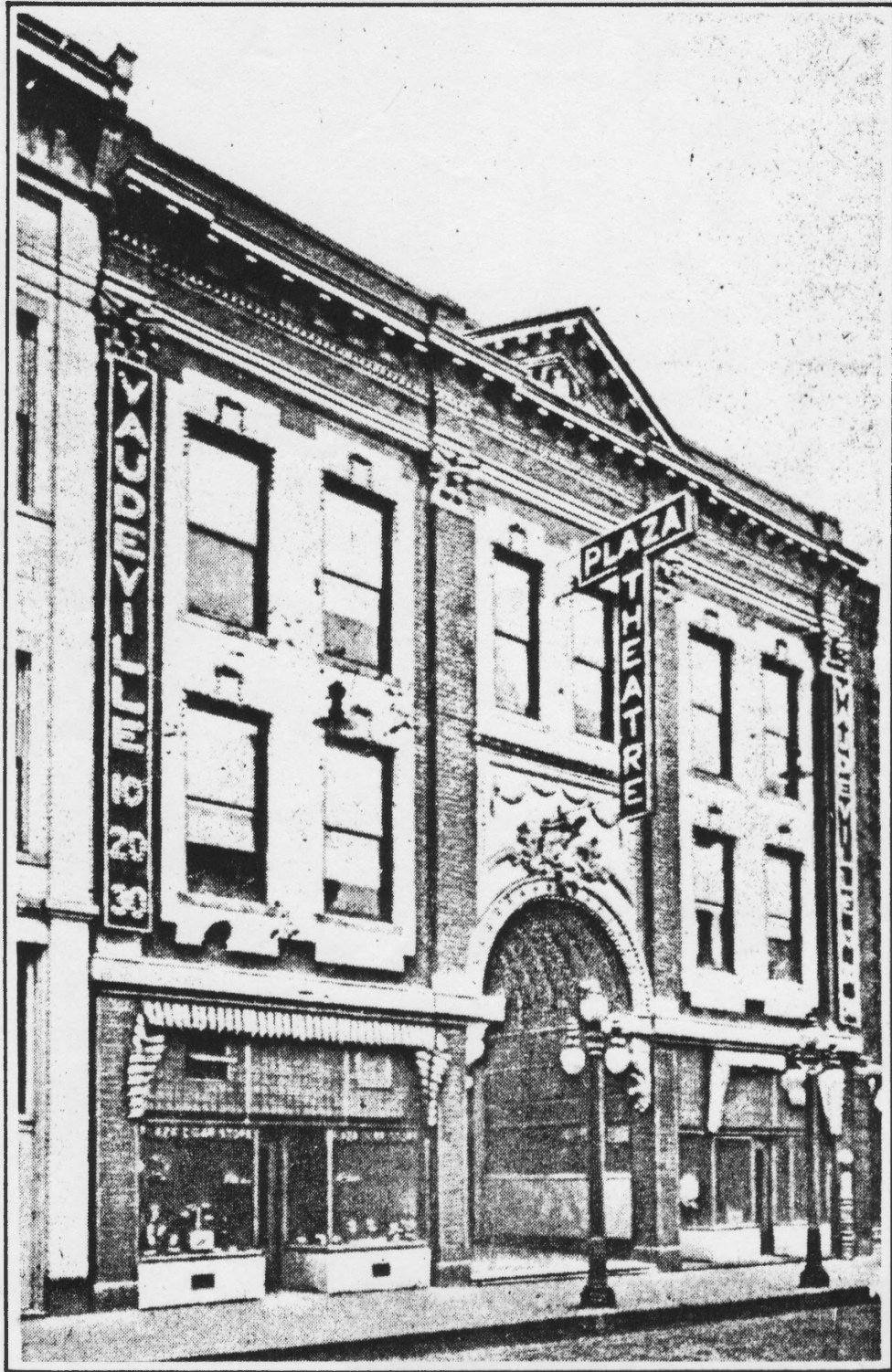
Photograph of the Plaza Theatre in its original architectural appearance as described in the Consolidated Amusement Co. lease. Photo courtesy of Charleston Newspapers.
