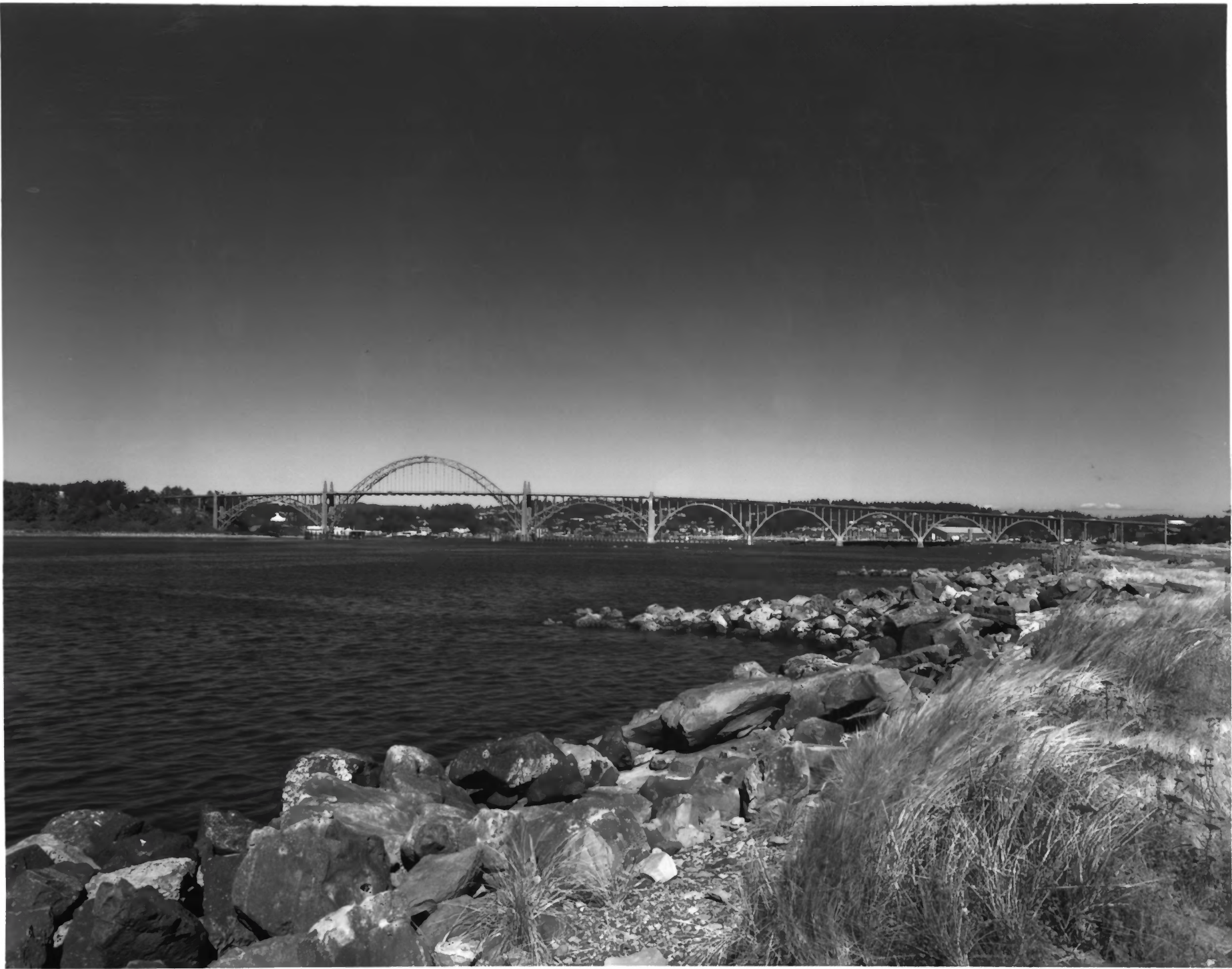
YARQUINA BAY BRIDGE, NEWPORT, OREGON
