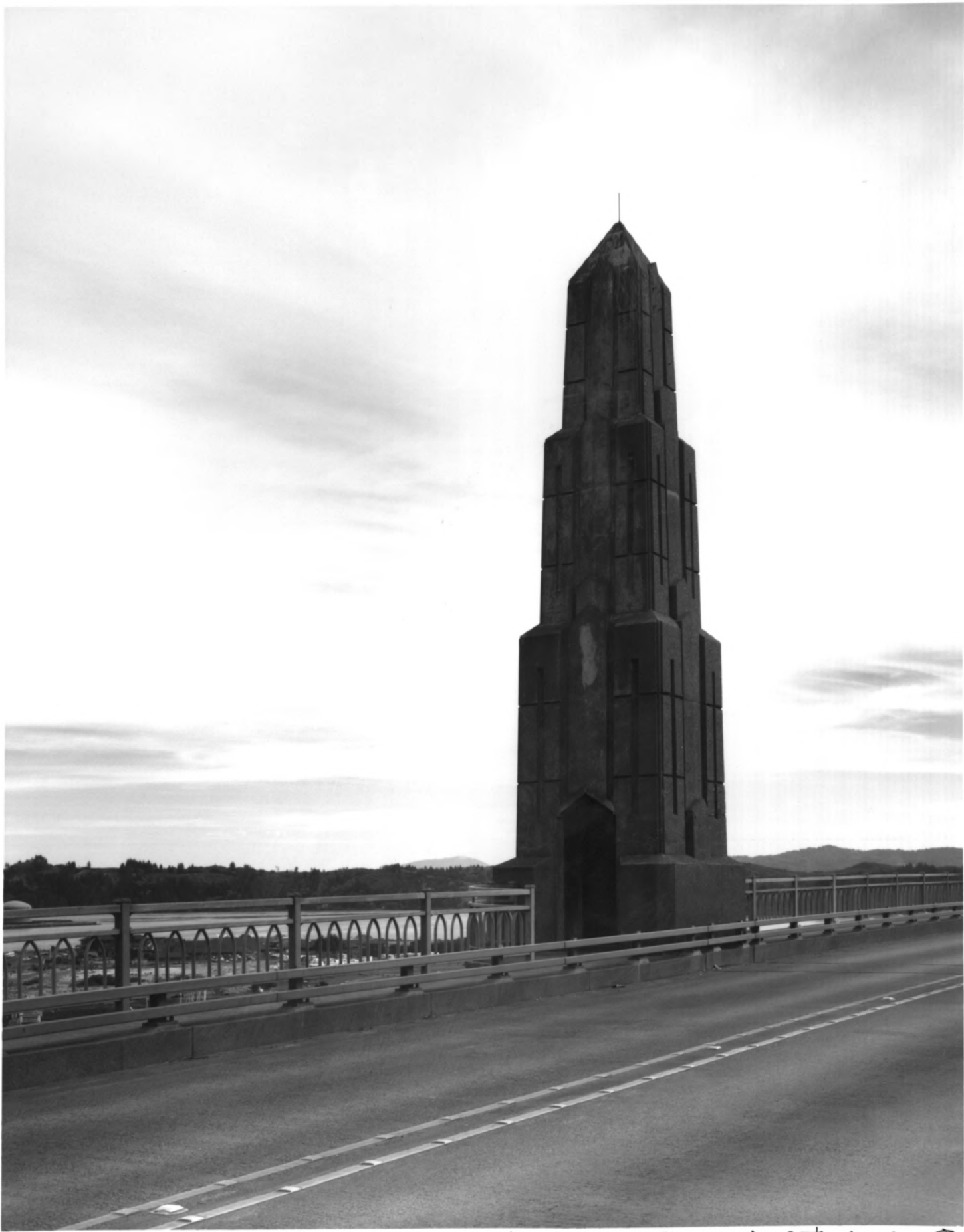
YAVINA BAY BRIDGE, NEWPORT, OREGON # 11
