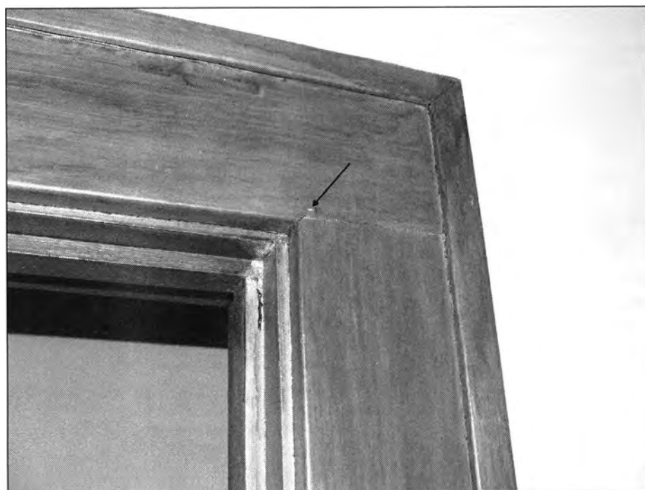
Figure 4: Door frame detail, arrow denotes mortised joint and 45-degree angle that is in line with the door jamb, etc.
