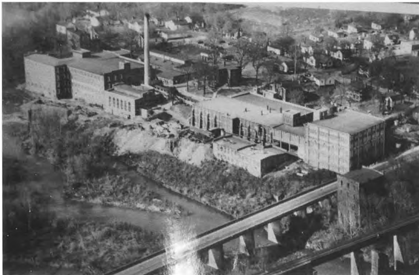
Figure 3. Granite Finishing Works, 1951 Photograph from the Haw River Historical Association Museum's collection
