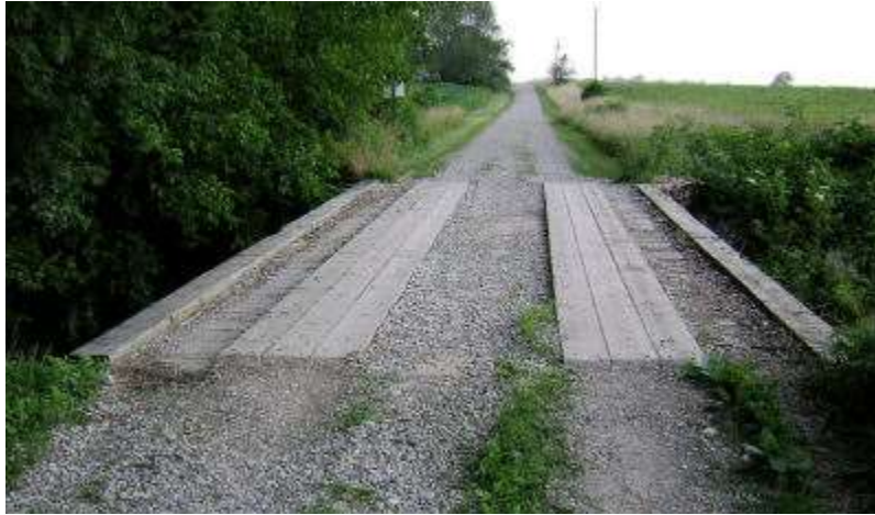
Figure 10: Typical bridge (50 years or older) classified as steel beam with wood decking by IDOT (Amity Bridge, Richland County, Wooden deck bridge over Paul Creek on TR 266. Bridgehunters.com)
