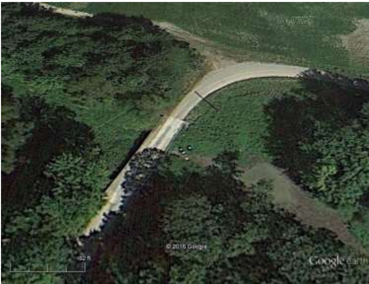
Figure 13: Chauncey vicinity, Bridge over the Slough from Google Earth
