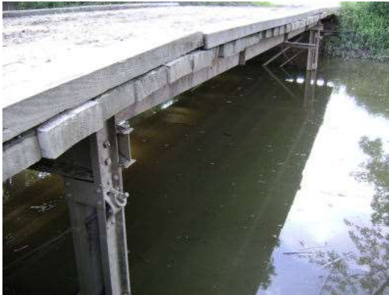
Figure 11: Richland County, Illinois Calfkiller Creek Bridge (Richland County, Illinois) Wooden deck steel beam bridge over Calfkiller Creek on TR 236
