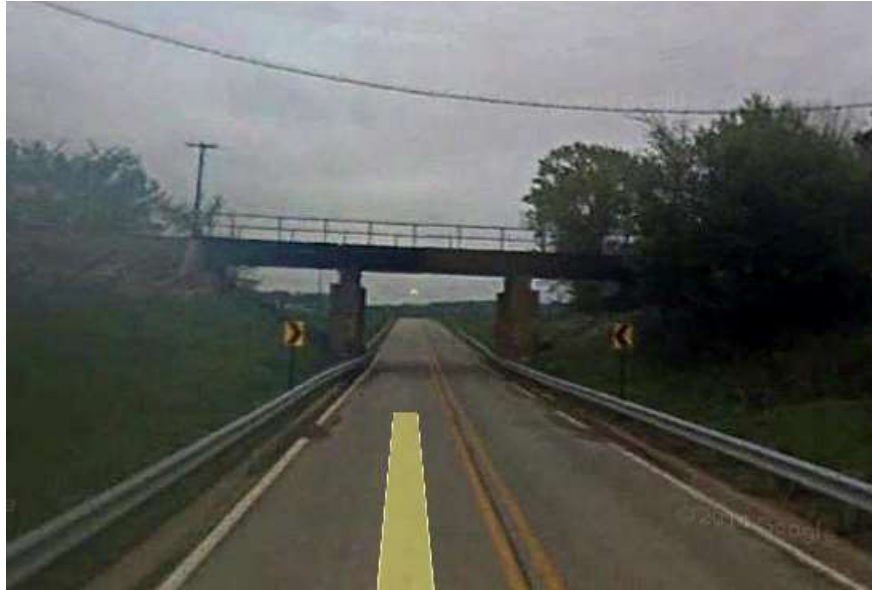
Figure 14: Vincennes vicinity, Bridge over ILL-33, from Google Earth
