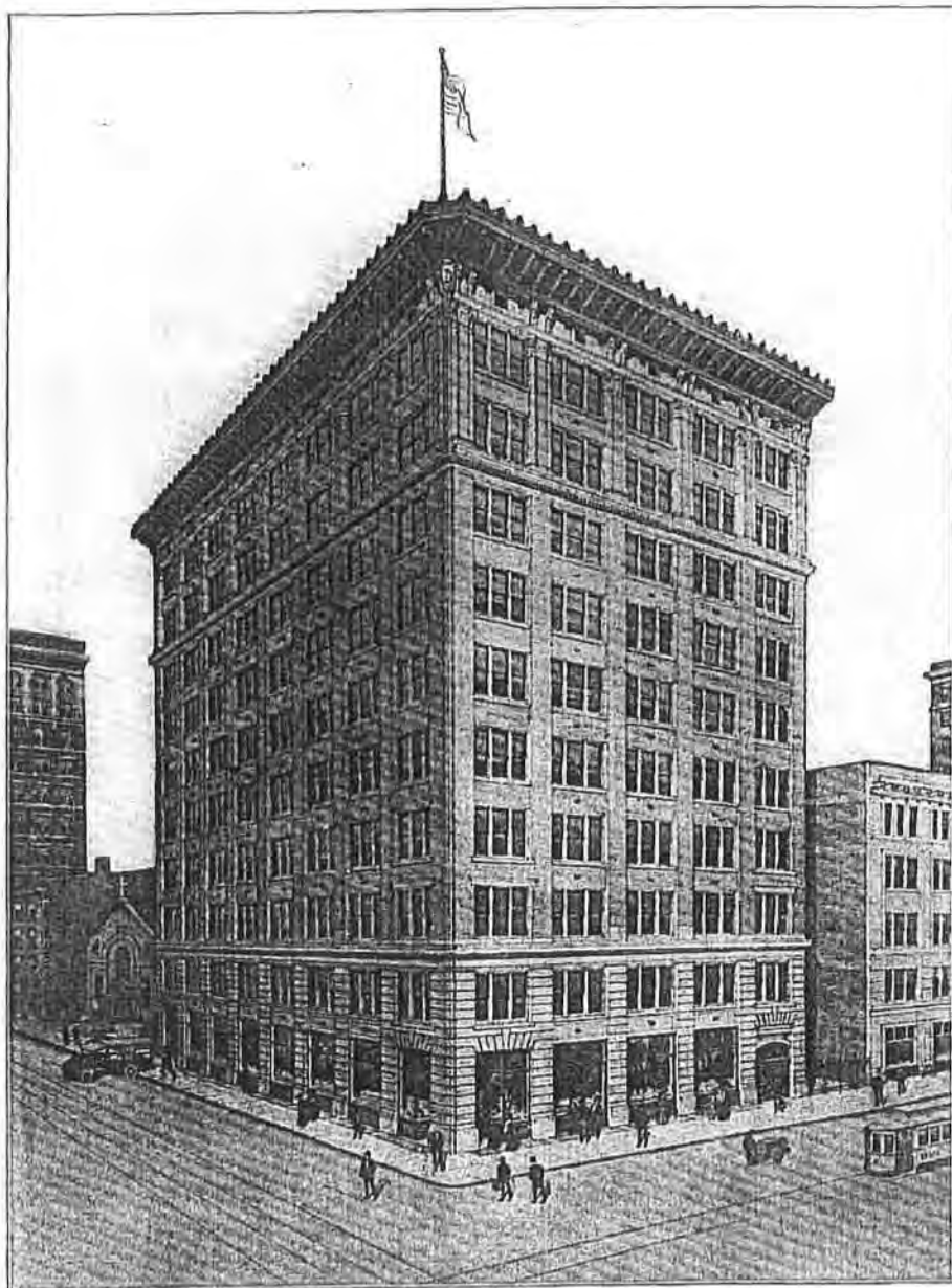
DUTTENHOFER BUILDING S. W. COR. SIXTH & SYCAMORE STREETS Ready For Occupancy December 1st, 1915 VAL DUTTENHOFER, Jr., Owner
