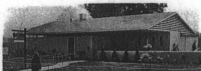
Riverside, California. Builder Gordon Fields followed specifications closely in building this house. Visitors numbered in the thousands
