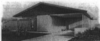
Fort Worth, Texas. Approximately 2,500 people visited this house the first day it was opened for inspection. Built by Frank S. Retzlaff
