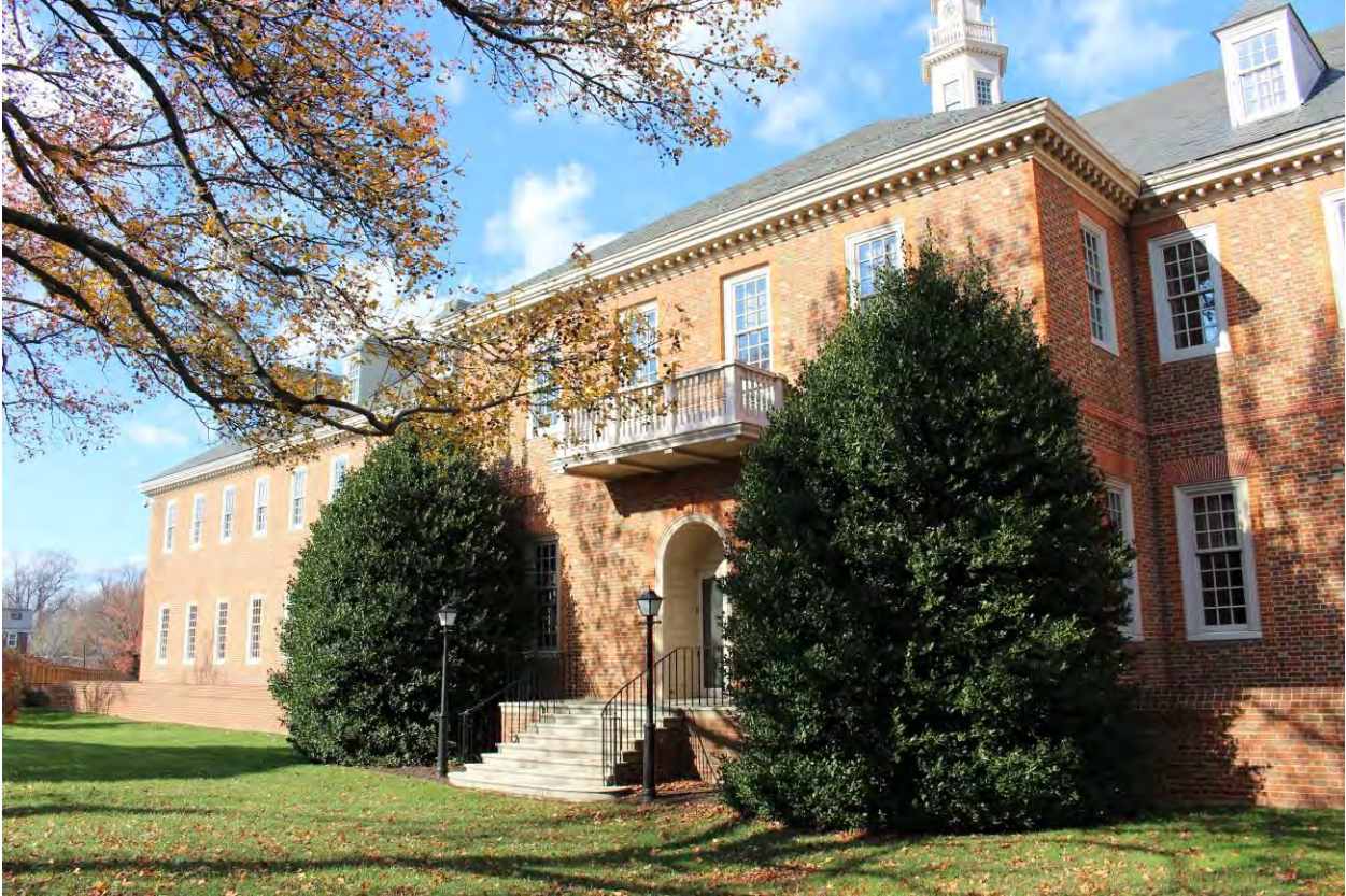
Photograph 6 of 26: South elevation of south wing, facing northwest.
