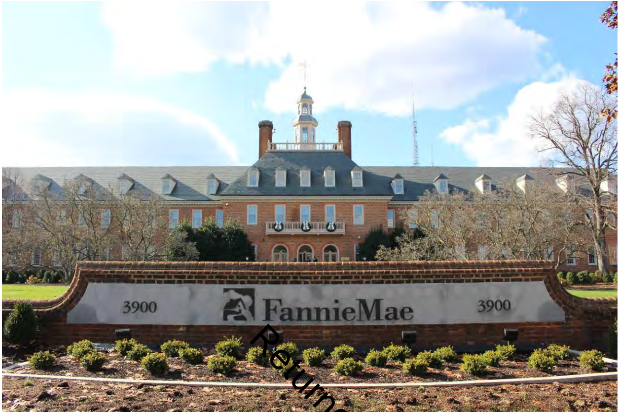
Photograph 1 of 22: Front (east) elevation facing southwest.
