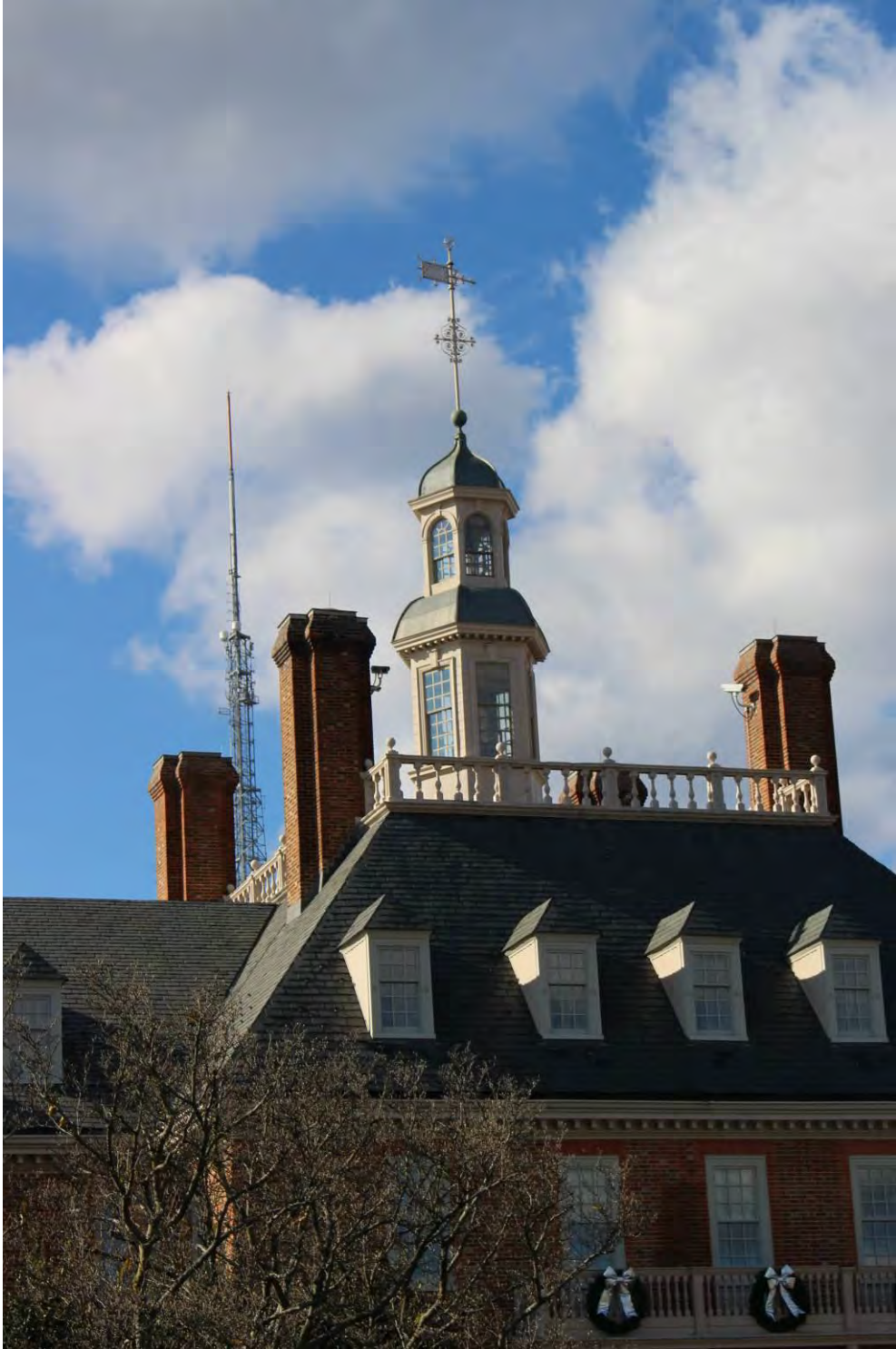
Photograph 3 of 26: Center hall roof with cupola and chimneys, facing west.
