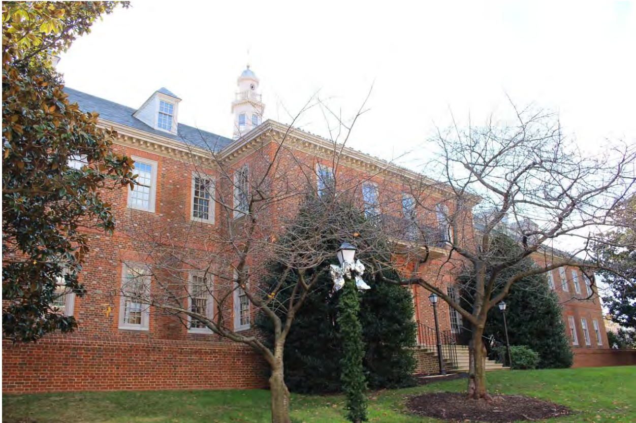
Photograph 12 of 26: North elevation of north wing, facing southwest.
