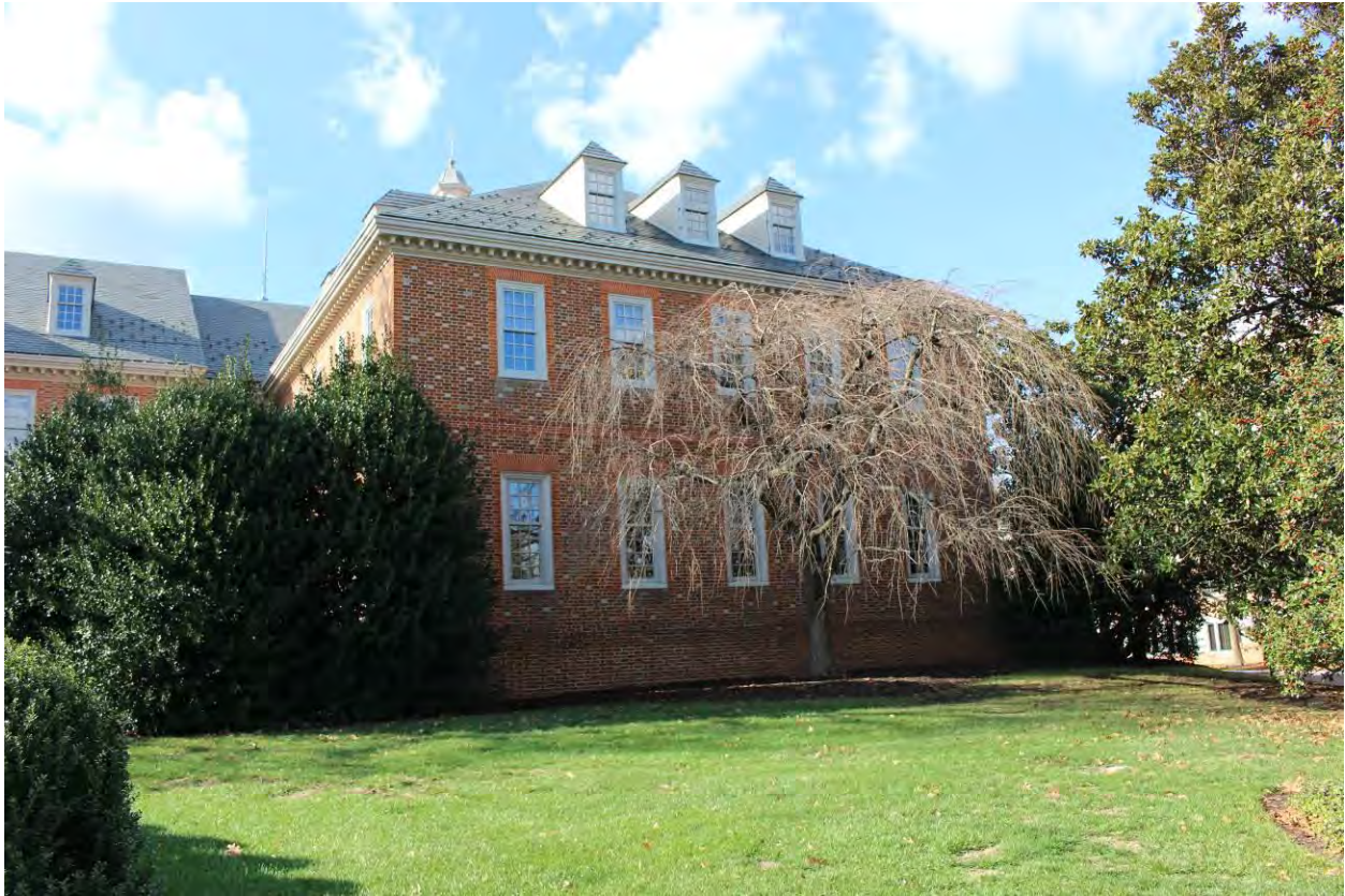
Photograph 11 of 26: East elevation of north wing, facing west.
