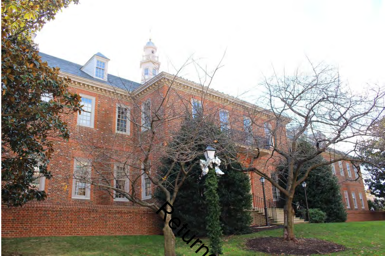
Photograph 12 of 22: North elevation of north wing, facing southwest.
