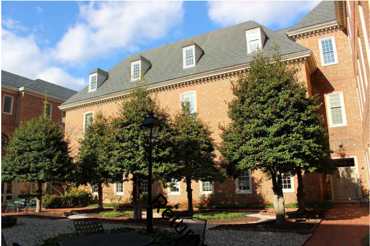
Photograph 17 of 22: View from south courtyard showing south elevation of 1950s section, facing northwest.
