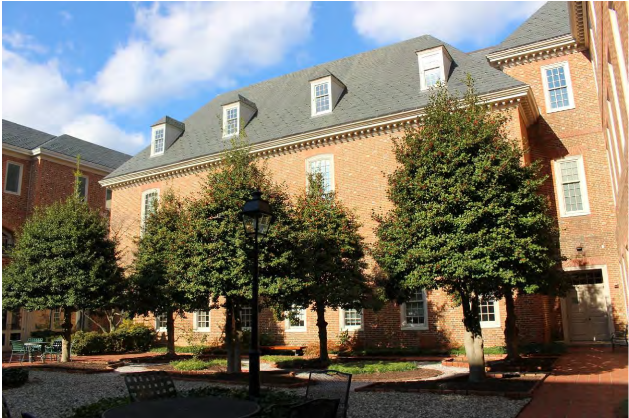
Photograph 17 of 26: View from south courtyard showing south elevation of 1950s section, facing northwest.
