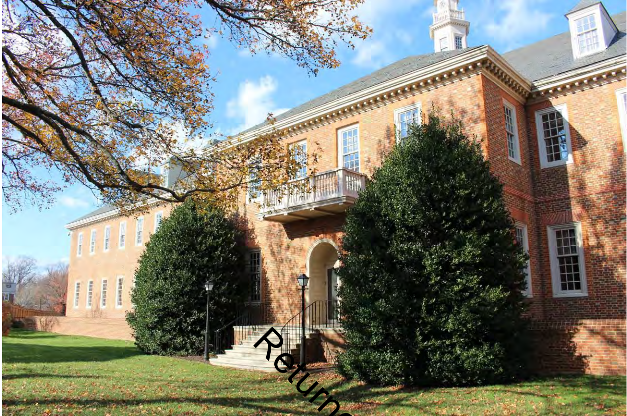
Photograph 6 of 22: South elevation of south wing, facing northwest.
