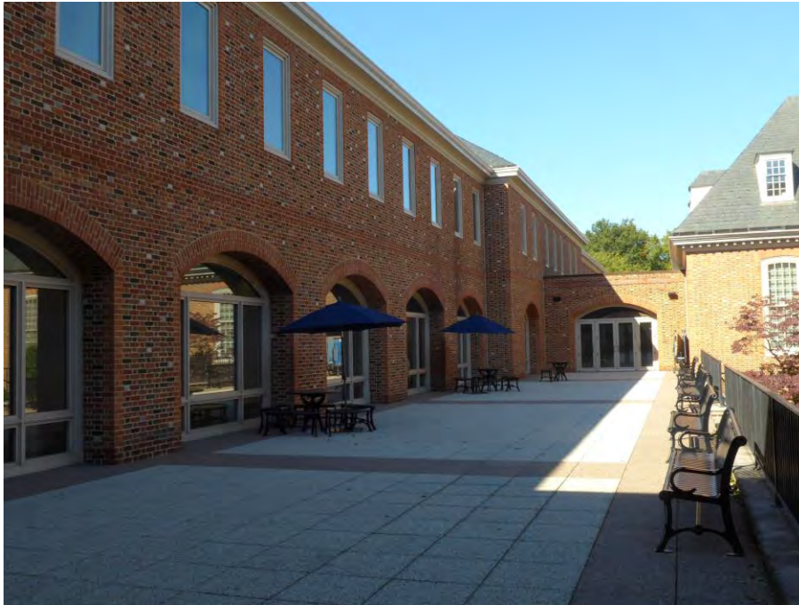
2018 view of the east elevation of the 1978 addition looking north. The brick hyphen (background) connected the addition to the original building's central pavilion
