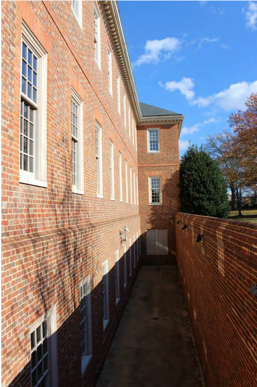
Photograph 8 of 26: South elevation of south wing, including basement level, facing east.
