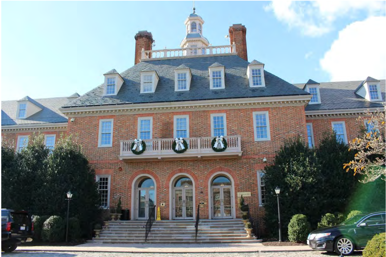
Photograph 2 of 26: Front entrance and center hall front elevation, facing southwest.
