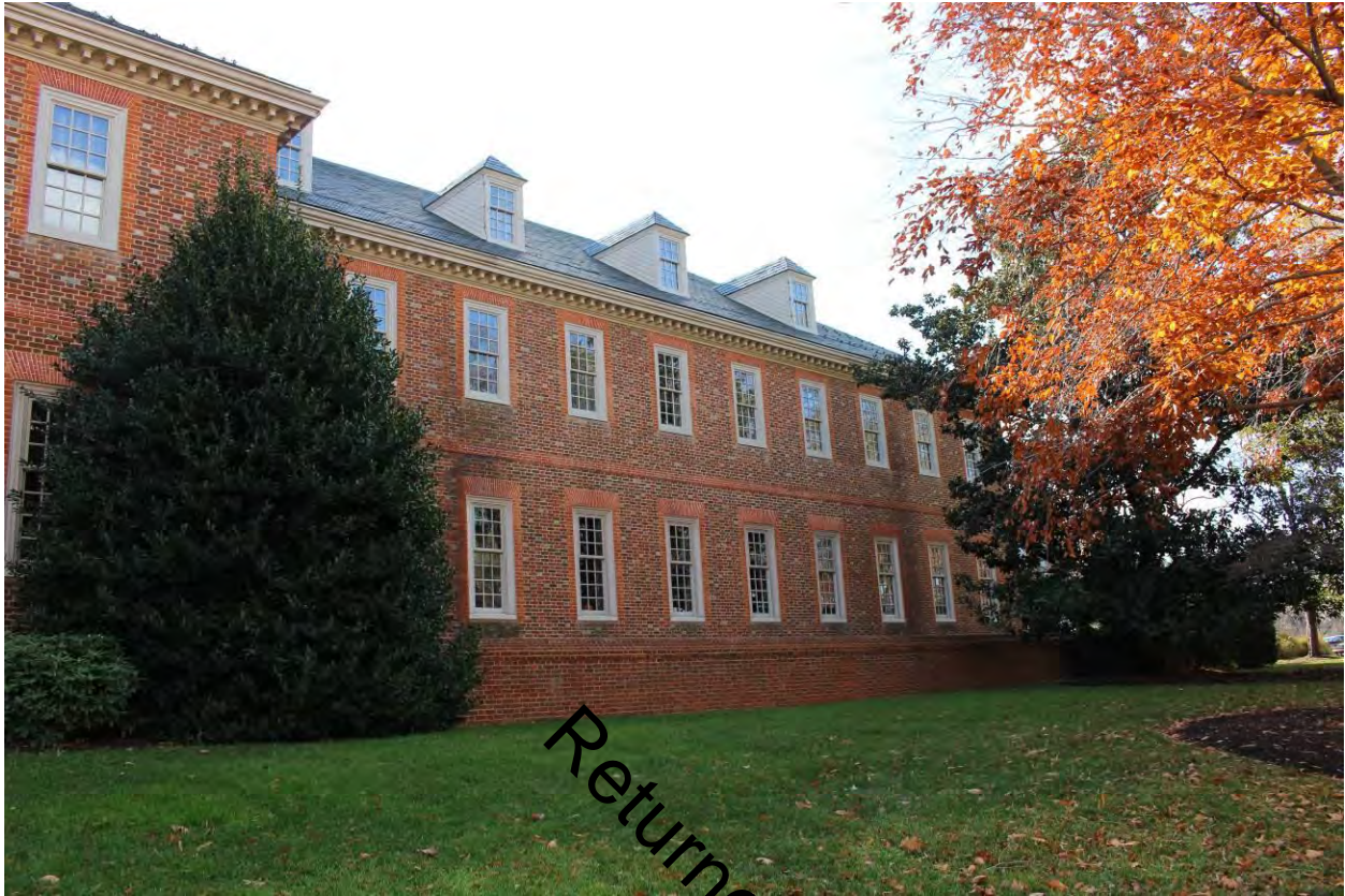
Photograph 14 of 22: North elevation of north wing, facing southwest.
