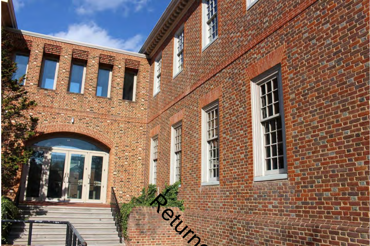
Photograph 9 of 22: West elevation of south wing and connection to 1978 addition, facing northeast.
