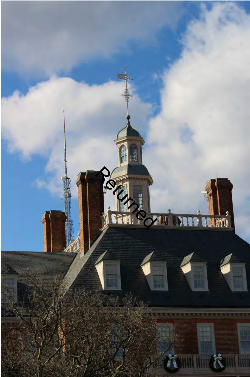
Photograph 3 of 22: Center hall roof with cupola and chimneys, facing west.
