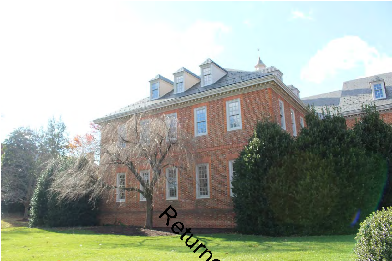
Photograph 5 of 22: East elevation of South wing, facing southwest.
