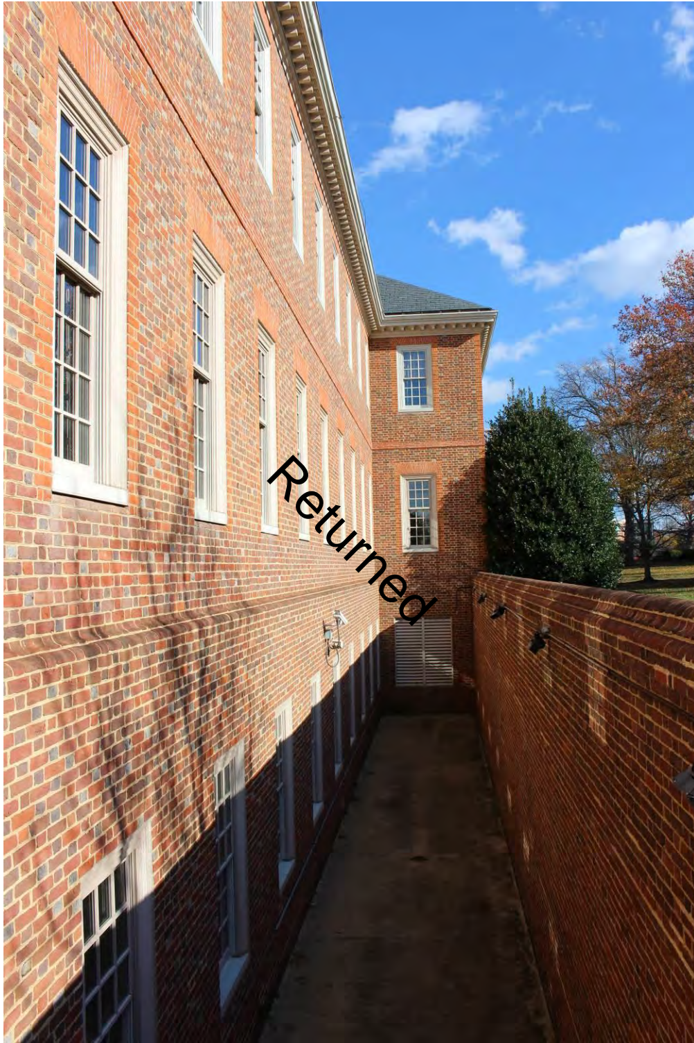
Photograph 8: South elevation of south wing, including basement level, facing east.
