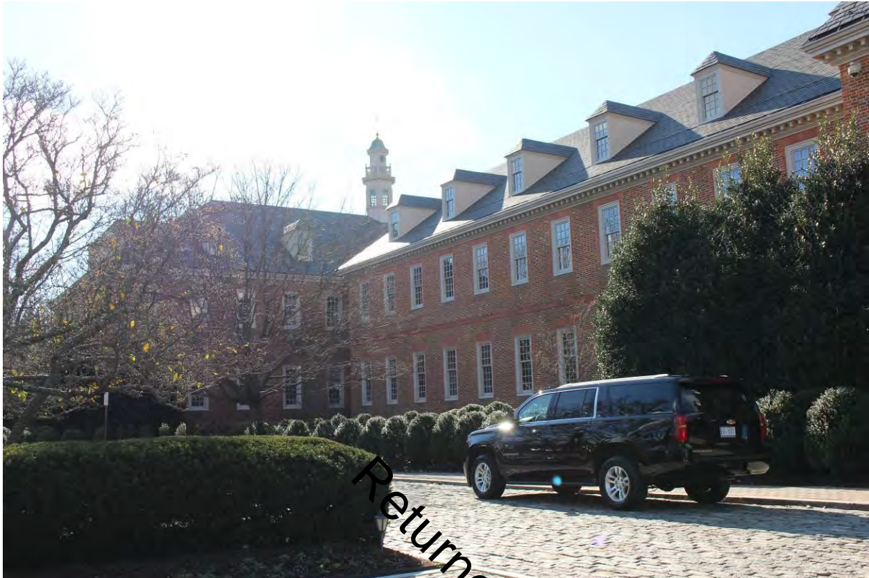
Photograph 4 of 22: Front (east) elevation of south connector and north elevation of south wing, facing southwest.
