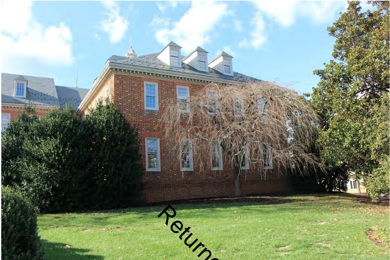
Photograph 11 of 22: East elevation of north wing, facing west.
