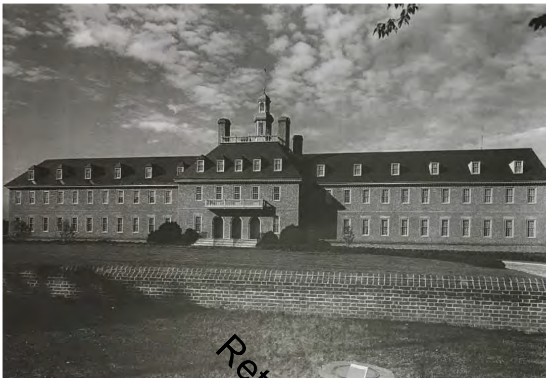
Equitable Life Headquarters before construction of the side wings, c.1958-1962 (Courtesy of Leon Chatelain III)
