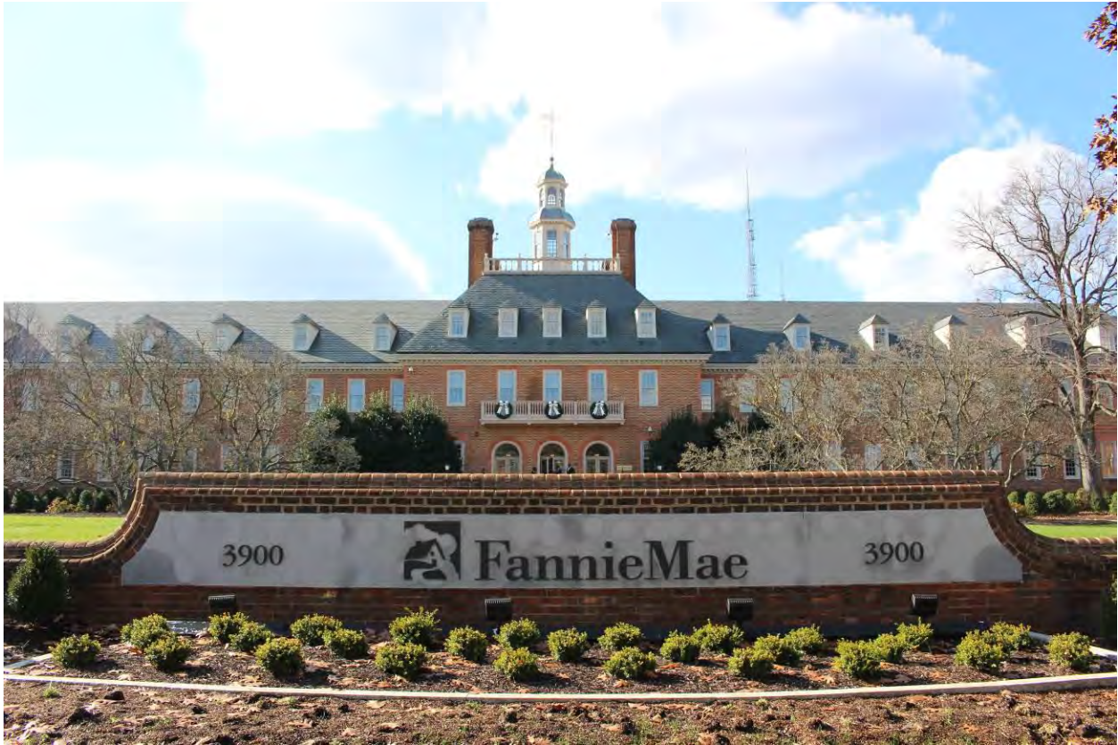
Photograph 1 of 26: Front (east) elevation facing southwest.
