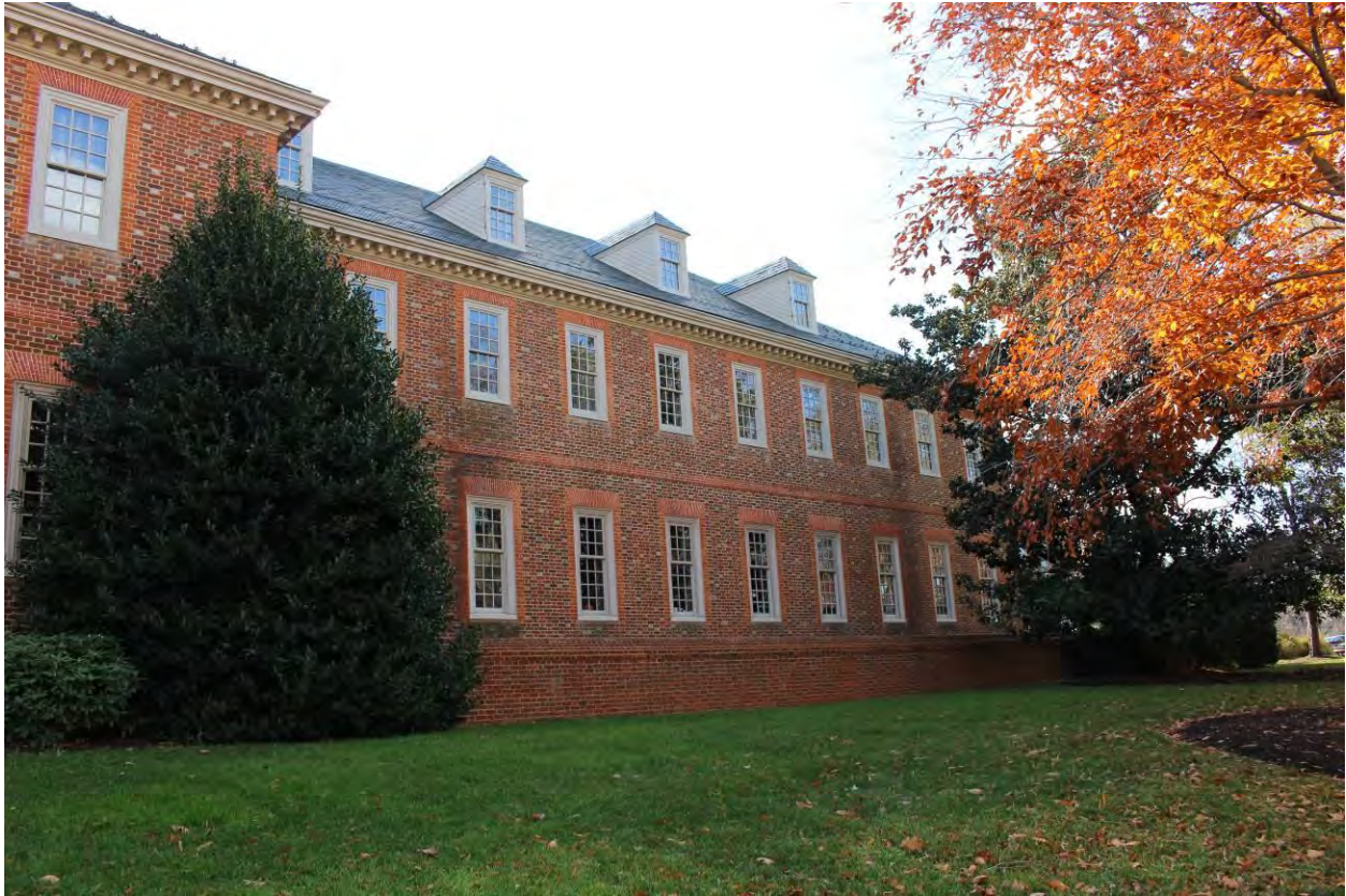
Photograph 14 of 26: North elevation of north wing, facing southwest.
