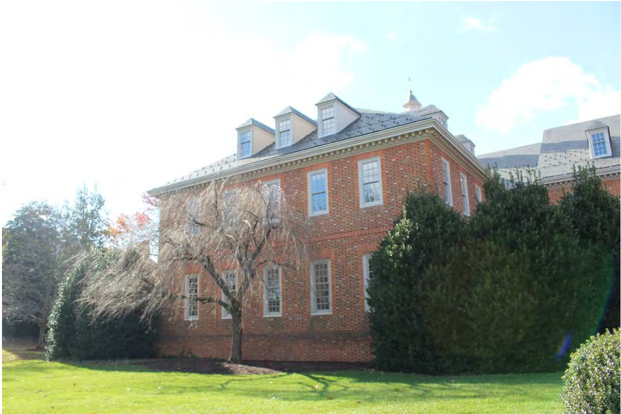
Photograph 5 of 26: East elevation of south wing, facing southwest.
