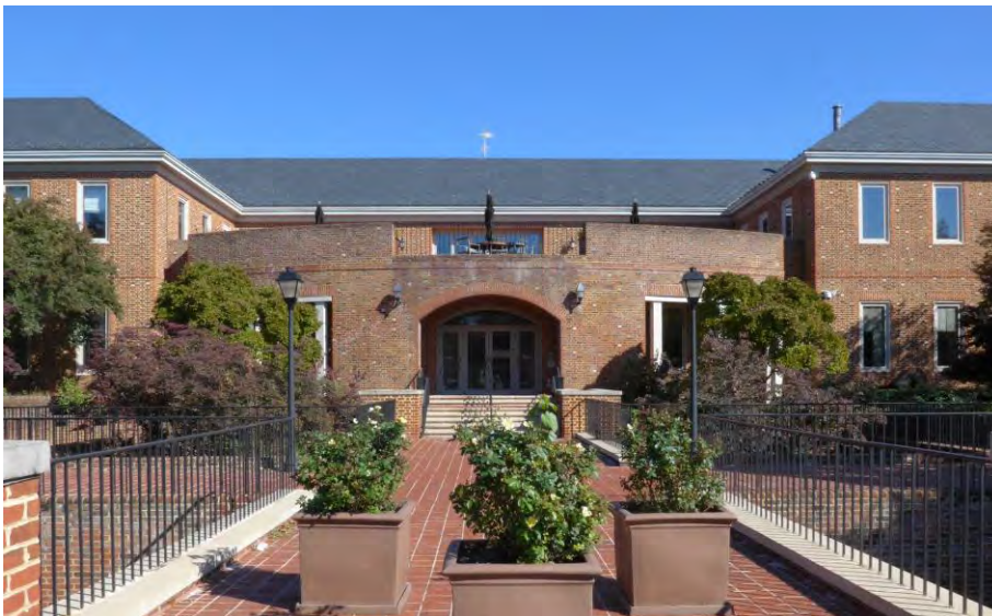
West elevation of center block of 1978 addition (2018)
