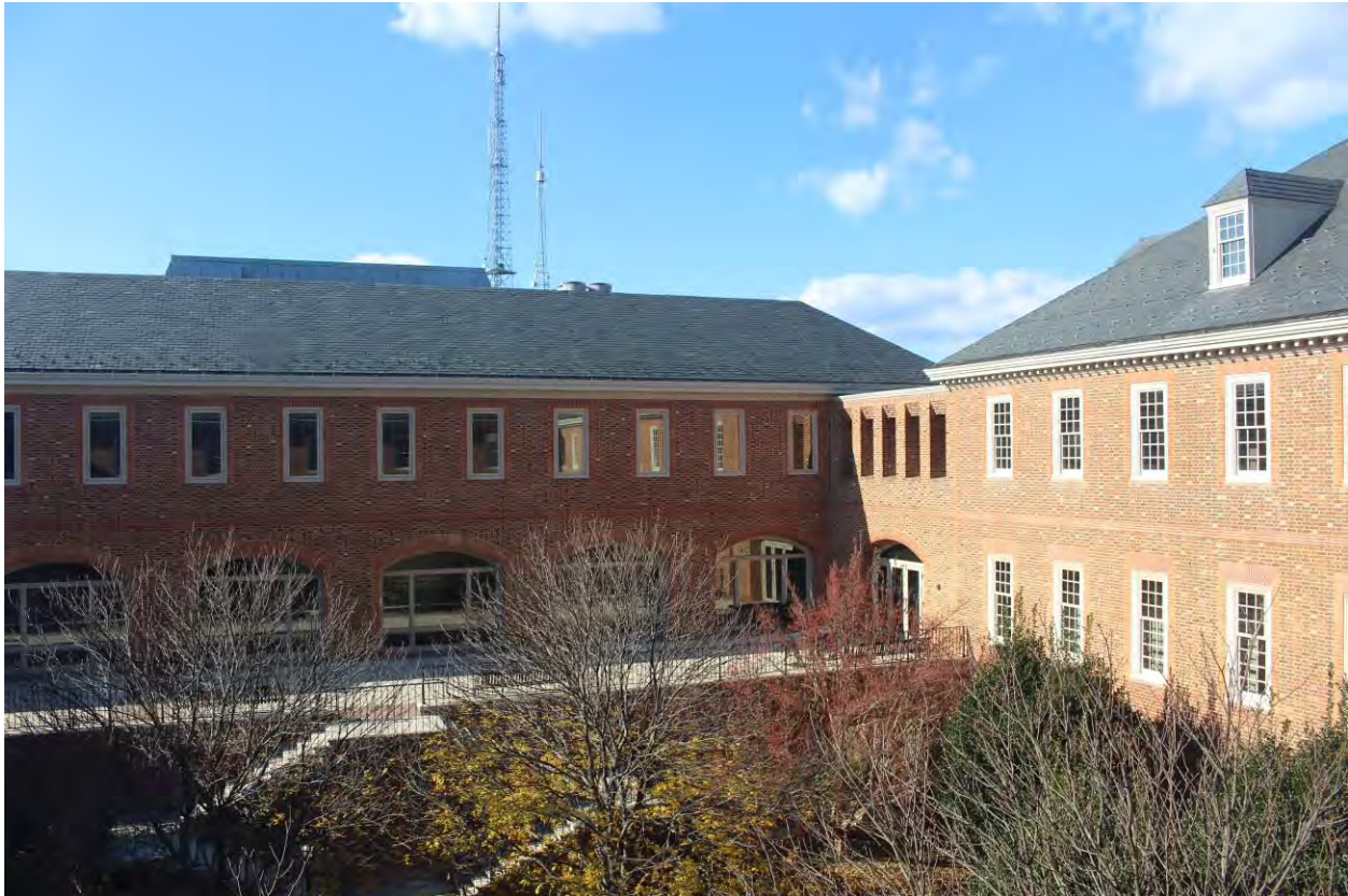
Photograph 15 of 26: View from second floor onto north courtyard showing connection between north wing and 1978 addition, facing west. The 1978 addition was demolished in 2019.
