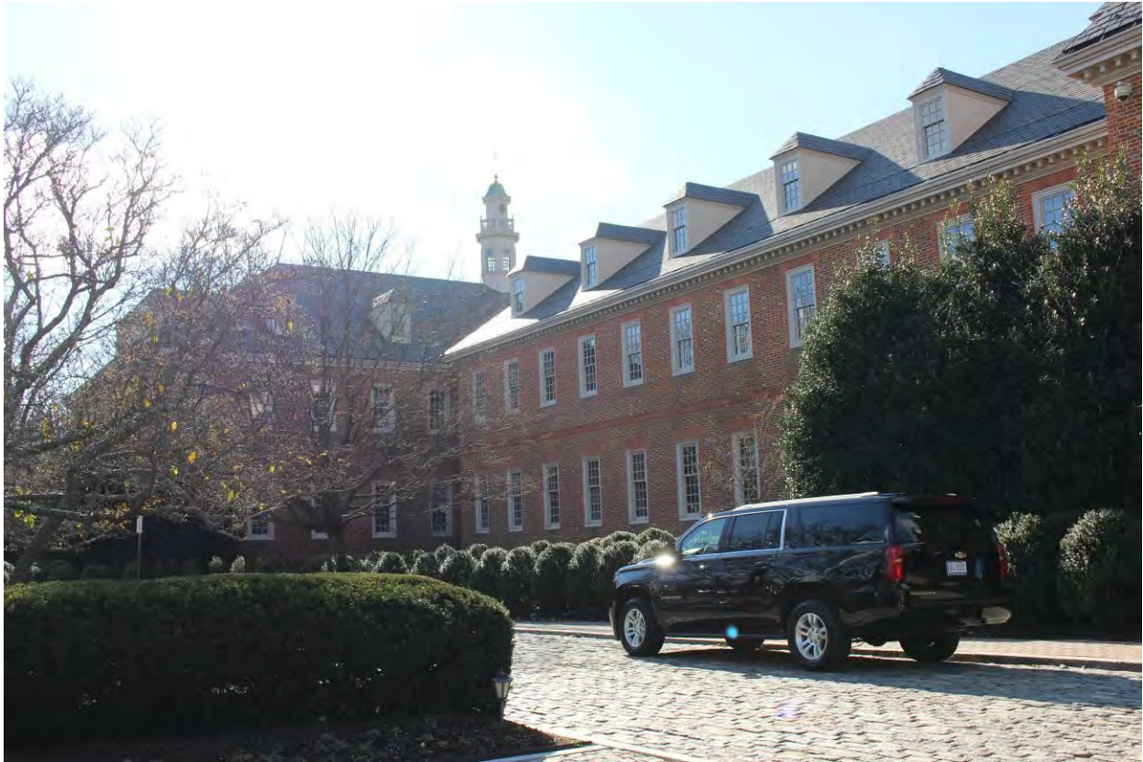
Photograph 4 of 26: Front (east) elevation of south connector and north elevation of south wing, facing southwest.
