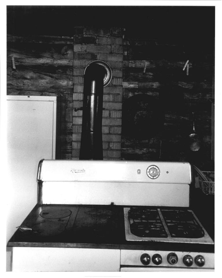
JACK CREEK GUARD STATION (48CR4074) Cabin interior detailing: split pole wedge chinking, brick chimmey, etc.
