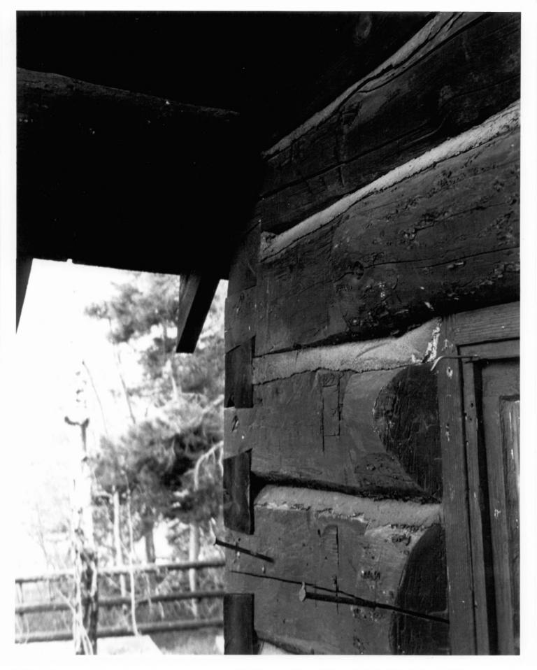
JACK CREEK GUARD STATION (48CR4074) Cabin construction detail: sawn log dovetail notching, hewn corners Photo taken facing southwest July 1985 Negative at Medicine Bow NF
