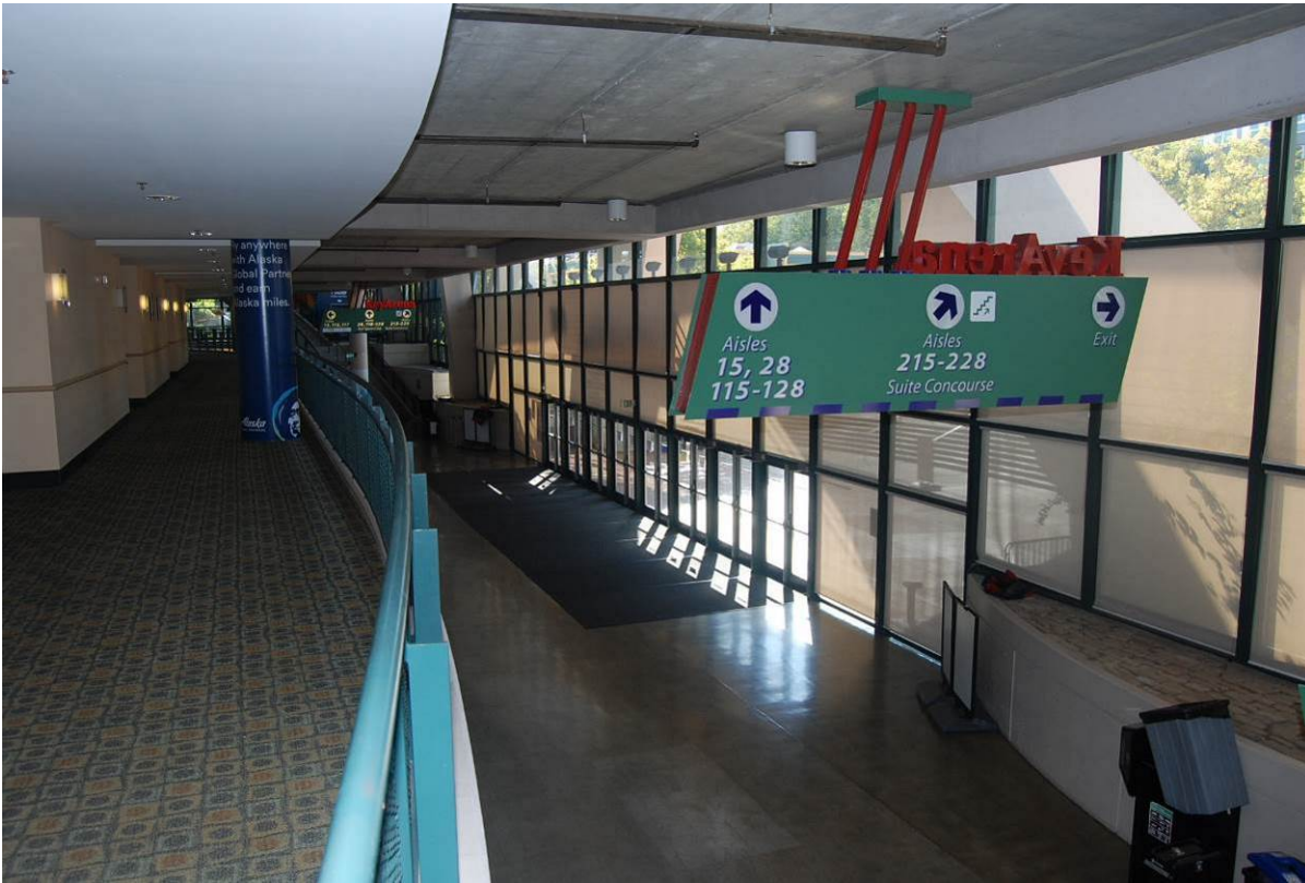
Photo 34 of 46 (WA_King County_Century 21 Coliseum_0034) – October 2017 View of the west side of the suite concourse level, facing southwest
