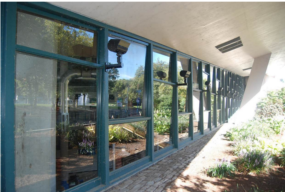
Photo 17 of 46 (WA_King County_Century 21 Coliseum_0017) – October 2017 Detail view of the east façade, facing northwest
