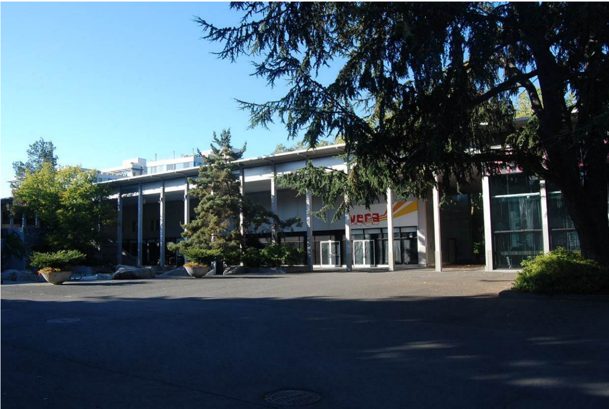
Photo 25 of 46 (WA_King County_Century 21 Coliseum_0025) – October 2017 Context view of adjacent International Plaza and International Commerce and Industry Buildings, facing northwest
