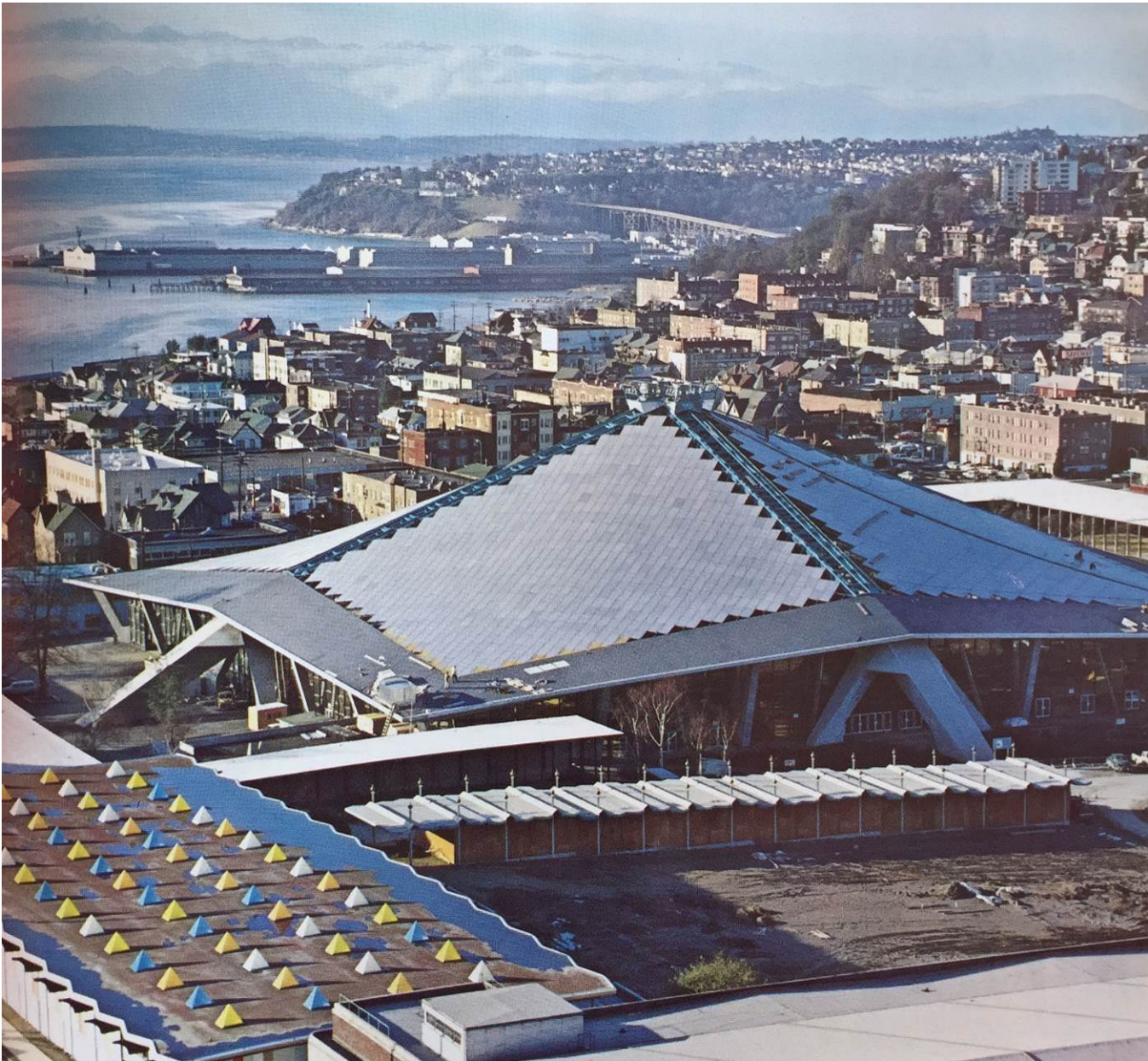
Century 21 Coliseum, 1961 - southeast corner, view towards the northwest. "Plaza of the States" in foreground under construction. Mayor Gordon S. Clinton, "Seattle's Permanent Civic Center." Unknown, 66-71. Seattle Municipal Archives
