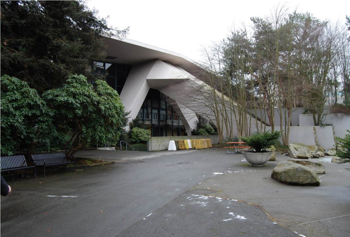
Photo 24 of 46 (WA_King County_Century 21 Coliseum_0024) – February 2017 Overall view of the north façade, facing southwest
