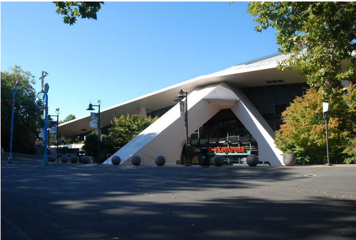
Photo 21 of 46 (WA_King County_Century 21 Coliseum_0021) – October 2017 Overall view of the east façade, facing southwest
