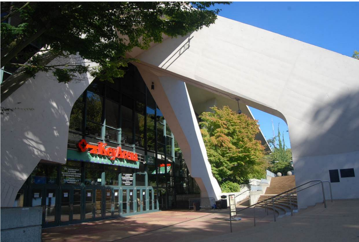
Photo 19 of 46 (WA_King County_Century 21 Coliseum_0019) – October 2017 Detail view of the entrance on the east façade and tripodal concrete buttress, facing northwest
