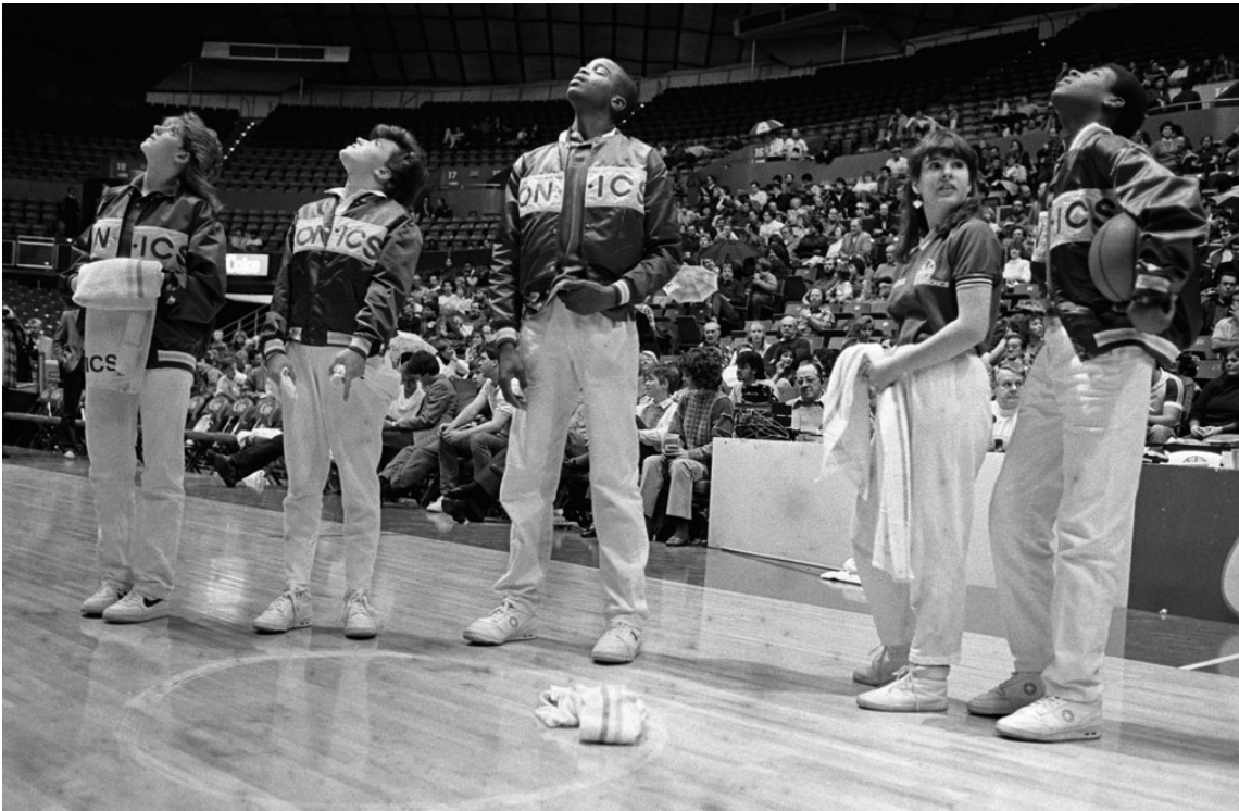
Members of the Sonics look up at the leaky roof of the Seattle Coliseum The Seattle Times – January 5, 1986
