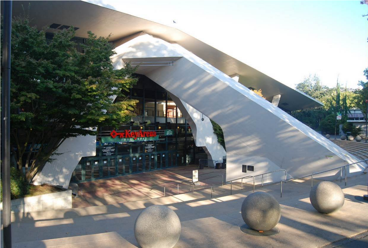
Photo 18 of 46 (WA_King County_Century 21 Coliseum_0018) – October 2017 Overall view of the east façade, facing northwest
