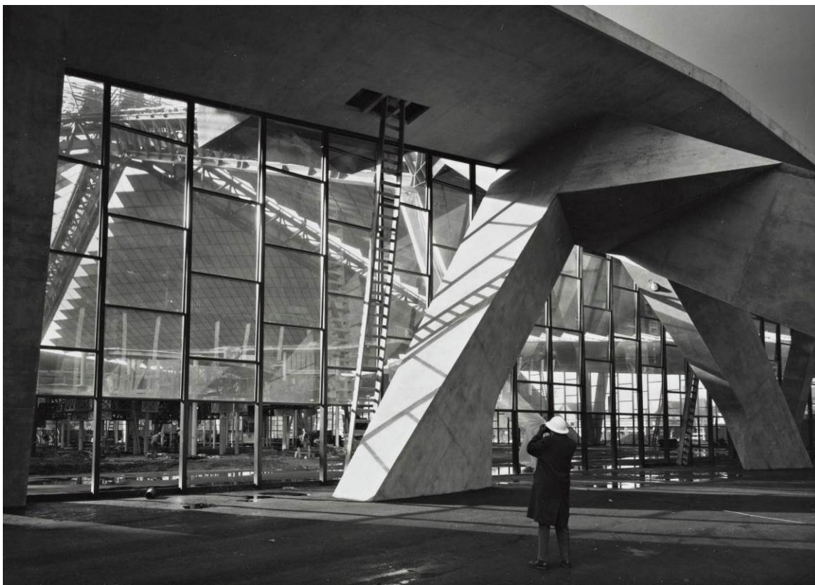
Century 21 Coliseum under construction, 1961 Department of Archaeology & Historic Preservation
