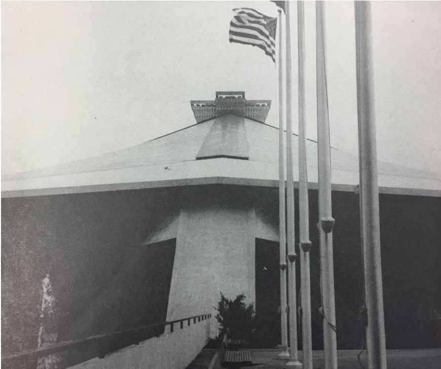
Century 21 Coliseum just after roof completed, 1962 Architectural Record – June 1962
