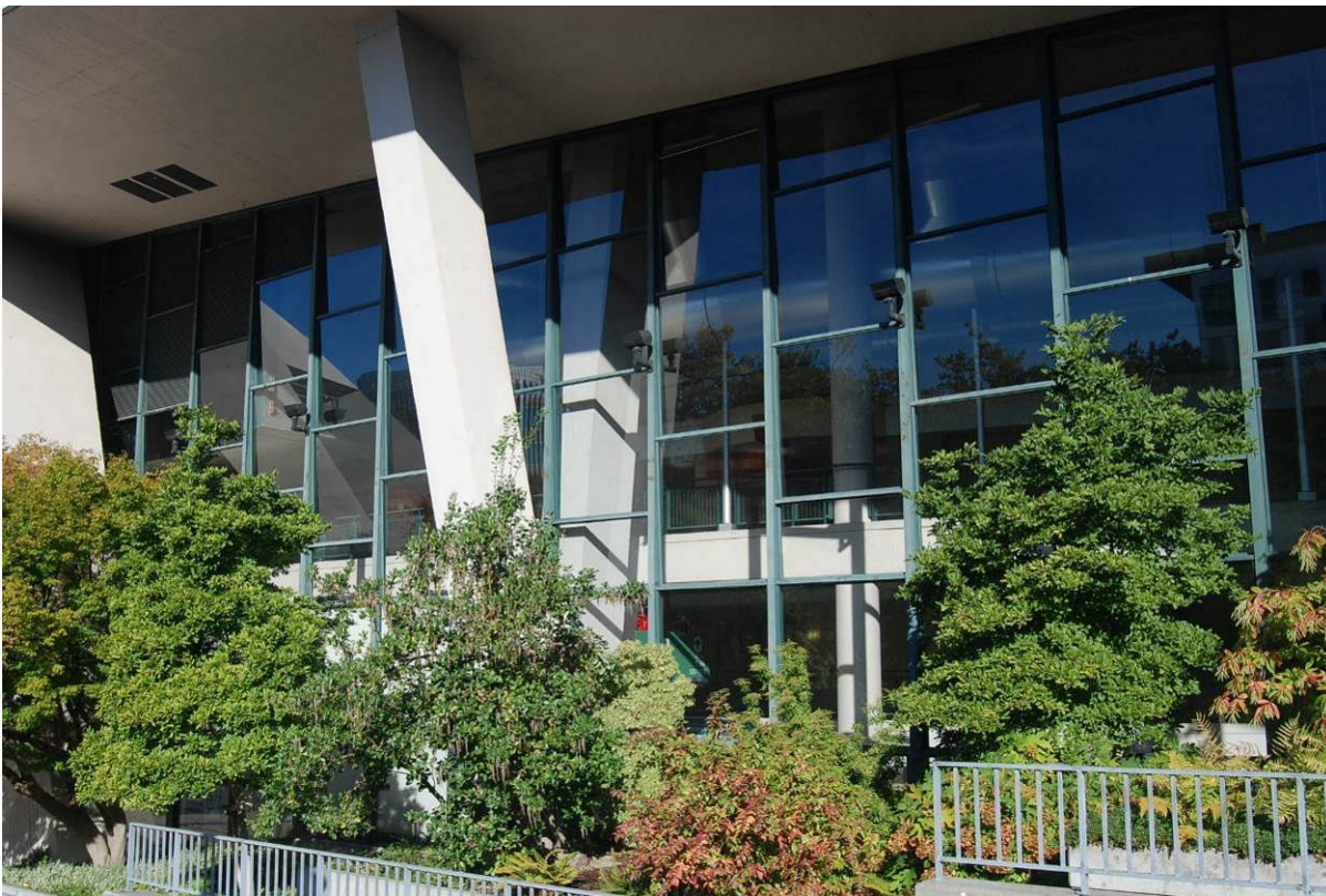
Photo 7 of 46 (WA_King County_Century 21 Coliseum_0007) – October 2017 Detail view of the curtain wall and v-shaped piers on the west façade, facing east
