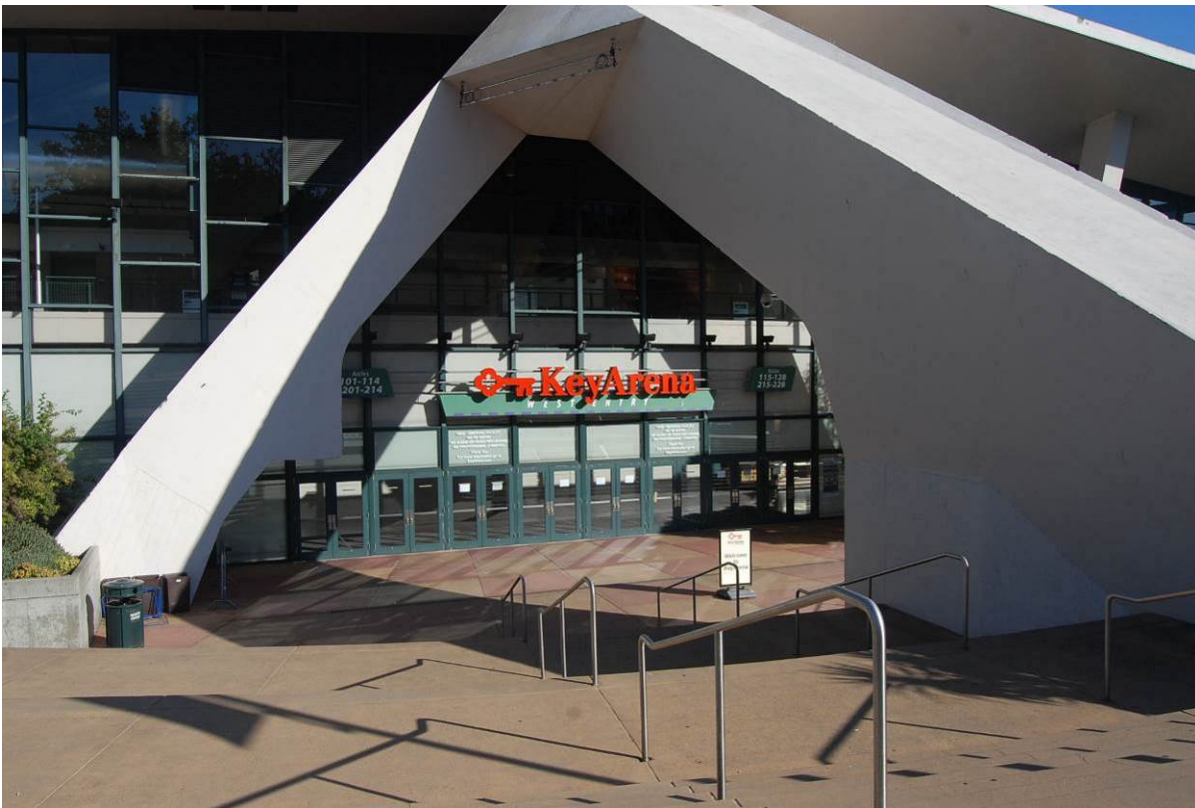
Photo 5 of 46 (WA_King County_Century 21 Coliseum_0005) – October 2017 Detail view of the tripod concrete buttress and entrance on the west façade, facing east
