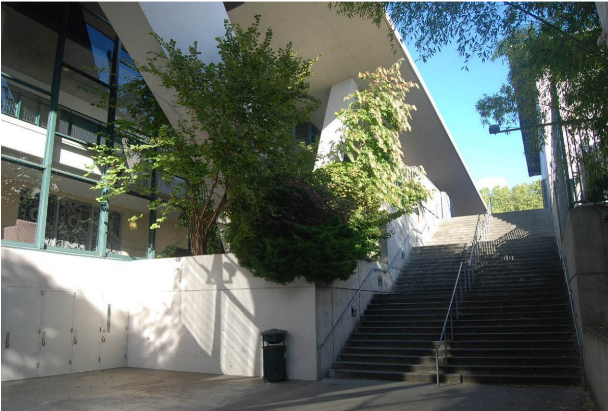
Photo 14 of 46 (WA_King County_Century 21 Coliseum_0014) Detail view of stairs on the south façade, facing east
