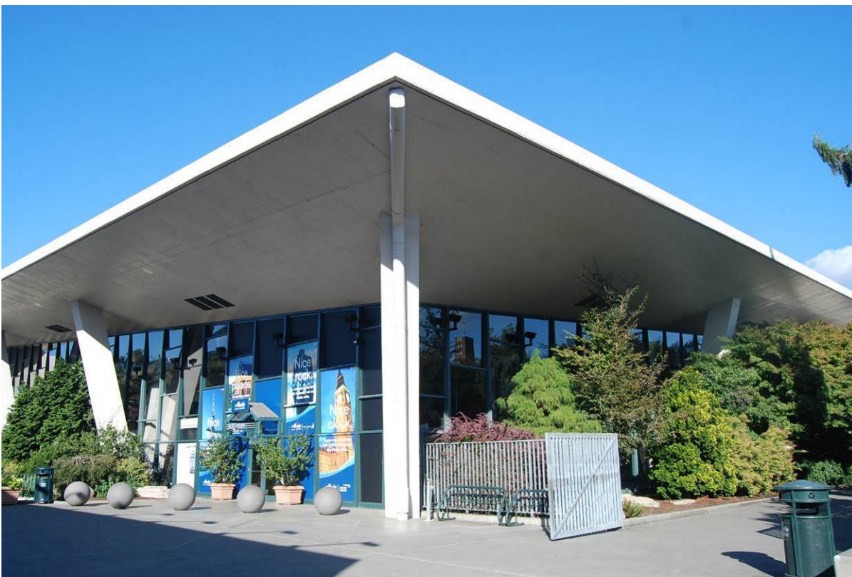
Photo 9 of 46 (WA_King County_Century 21 Coliseum_0009) – October 2017 Oblique view of the west and south facades, facing northeast
