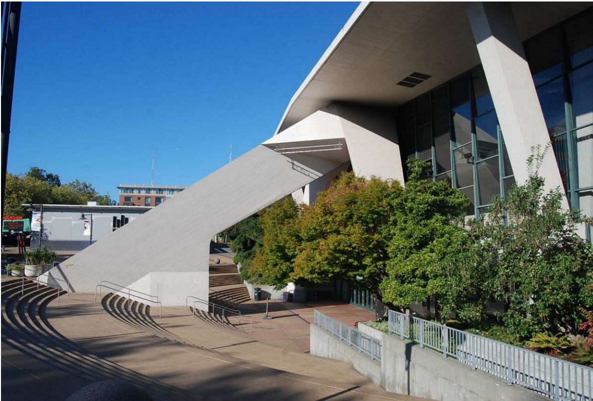
Photo 8 of 46 (WA_King County_Century 21 Coliseum_0008) – October 2017 Detail view of the tripodal concrete buttress on the west façade, facing north
