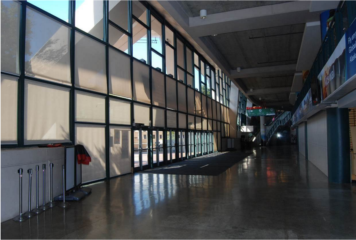
Photo 28 of 46 (WA_King County_Century 21 Coliseum_0028) – October 2017 Interior of the west entrance, main concourse level, facing north
