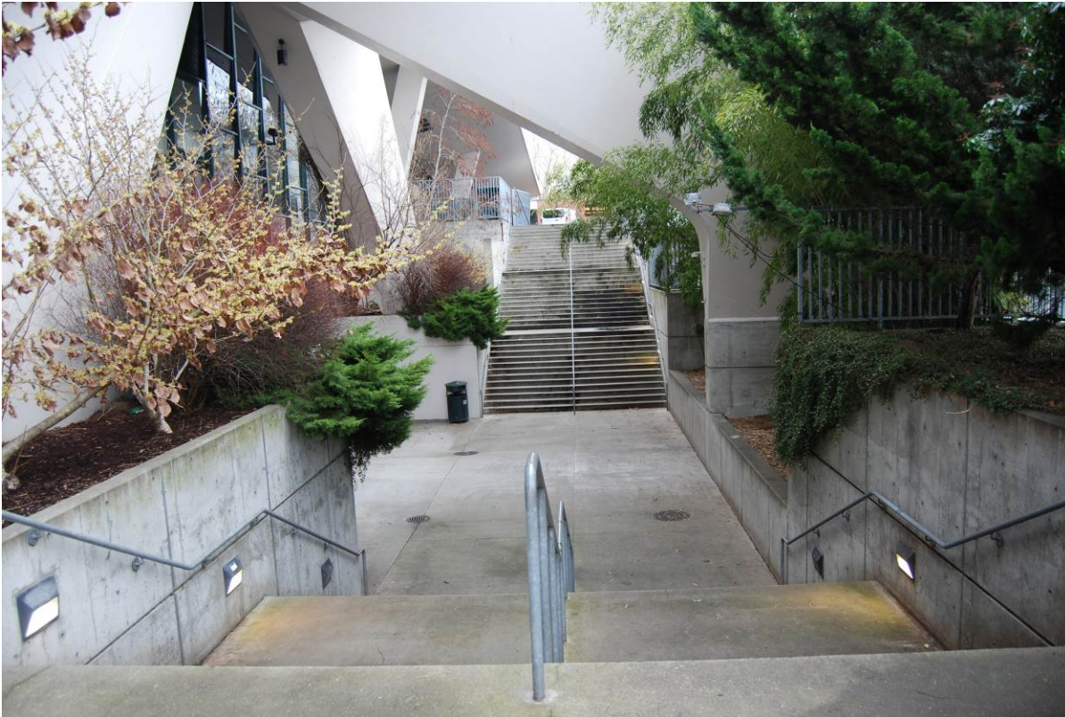
Photo 11 of 46 (WA_King County_Century 21 Coliseum_0011) – October 2017 Detail view of the stairs along south façade, facing east
