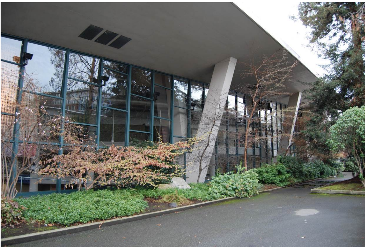
Photo 23 of 46 (WA_King County_Century 21 Coliseum_0023) – February 2017 Detail view of the curtain wall and V-shaped piers on the north façade, facing southwest
