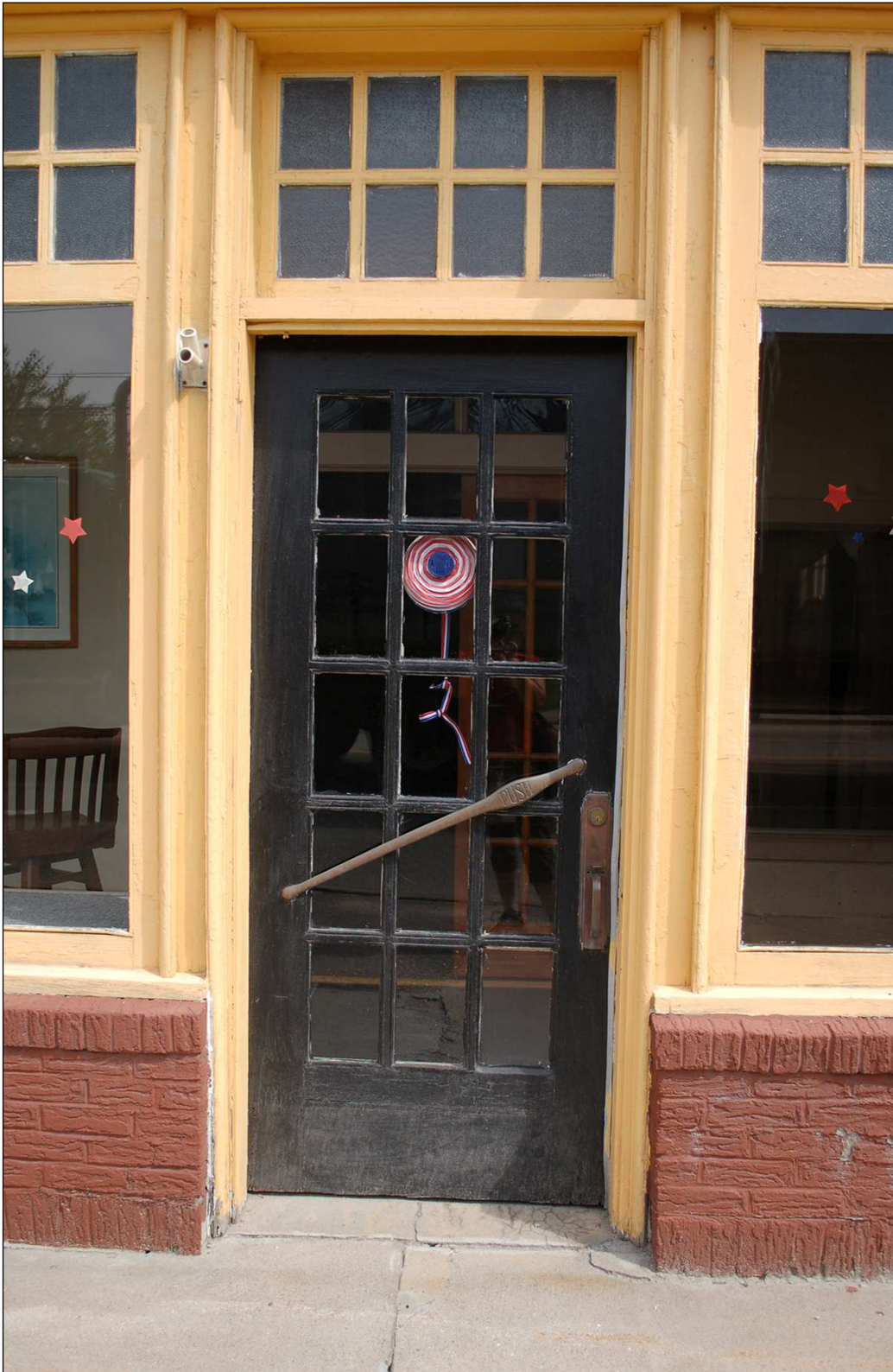
Photo 0004: Detail of store entrance door with historic door hardware, facing north
