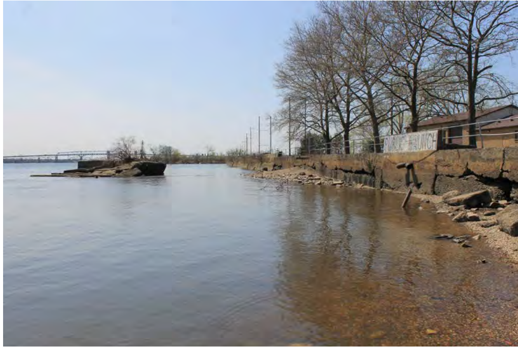
Photograph 43: Overall view of the bank of the Delaware River, facing southwest. Building No. 409 (Laboratory Storage) is visible to the left; a sea wall that appears to be contemporary with the arsenal is visible to the right. The Boat Launch Area maintenance building is also visible to the right.
