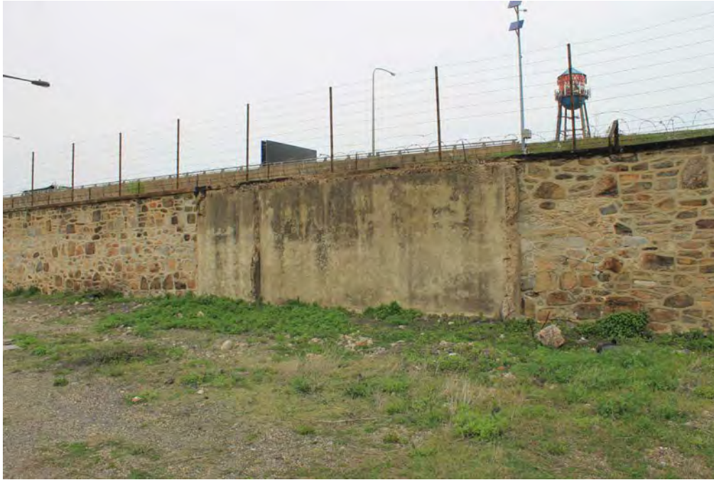
Photograph 5: View of what was historically the north wall of Building Nos. 60 and 61 (both, Inflammable Materials Storehouses), facing northwest. Note it appears to be attached to the stone boundary wall along Tacony Street. Building Nos. 60 and 61 were demolished c.1980.
