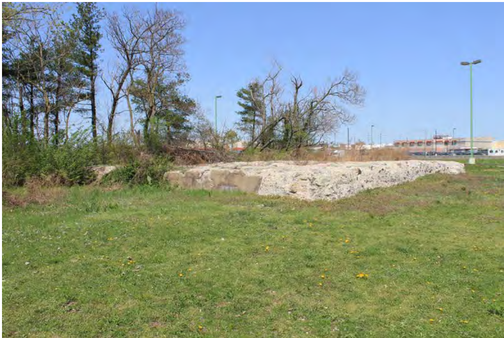
Photograph 16: View of the Building No. 334 (High Explosive Magazine) ruins, facing northeast. Note the small section of wall that retains its historic finished surface just left of center, and the brick infill to the right of center.
