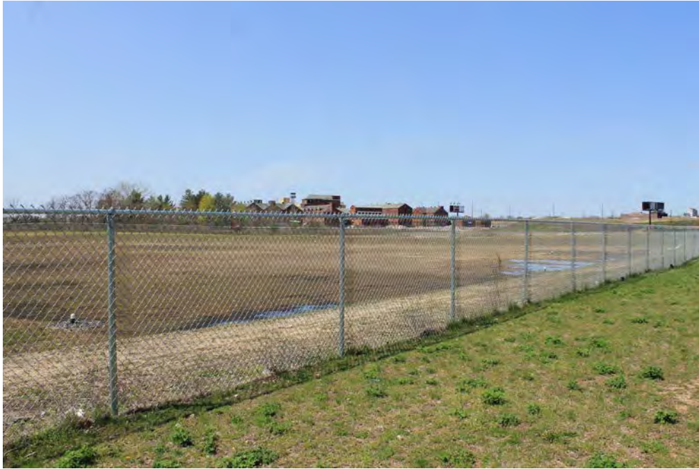
Photograph 37: Overall view of the now-vacant area of the Frankford Arsenal, facing northwest. The circa-2015 retention pond is to the left behind the chain-link fence; the extant portion of the arsenal is visible in the background.
