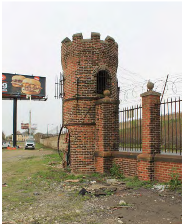
Photograph 10: View of the Machine Gun Tower (Building No. 49), facing northwest.
