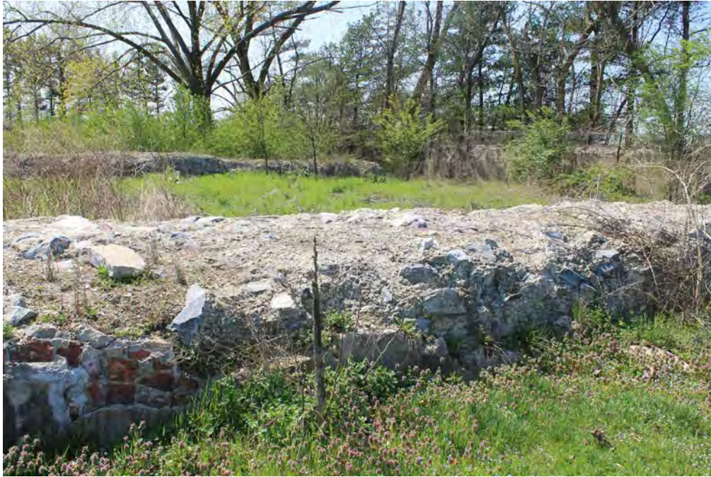
Photograph 17: View of the Building No. 334 (High Explosive Magazine) ruins, facing west. Note the small section of brick infill at the left. The separate, north blast wall, which stands 6-7 feet in height, is visible in the back right.
