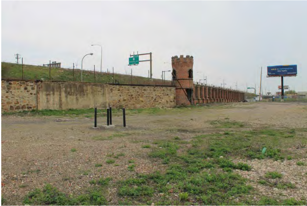
Photograph 9: View of the south face of the Tacony Street boundary wall, facing northeast. Note the remains of Building Nos. 60 and 61 (both Inflammable Materials Storehouses) to the left (within the stone portion) and the Machine Gun Tower (Building No. 49) just right of center. Building Nos. 60 and 61 were demolished c.1980.
