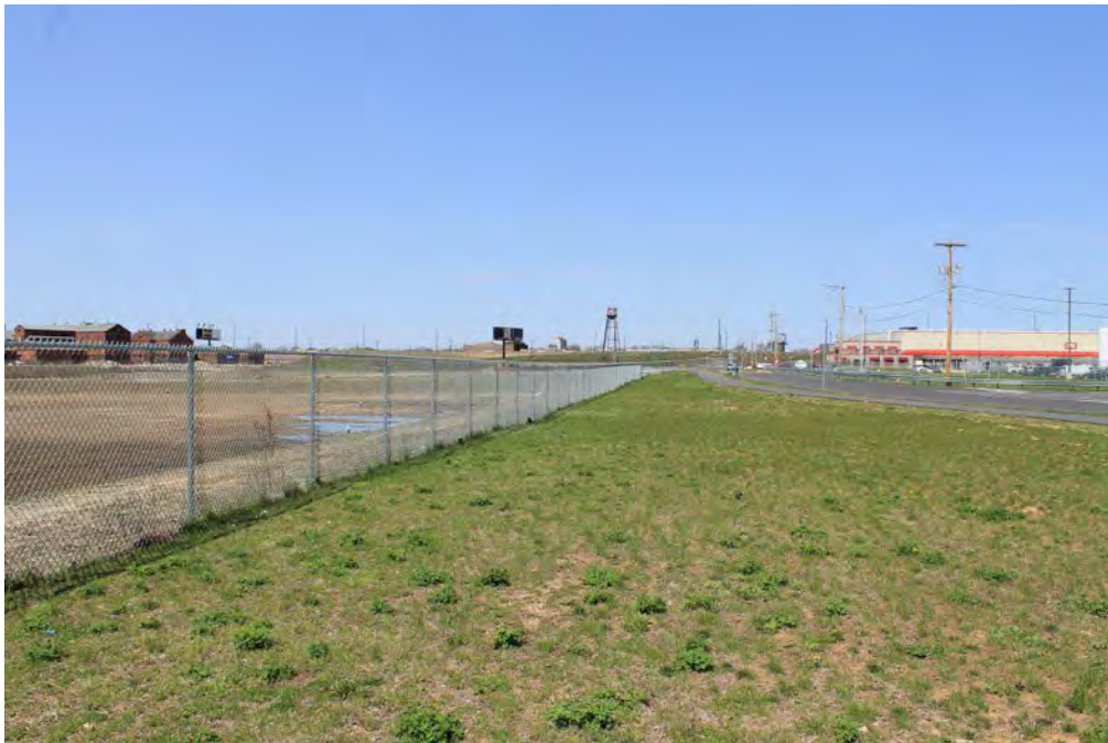
Photograph 38: Overall view of the Frankford Arsenal, facing northwest. The extant portion of the arsenal is visible to the far left; the now-vacant area is visible to the left and center; and the redeveloped portion is visible to the right.
