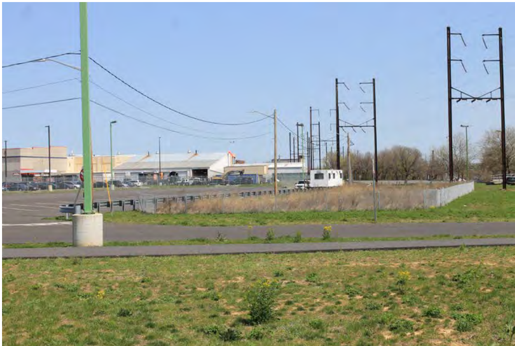
Photograph 40: Overall view of the redeveloped portion of the Frankford Arsenal, facing northeast. The new parking lot for the Boat Launch Area is visible to the left; the access road is in the foreground.
