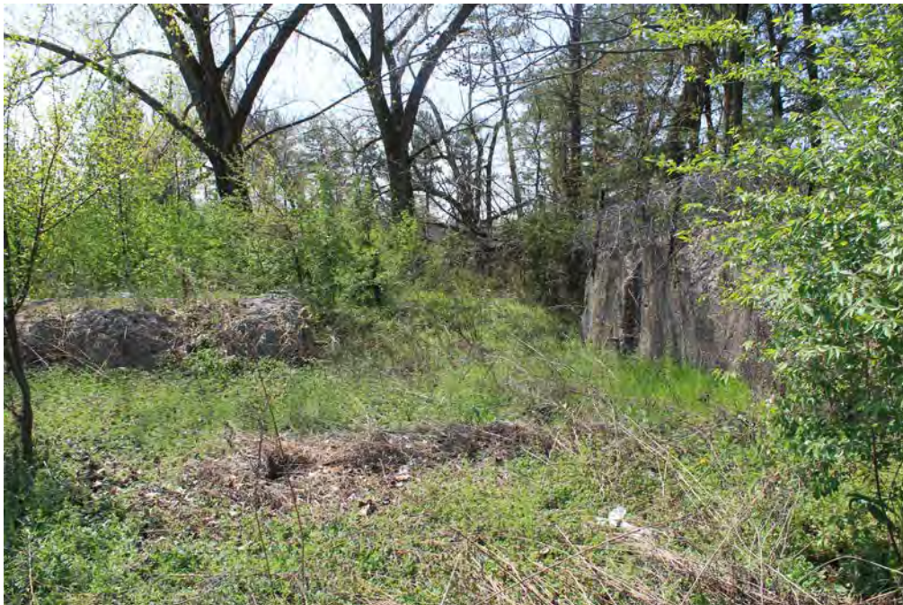
Photograph 18: View of the Building No. 334 (High Explosive Magazine) ruins, facing west. Note the gap between the west and north parts of the blast wall. Just visible are what appear to be iron mounts for some type of gate.
