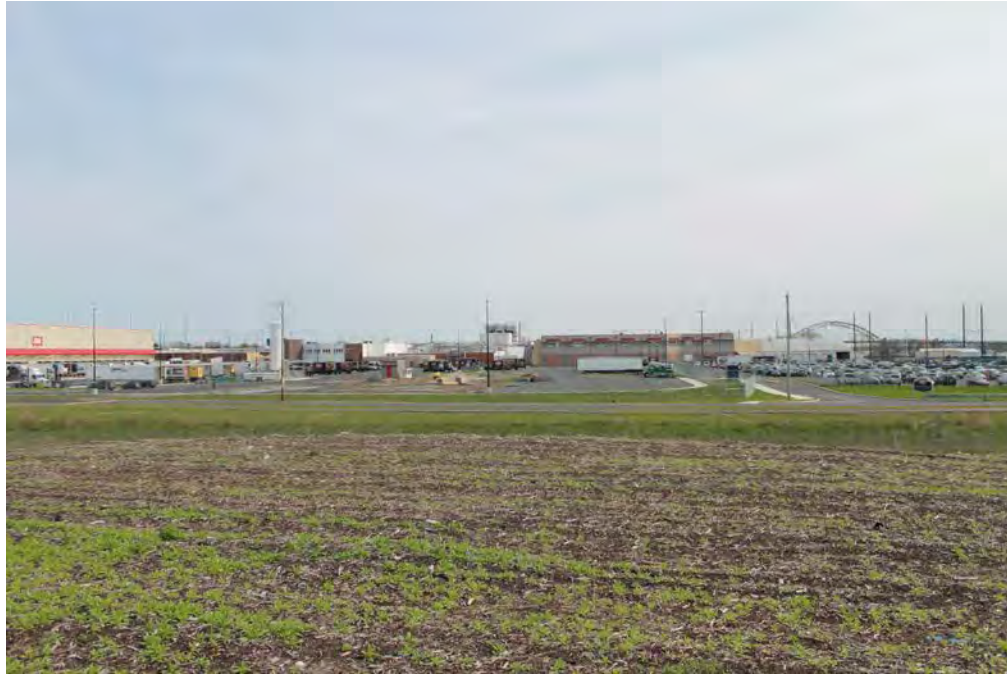
Photograph 35: Overall view of the redeveloped area of the Frankford Arsenal, facing east. The new Dietz & Watson Building (c.2015) is visible at the left; its parking lot is in the center and right; and the old Dietz & Watson building is in the background.
