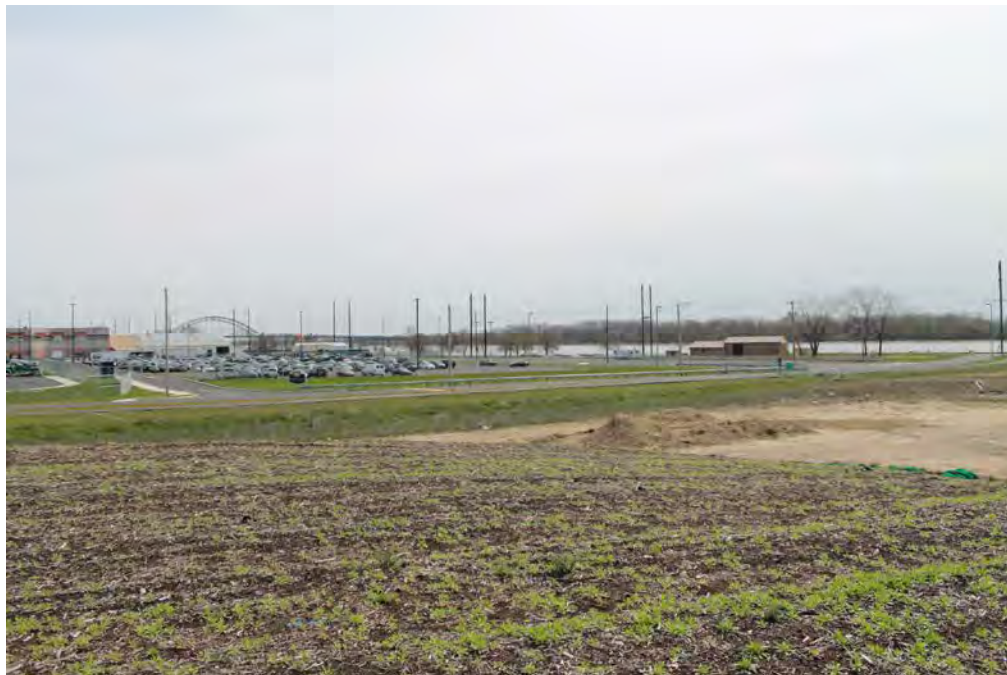
Photograph 34: Overall view of the now-vacant and redeveloped areas of the Frankford Arsenal, facing southeast. The older Dietz & Watson building (c.1995) located outside of the arsenal boundaries is to the left; the new (c.2015) Dietz & Watson and Boat Launch Area parking lots are in the center; the Boat Launch Area is to the right.
