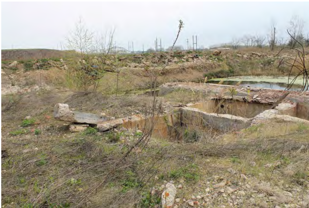
Photograph 6: View of the remaining basement walls of Building No. 301 (Heating Plant), facing southeast. This building was demolished c.2012.
