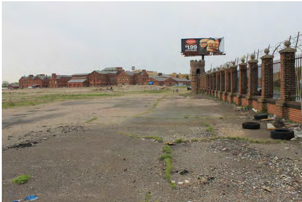
Photograph 26: Overall view of the now-vacant area of the Frankford Arsenal from the intersection of Tacony Street and the current Boat Launch Area access road, facing west. The Tacony Street boundary wall and the Machine Gun Tower (Building No. 49) are visible to the right; the extant portion of the arsenal is visible in the background.
