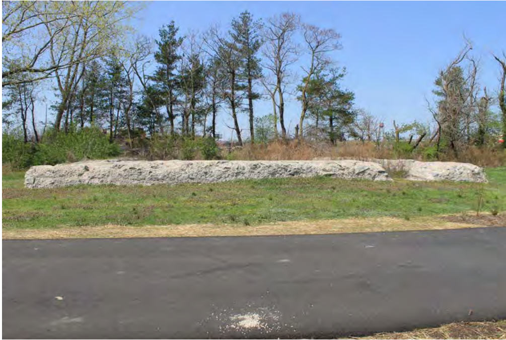
Photograph 15: View of the Building No. 334 (High Explosive Magazine) ruins, facing northwest. The visible walls are about 3-4 feet in height; note the doorway-type opening toward the right of the photograph.
