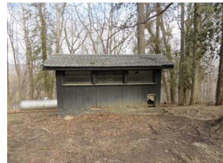
Animal Shelter, camera facing north
