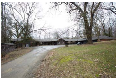
Main House, camera looking east
