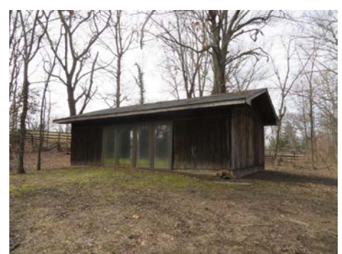
Carriage Storage Building, to west
