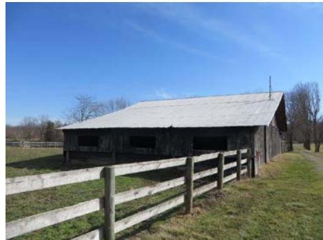
Six-stall Barn, to south
