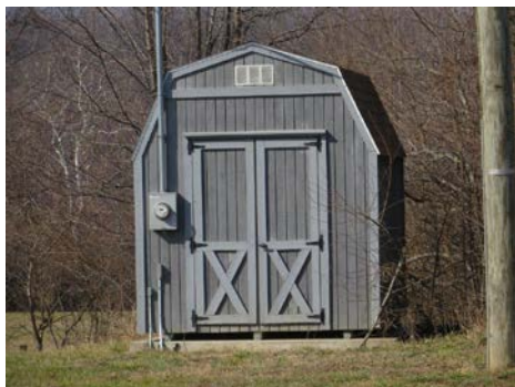
Prefabricated shed, to north
