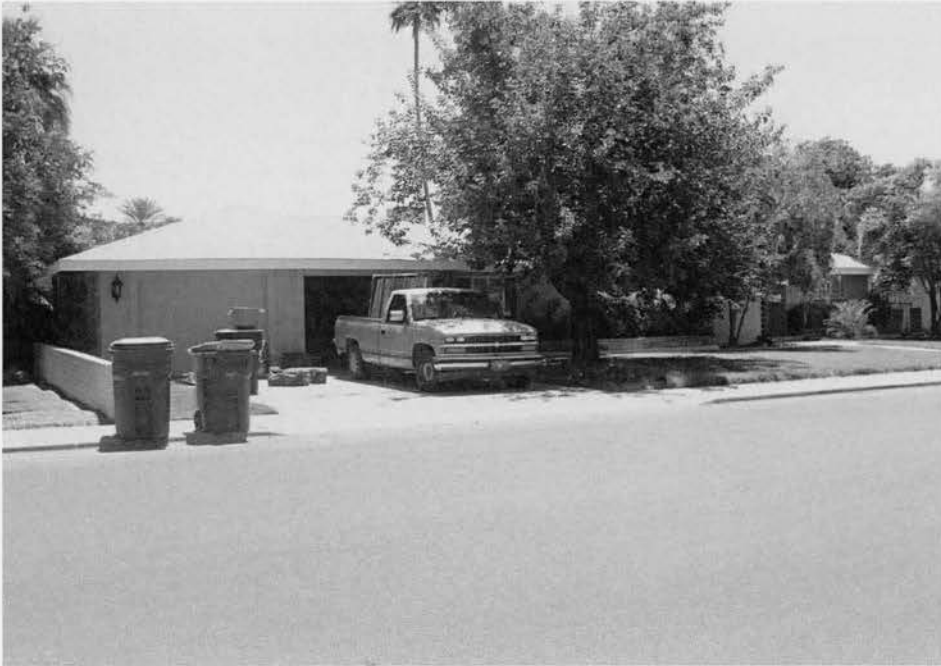
Evans House 136 N. Fraser Drive (Ryden Architects, 2005)
