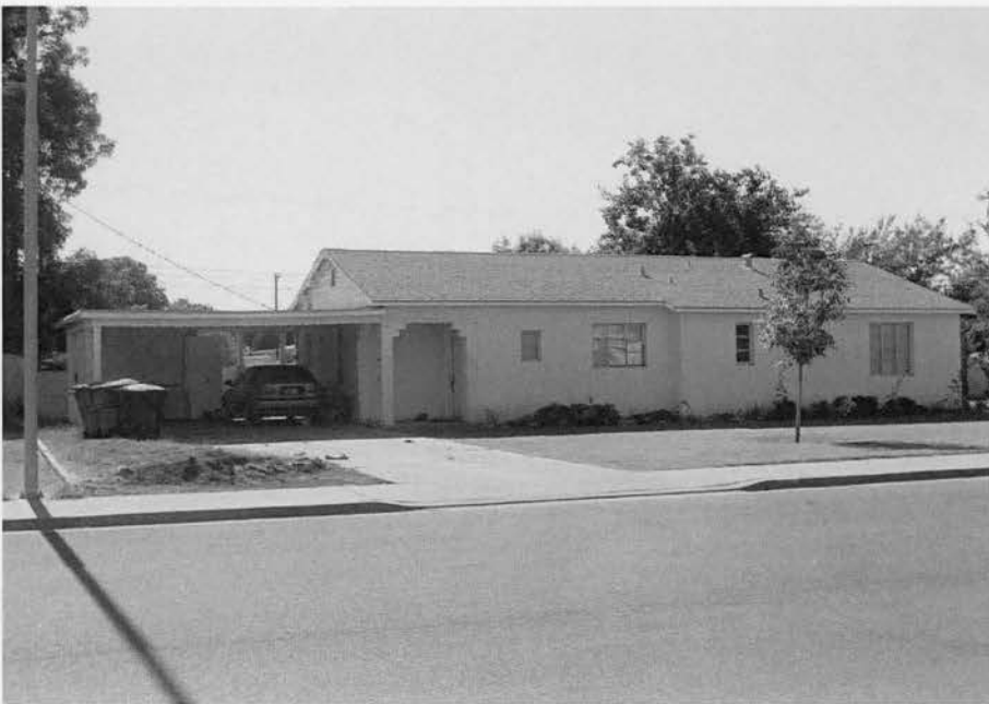
Van Kirk House 103 N. Fraser Drive East, F-017 ( Ryden Architects, 2005 )
