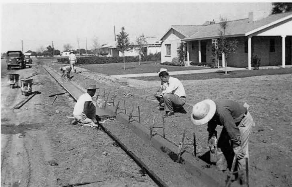
Construction of curbs in Fraser Fields, 1954 (Mesa Southwest Museum, Photo 98-455.86)
