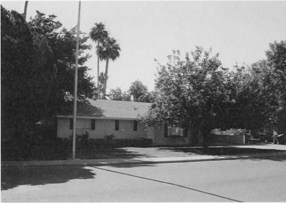
Ewart House 57 N. Fraser Drive East, F-019 (Ryden Architects, 2005)
