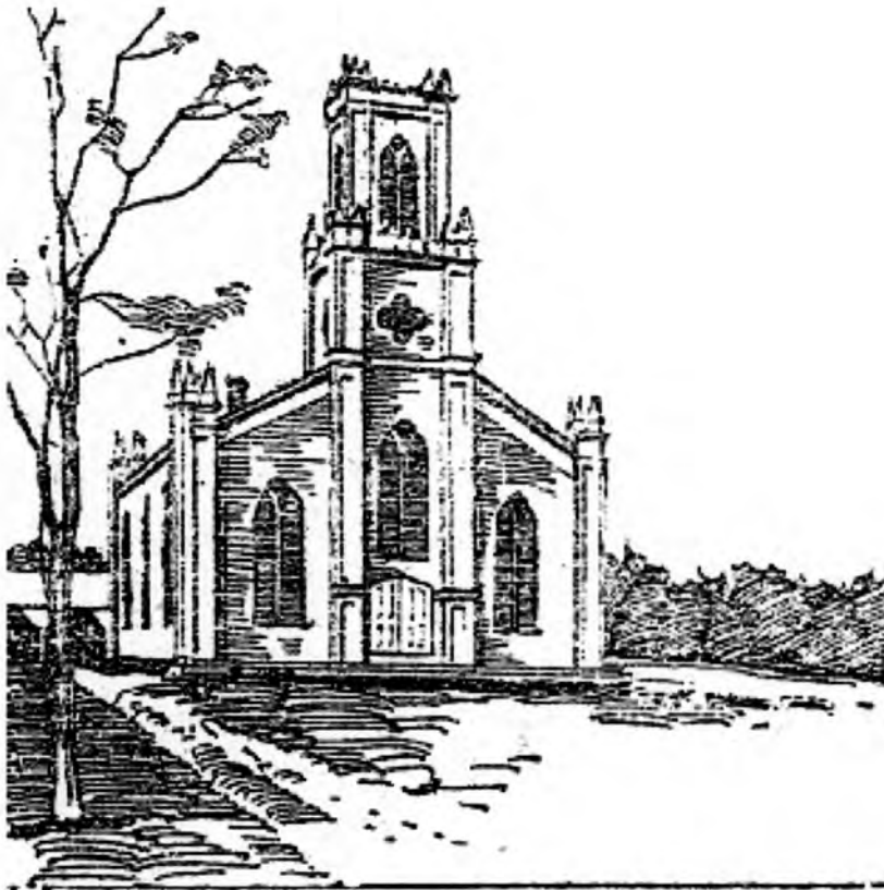
CONGREGATIONAL CHURCH AT ROCHESTER CENTRE.
