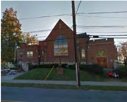
Bardstown Presbyterian Church
