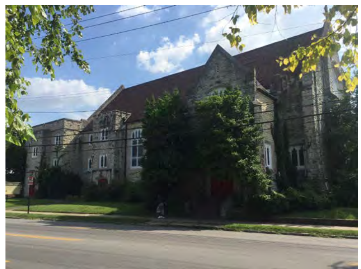
Northeast façade, along Bardstown Road
