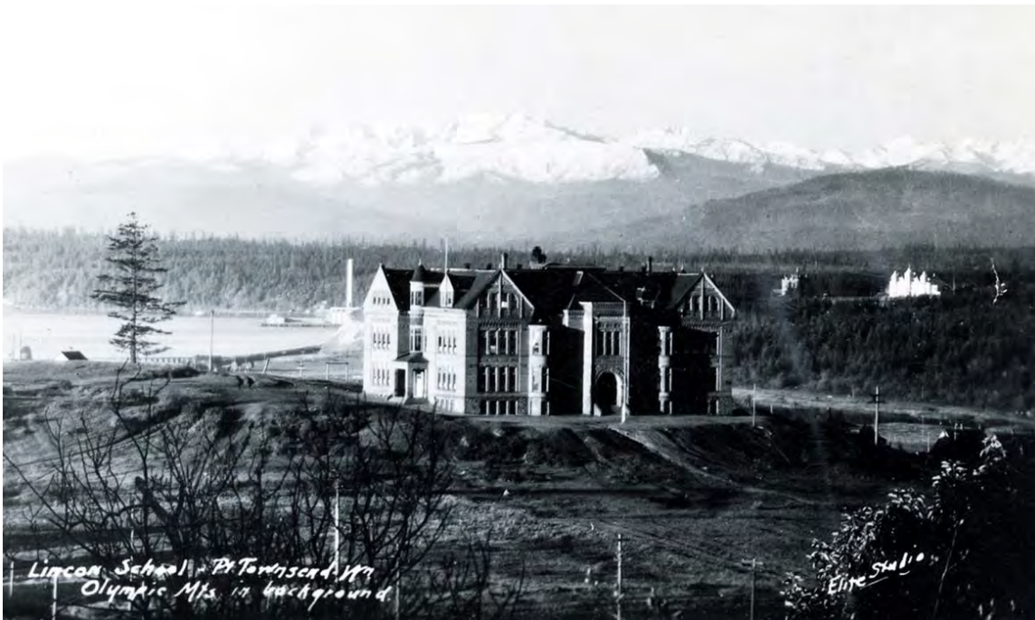
Lincoln School after tower was removed, facing north, c. 1928.
