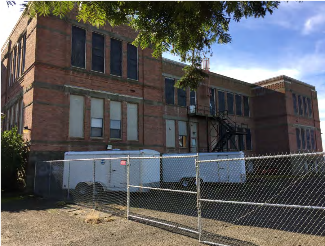
2 of 11 Lincoln School, north side, Northeast corner
