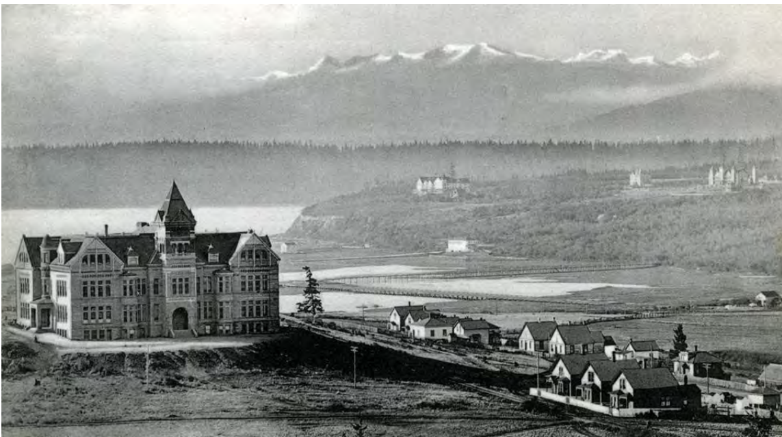
Lincoln School after 1899 with lowered clock tower, view facing north.
