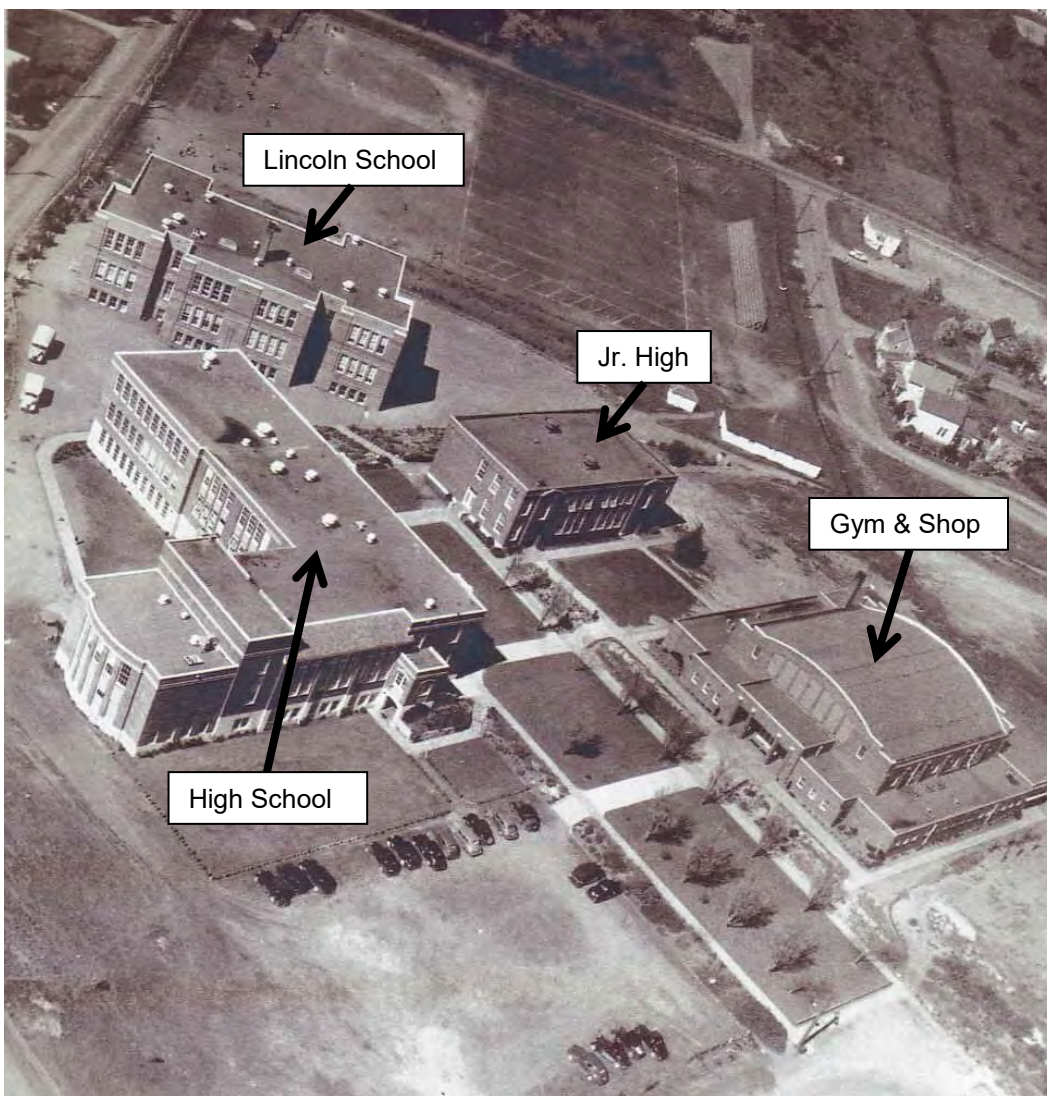
Aerial view of Public School Group, Port Townsend, c1950.
