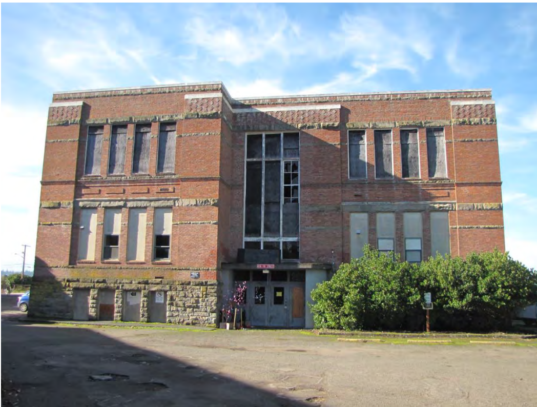
3 of 11 Lincoln School, East entrance
