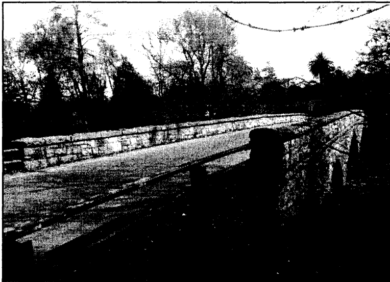
Photo No. 5 Deck and south elevation, from the west
