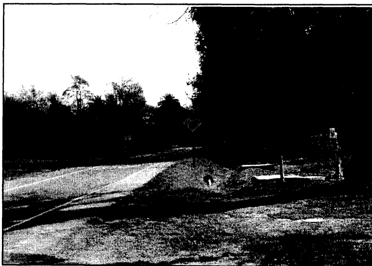
Photo No. 6 Roadway and deck, from the west
