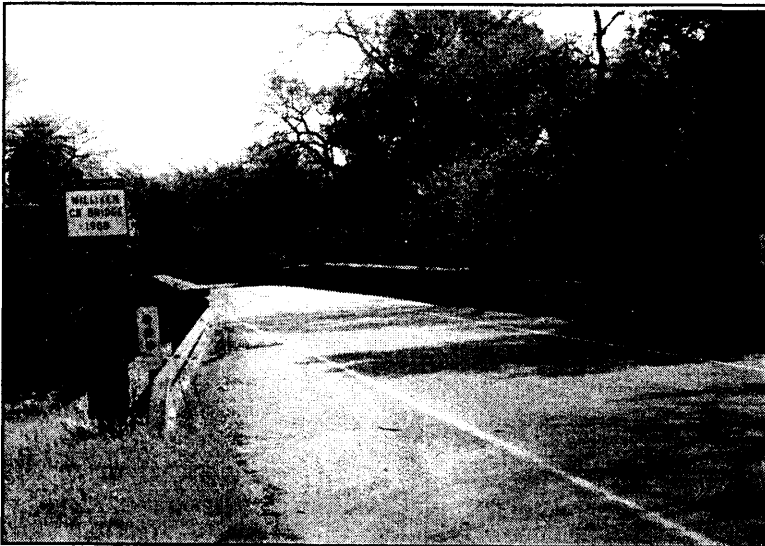
Photo No. 4 Deck, from the west
