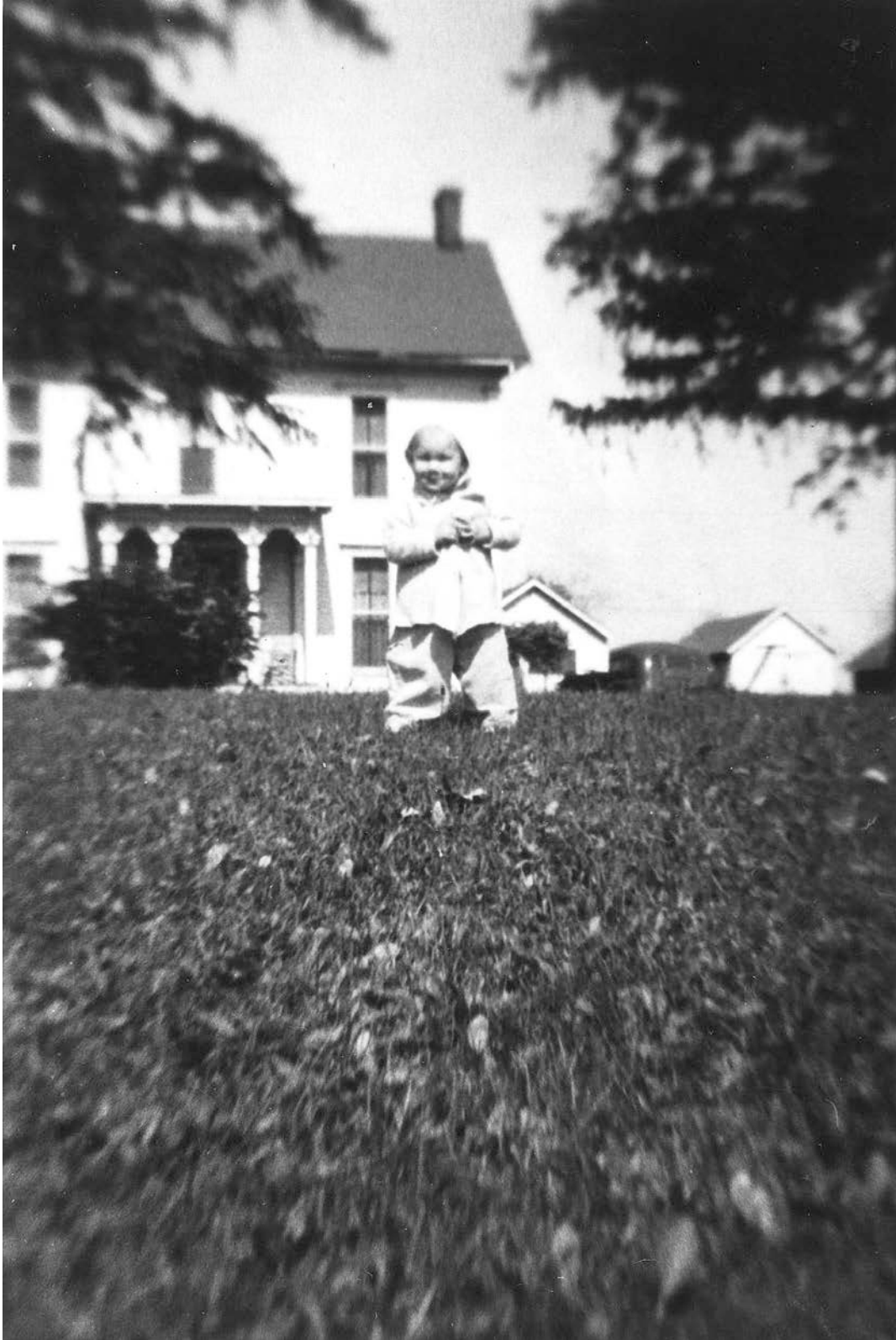
Figure 2: East elevation of Carter-Randall-Parker House with view of milking parlor and other outbuildings no longer extant; c.1945
