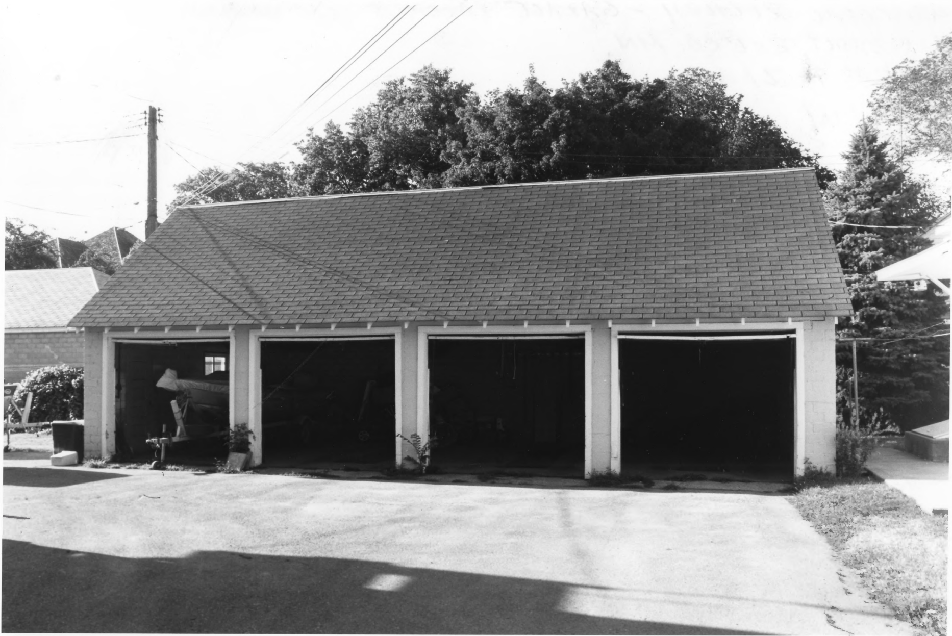
EPISCOPAL RECTORY GARAGE FARIBAUT RICE CO., MN PHOTO I.D. 09930 #24A
