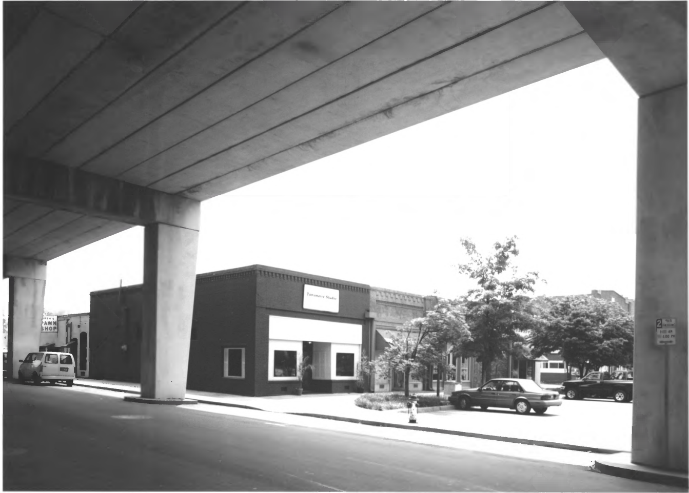
N. WALL STREET HISTORIC DISTRICT BARTOW COUNTY, GEORGIA 5 OF 7
