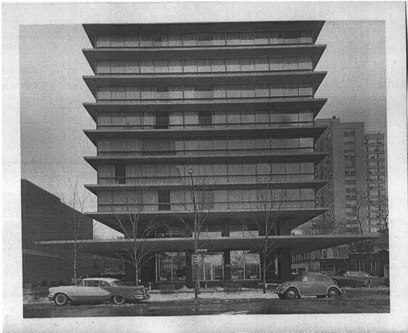
Figure 13: 320 West Oakdale after completion. Photography by Hedrich-Blessing, c. 1956. Collection of Robert Brueggemann.
