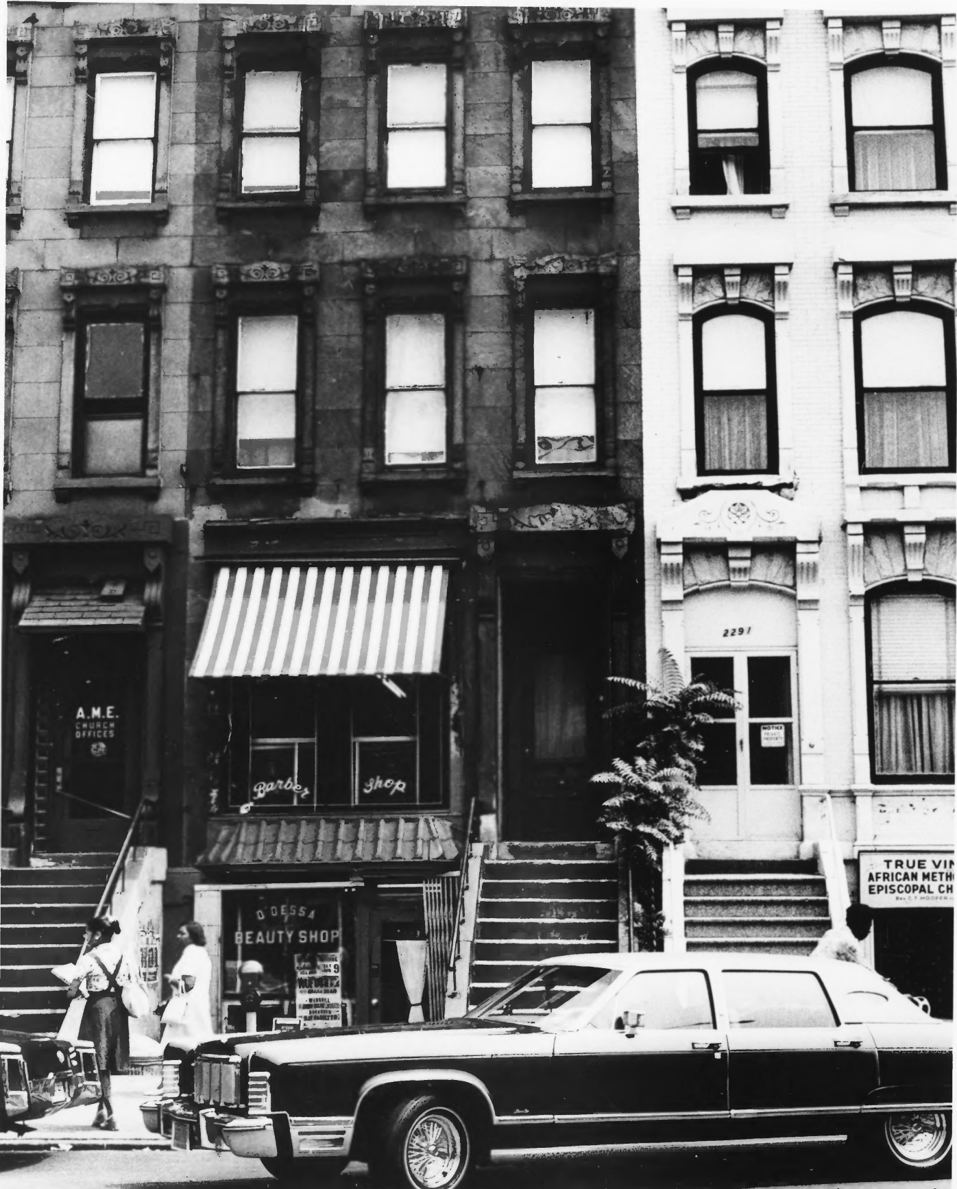
The New York Amsterdam News Building, New York, N.Y. Photo by Richard K. Dozier for the ABC (Middle Building) Front elevation
