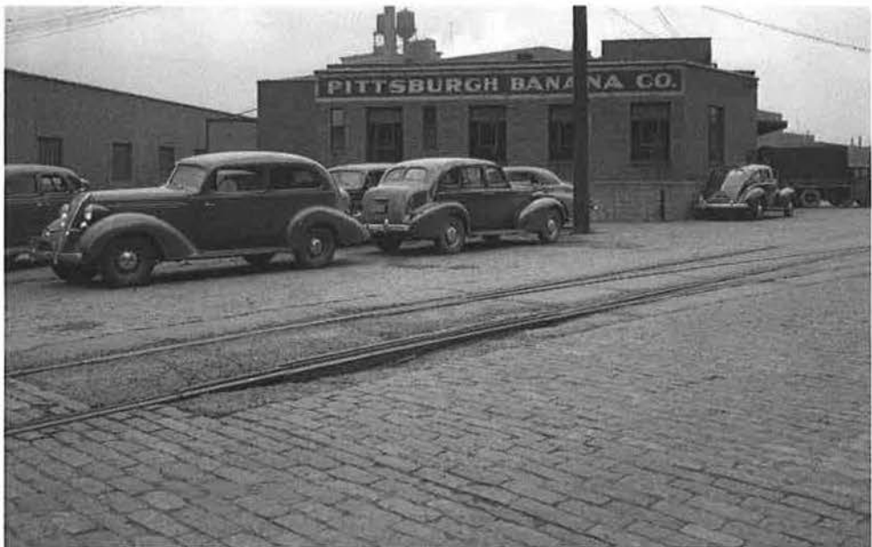
Figure 42: 1940 – Looking northeast along Smallman Street from 21st Street – repair at the railroad switch.
