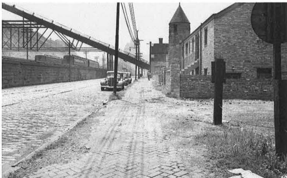
Figure 15: 26 July 1937 – Looking southwest along Liberty Avenue toward St. Patrick's Church (67 17 th Street) and the Penn Incline.
