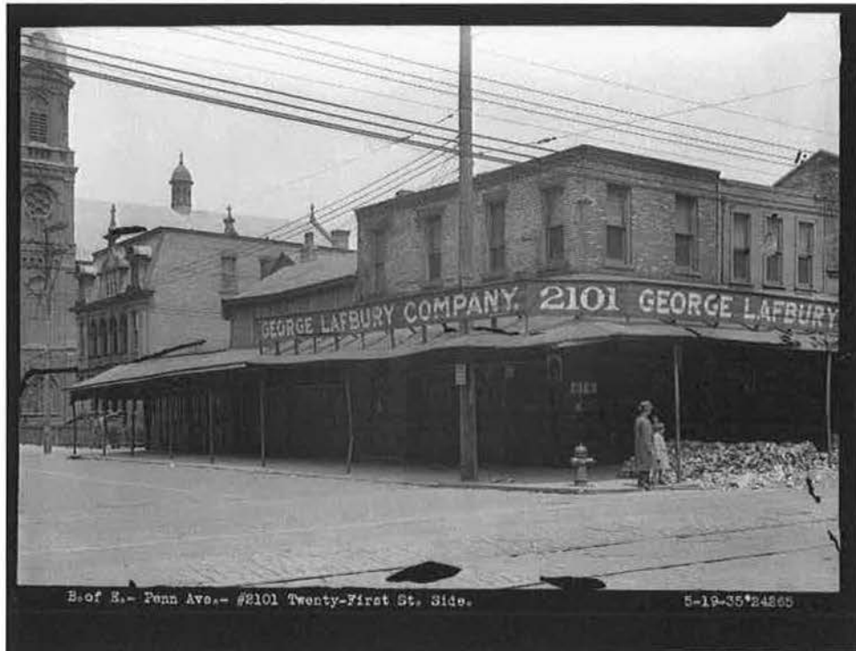
Figure 28.2: 1935 – Looking north at the north corner of Penn Avenue and 21st Street, 2101 Penn Avenue. St. Stanislaus Church and Rectory in the background.
