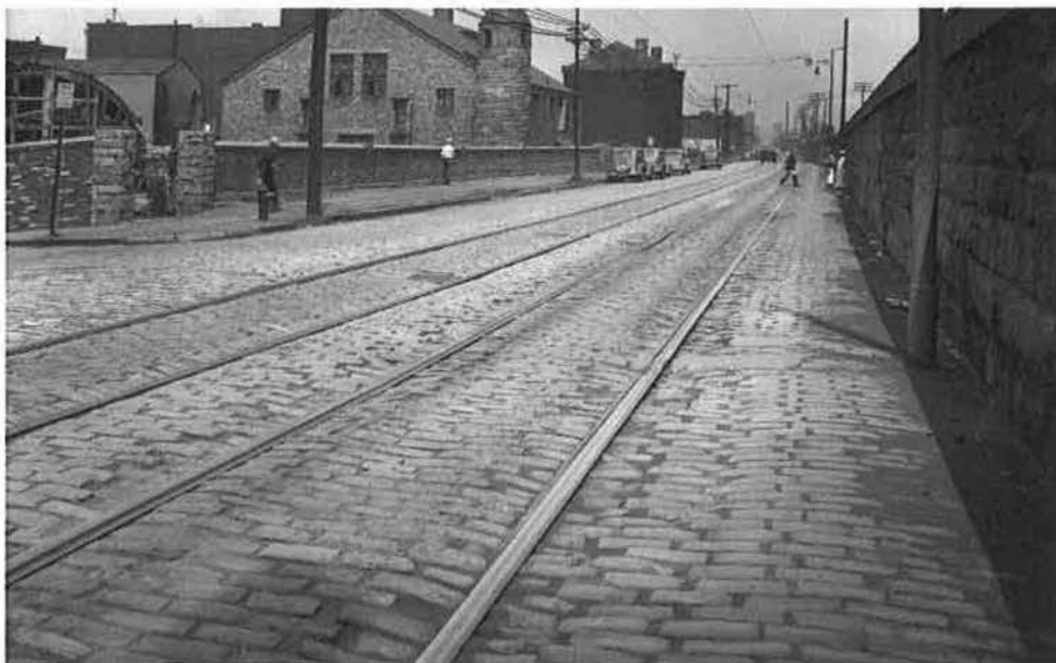
Figure 14: 26 July 1937 – Looking northeast along Liberty Avenue toward St. Patrick's Church (67 17 th Street) and 17 th Street.
