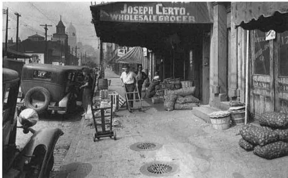
Figure 23: 22 July 1937 – Looking southwest from 1715 Penn Avenue.
