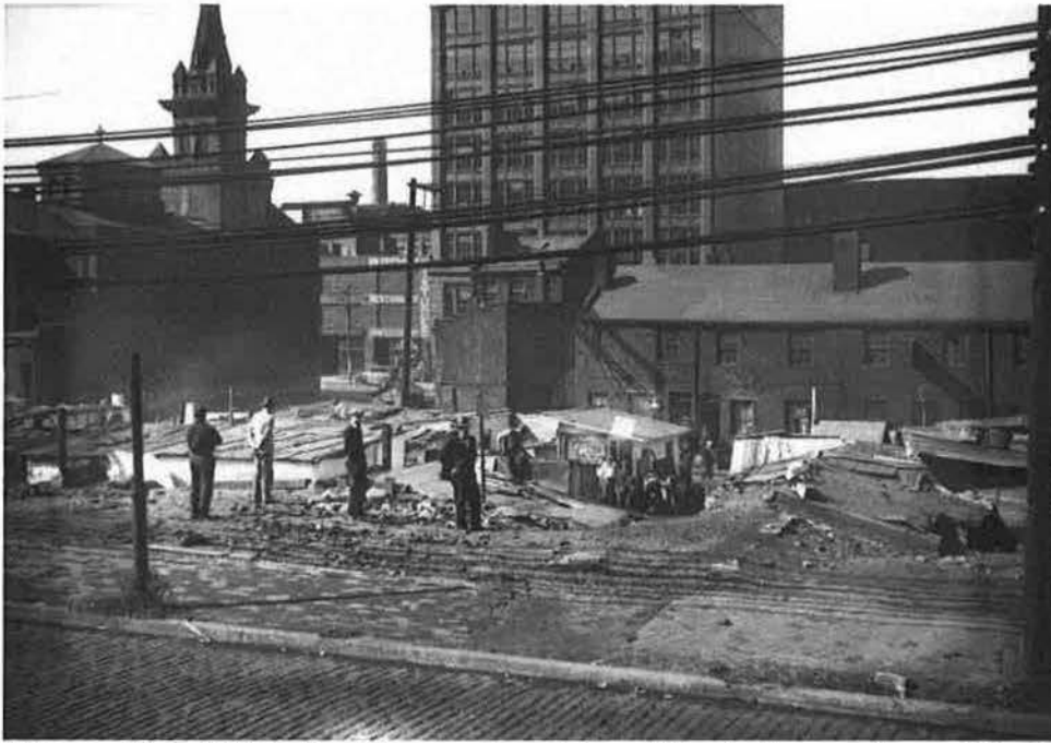
Figure 43: c. 1930 – Looking northwest from Liberty Avenue toward Spring Way, between 16th and 17th streets. The Penn Rose Building (1627 Penn Avenue) and St. Elizabeth’s Church (1620 Penn Avenue) are visible in the photograph. Image depicts the Strip District Hooverville or shantytown, where unemployed homeless men found shelter in shacks in the foreground. A sign on the shack advertises the sale of “washing fluid,” and notes that “Profits go to Father Cox.”
