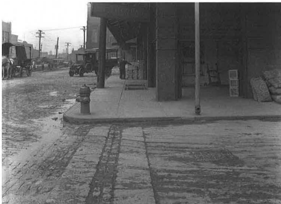
Figure 37: 25 March 1929 – Looking northeast along Pike Street (Smallman) from 20th Street toward James B. Catanzaro Building, 62 21 st Street.
