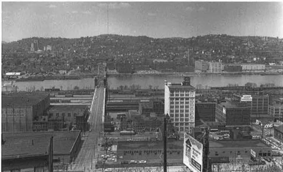
Figure 3: 9 May 1962 – View from the Upper Hill District.
