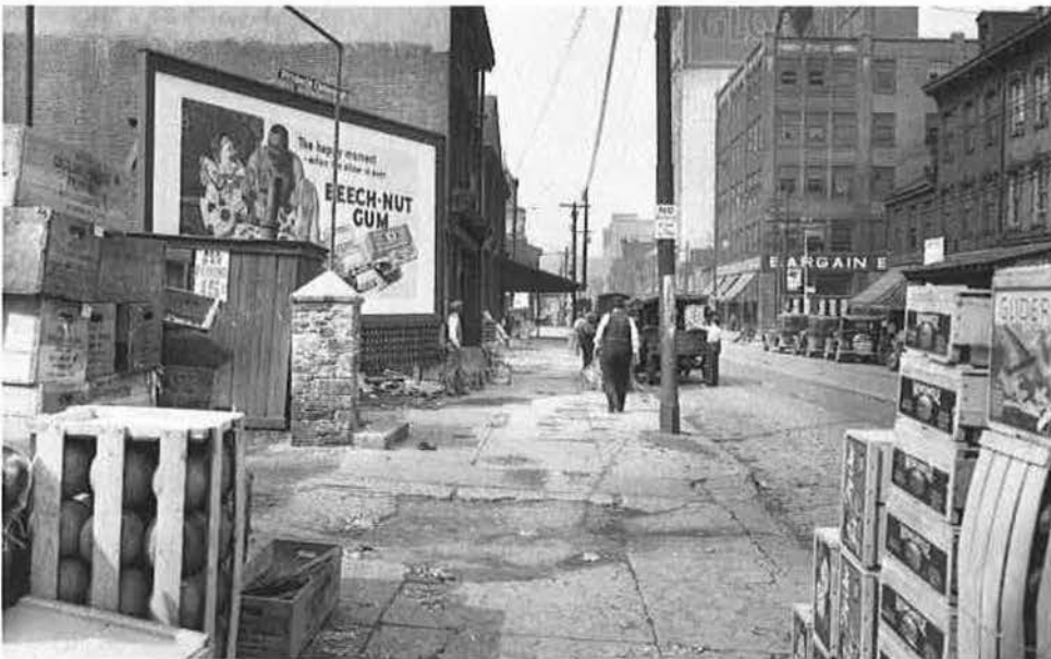
Figure 22: 22 July 1937 – Looking southwest along Penn Avenue from address 1725. 1649 Penn Avenue is visible to the upper right of the photograph, Butler’s Bargain Base, now Lotus Food Co.
