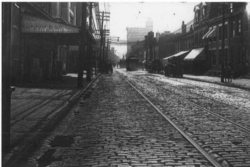
Figure 29: 28 July 1909 – View of storefronts and horse-drawn buggies on Penn Avenue near 21st Street.
