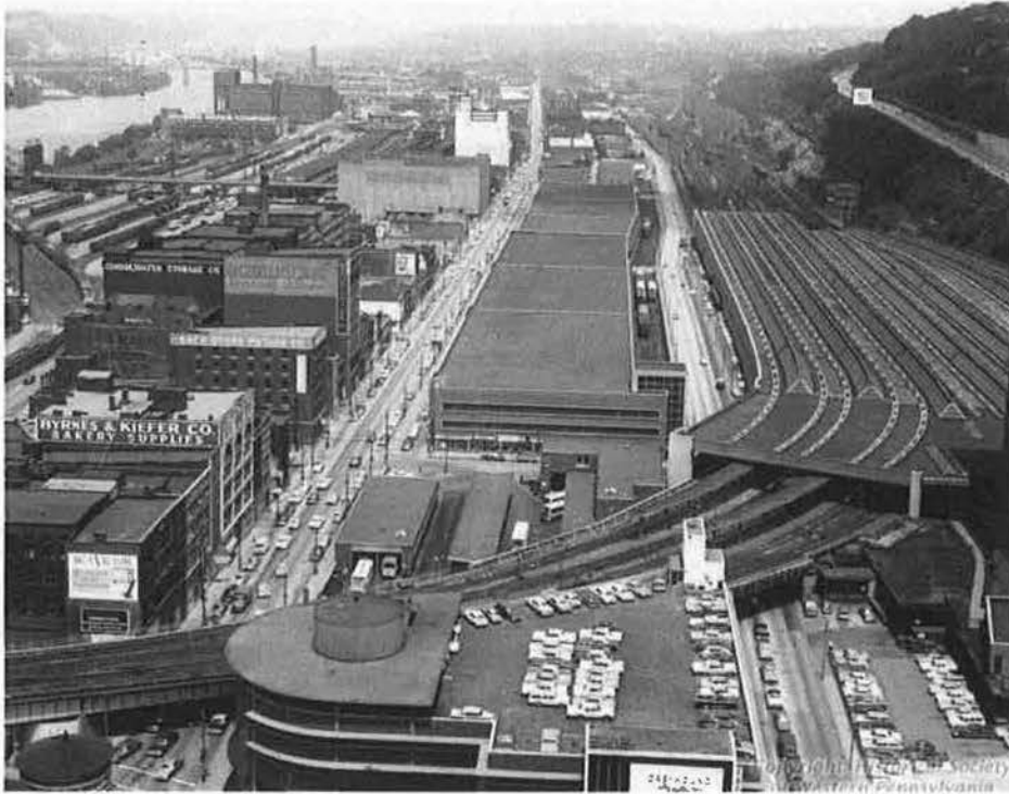
Figure 6: 1965-70 – Looking northeast along Penn and Liberty avenues toward the Strip District, in the distance.
