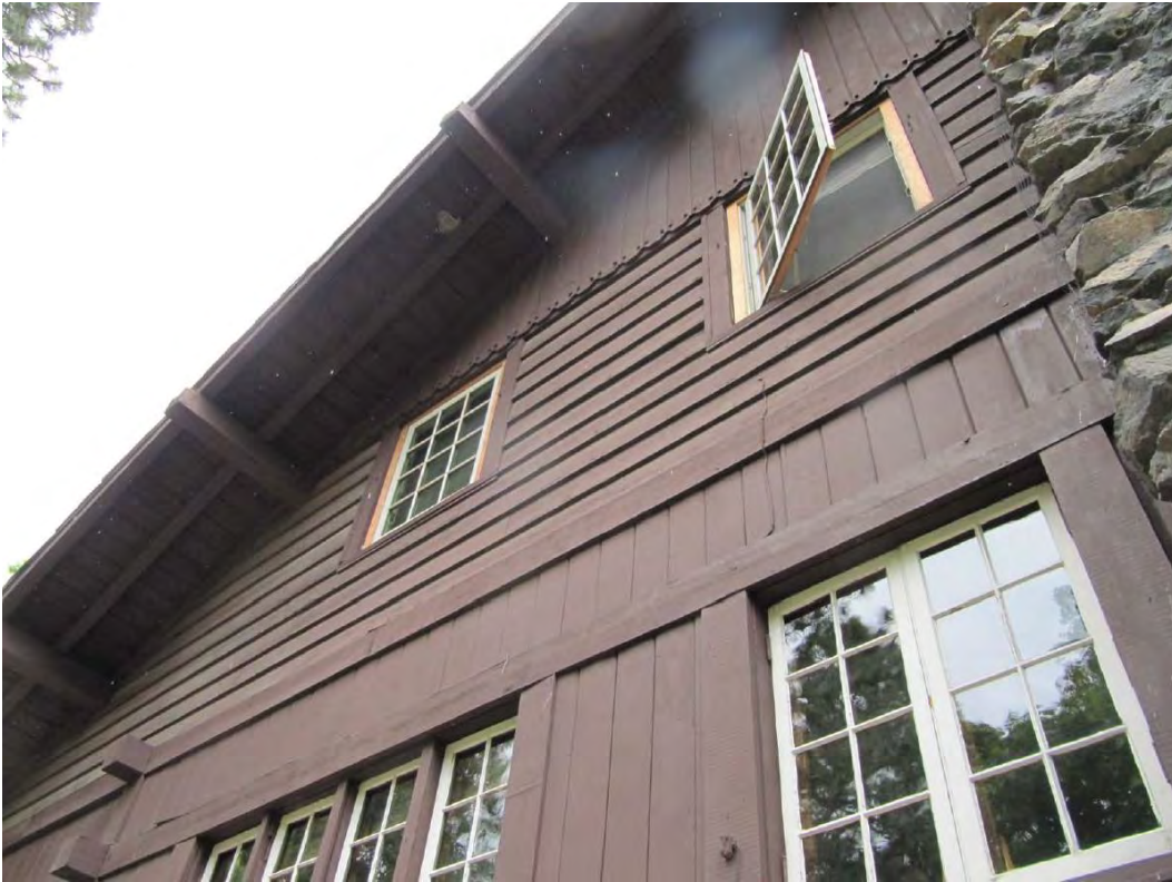
4 of 20: west gable peak detail
