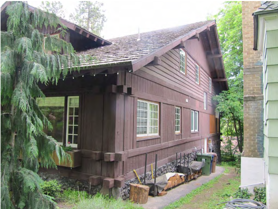
6 of 20 east face of house in 2014
