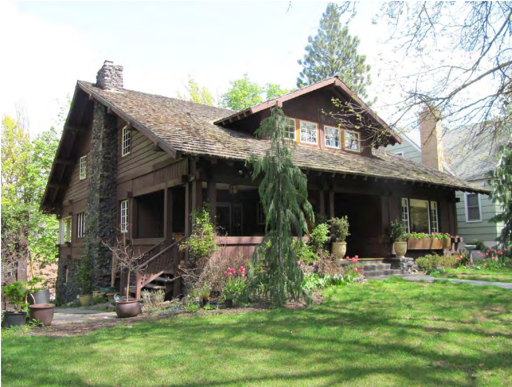
2 of 20: southwest corner of house in 2014
