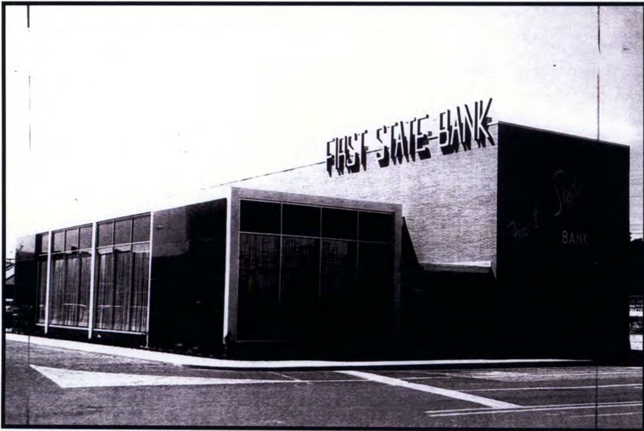
Figure 13. 1960 Photograph of the 1960 First State Bank (FA1076) at the corner of Front and Oak streets, viewing south. [Courtesy of the Faulkner County Historical Society Photograph Collection at the University of Central Arkansas.]
