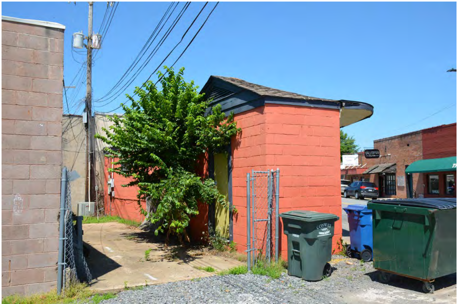
Figure 3: Current photograph of the building at 1015 Van Ronkle. (Photo date: June 2016.)
