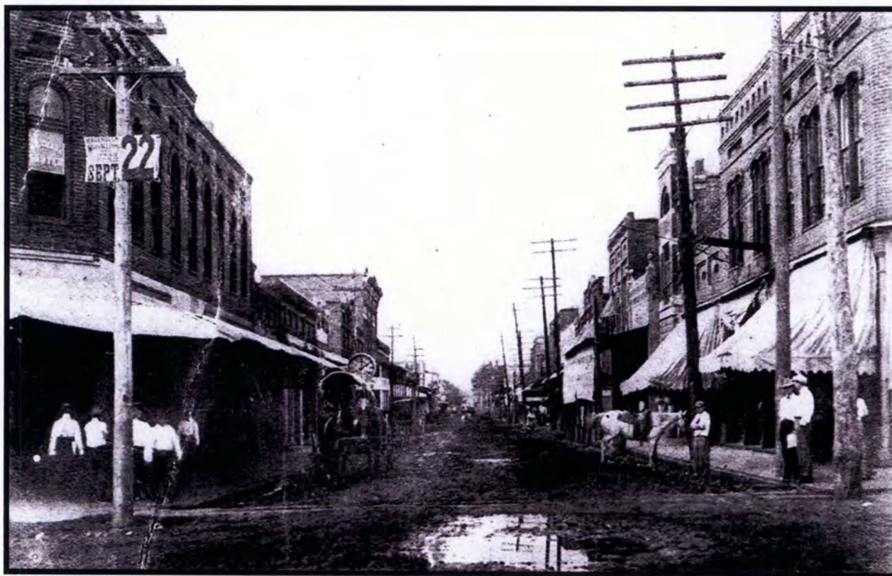
Figure 3. Front Street viewing north-northwest from Oak Street, ca. 1910. [Courtesy of the Faulkner County Historical Society Photograph Collection at the University of Central Arkansas.]
