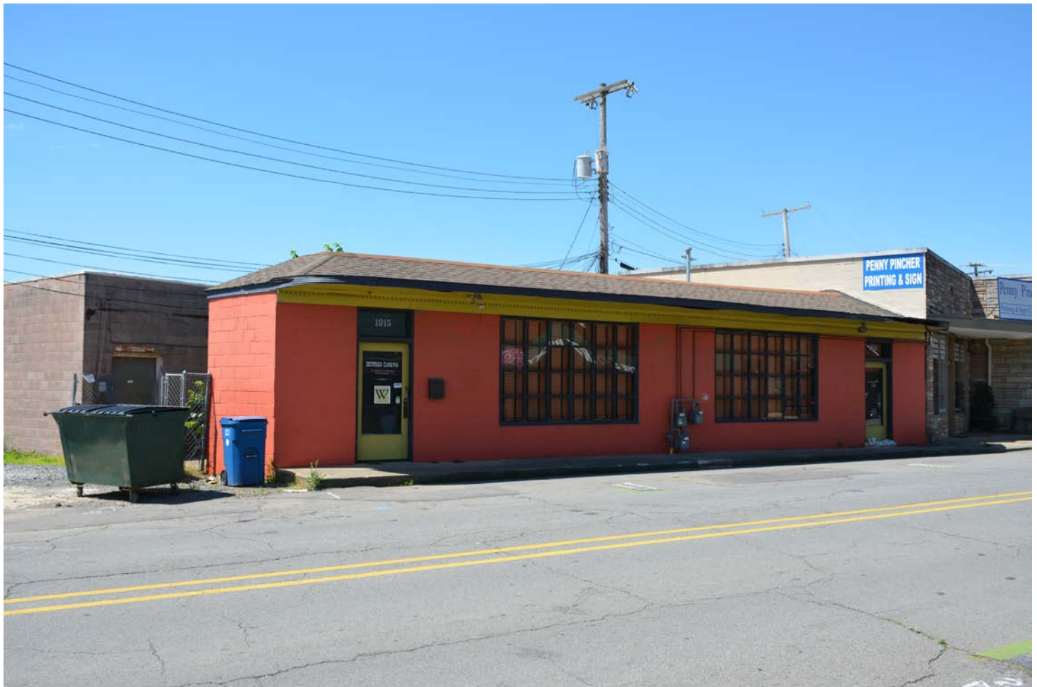
Figure 2: Current photograph of the building at 1015 Van Ronkle. (Photo date: June 2016.)
