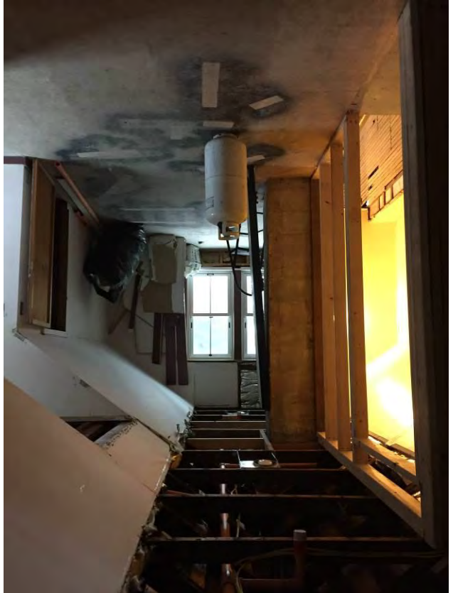
19 of 22 – Bush House, Third floor – view north.
