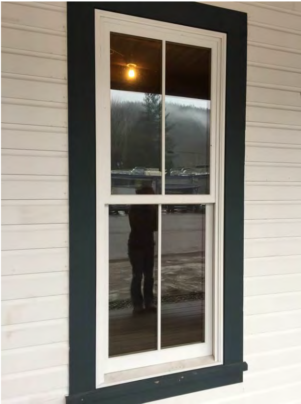
6 of 22 – Bush House, Window detail.
