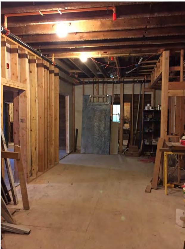
13 of 22 – Bush House, Kitchen – view looking south.
