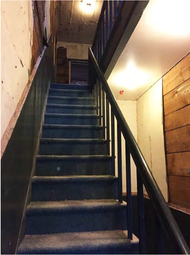
14 of 22 – Bush House, Main Stair from first floor.
