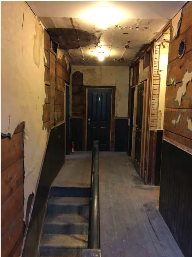
15 of 22 – Bush House, Main Stair from second floor.
