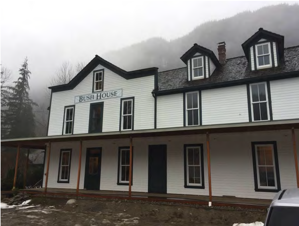
2 of 22 – Bush House, Main façade detail.
