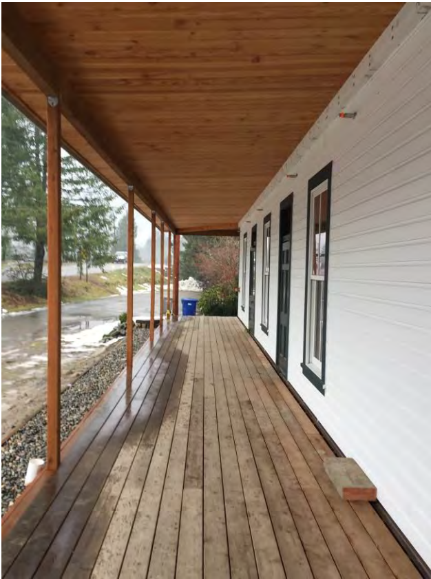
4 of 22 – Bush House, Reconstructed porch detail.
