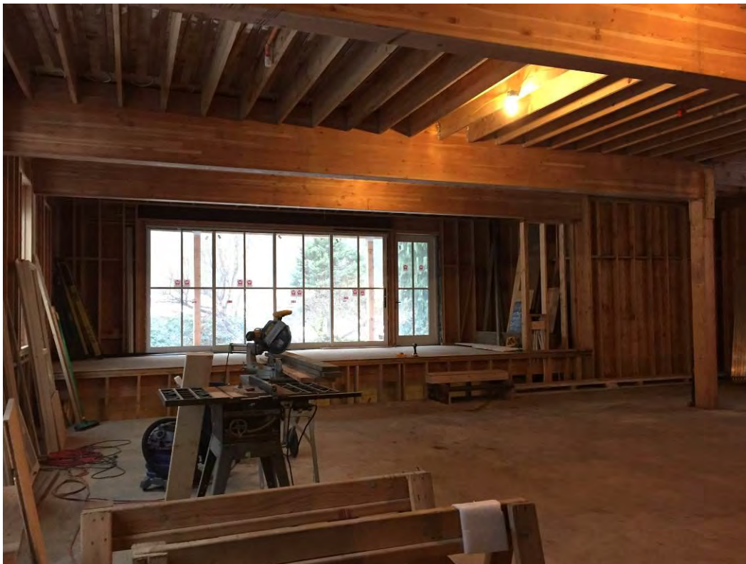
22 of 22 – Bush House, New rear wing, first floor – view west.
