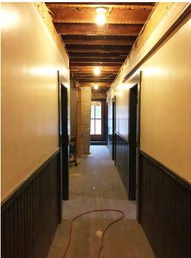
17 of 22 – Bush House, Second floor hallway – view north.
