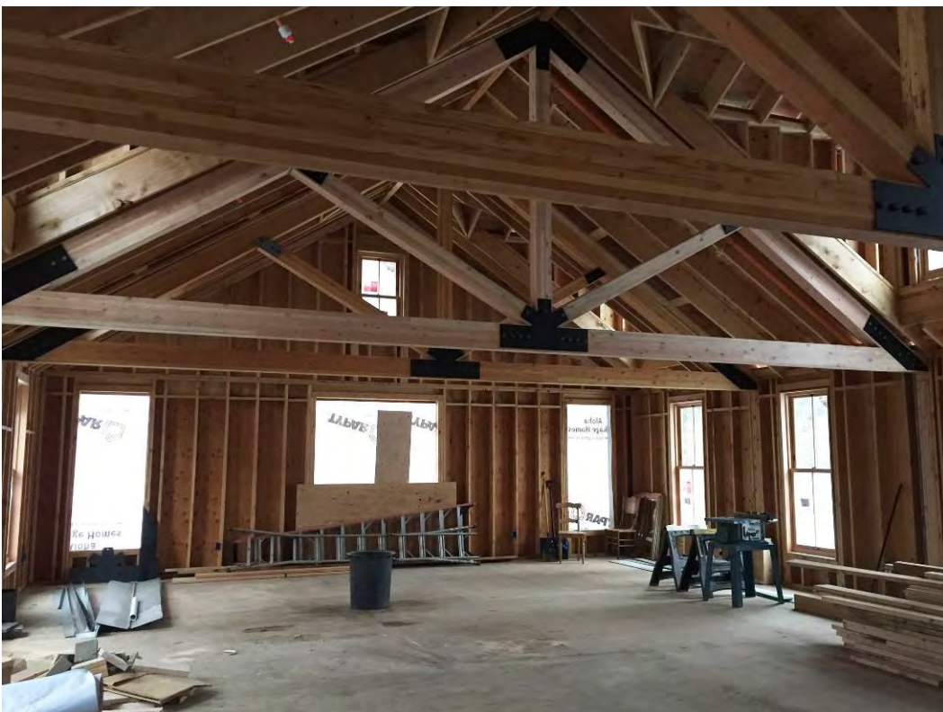
21 of 22 – Bush House, New rear wing, second floor – view west.
