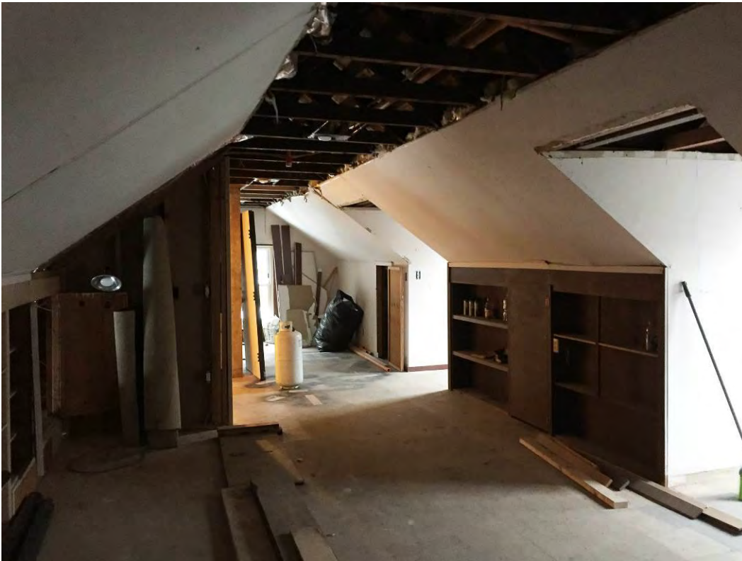
20 of 22 – Bush House, Third floor – view south.
