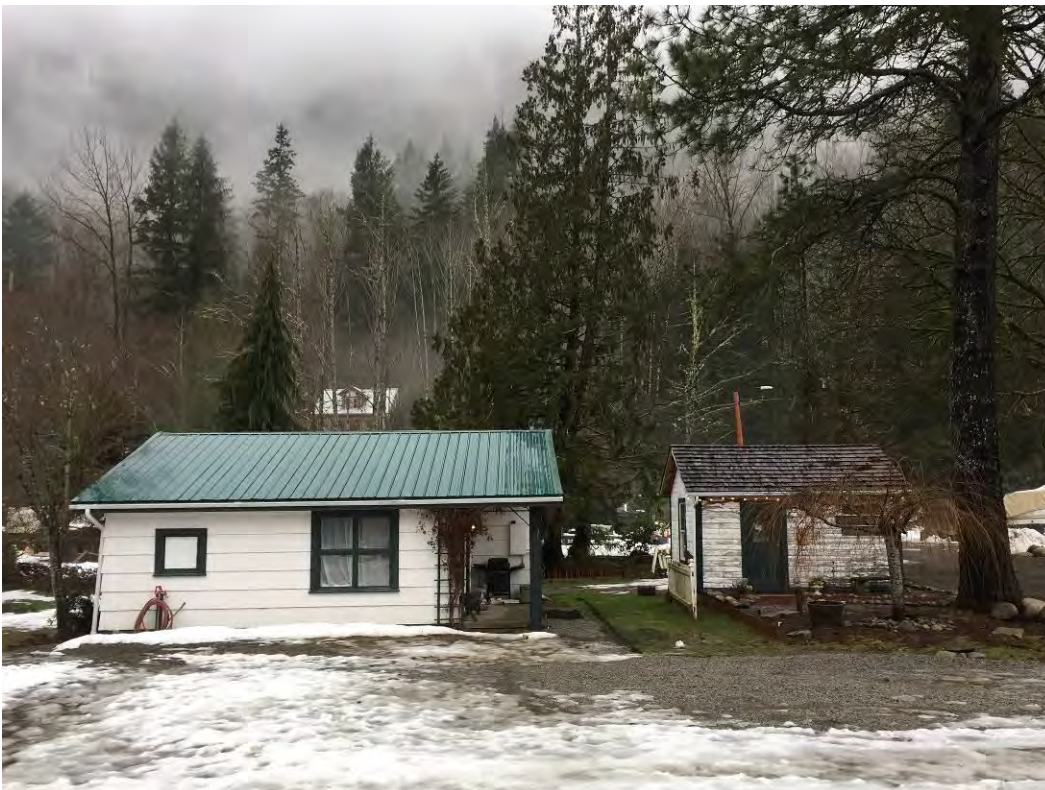
7 of 22 – Bush House, Caretakers house (left), garage (right).
