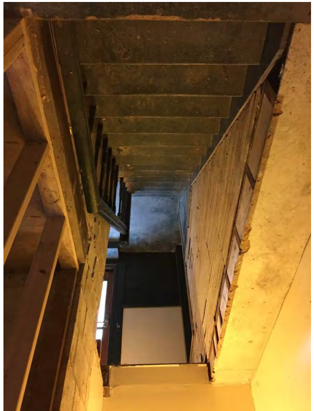
18 of 22 – Bush House, Secondary stairwell from third floor to second floor.
