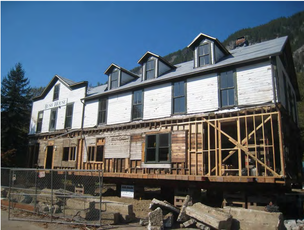
8 of 22 – Bush House, Elevated in preparation for new foundation. 2015.
