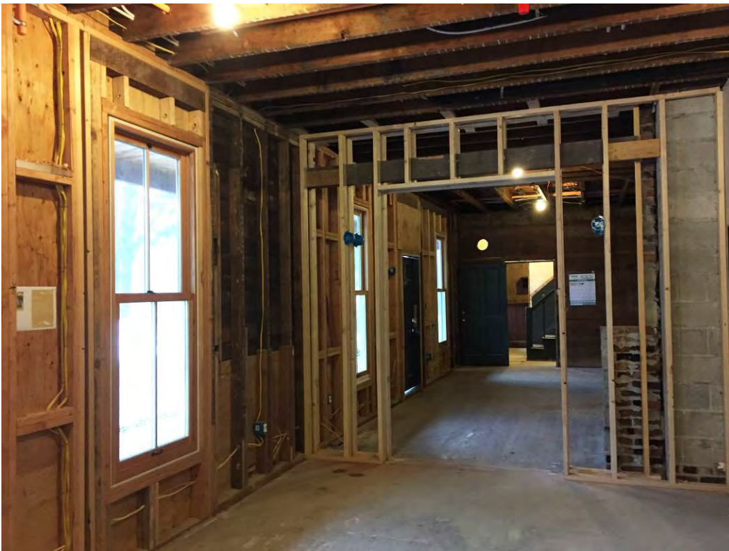
11 of 22 – Bush House, Interior dining – view looking south.
