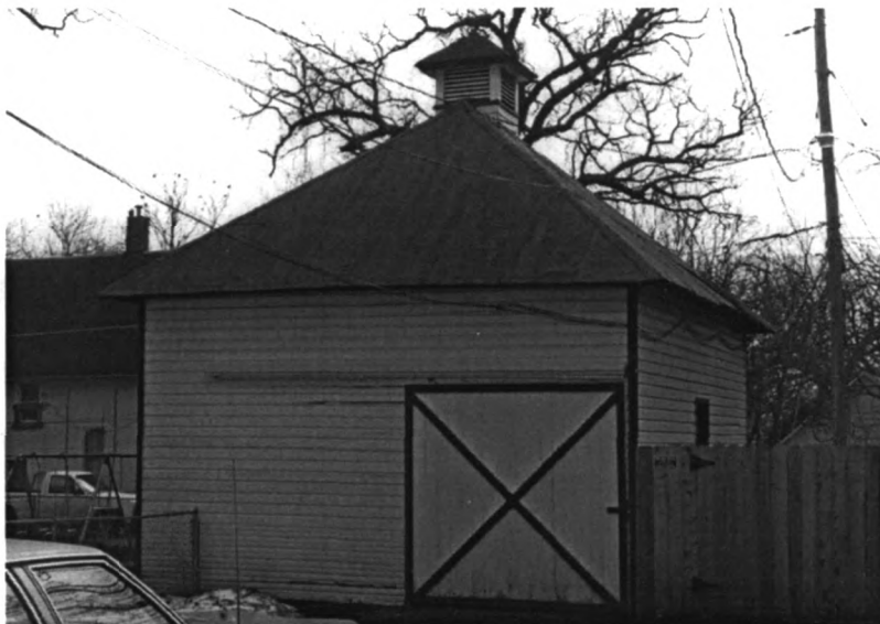
Carriage House, 2704 Cottage Grove Avenue (1908) (photo by James Jacobsen, February 23, 2000)
