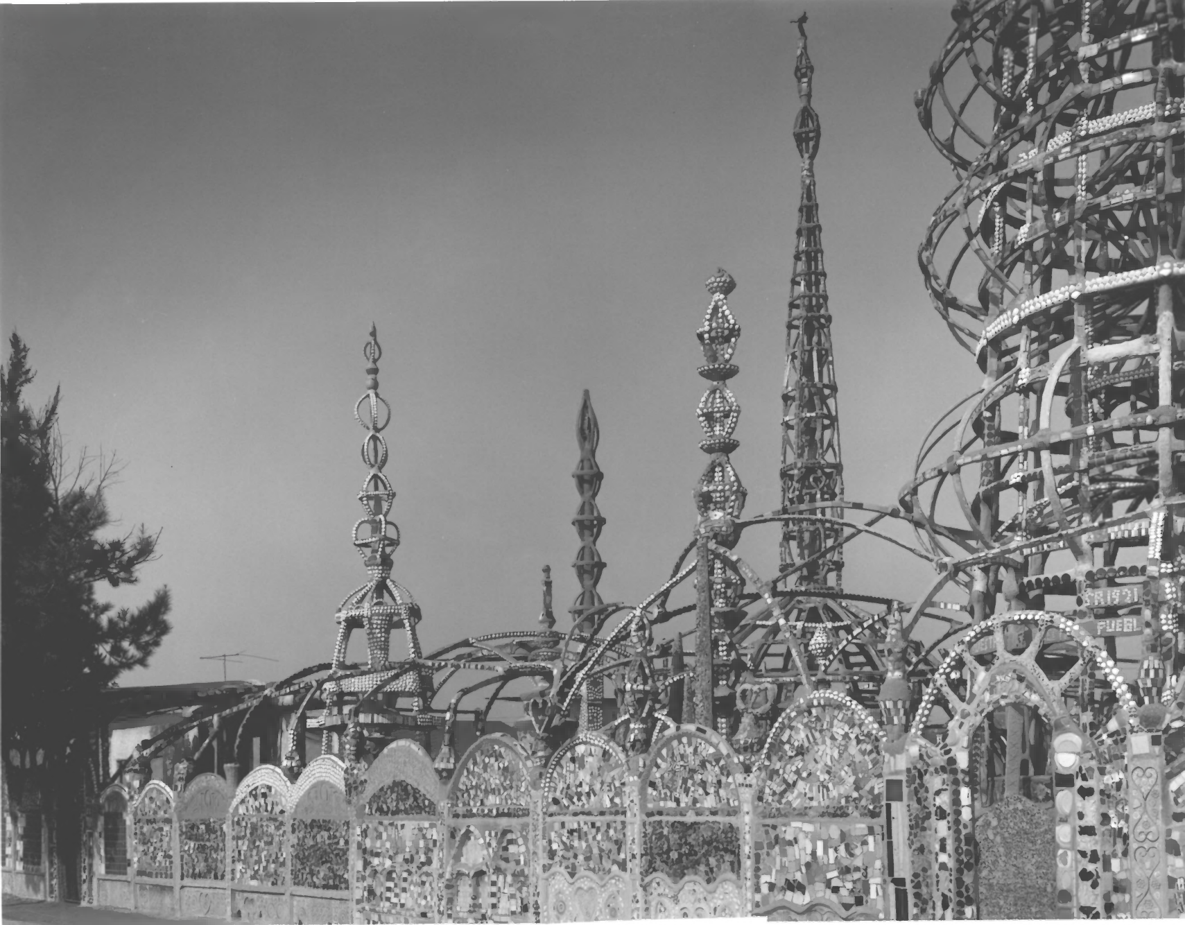
Towers of Simon Rodia, Watts, Ca View showing entrance Photo: Marvin Rand, 1989
