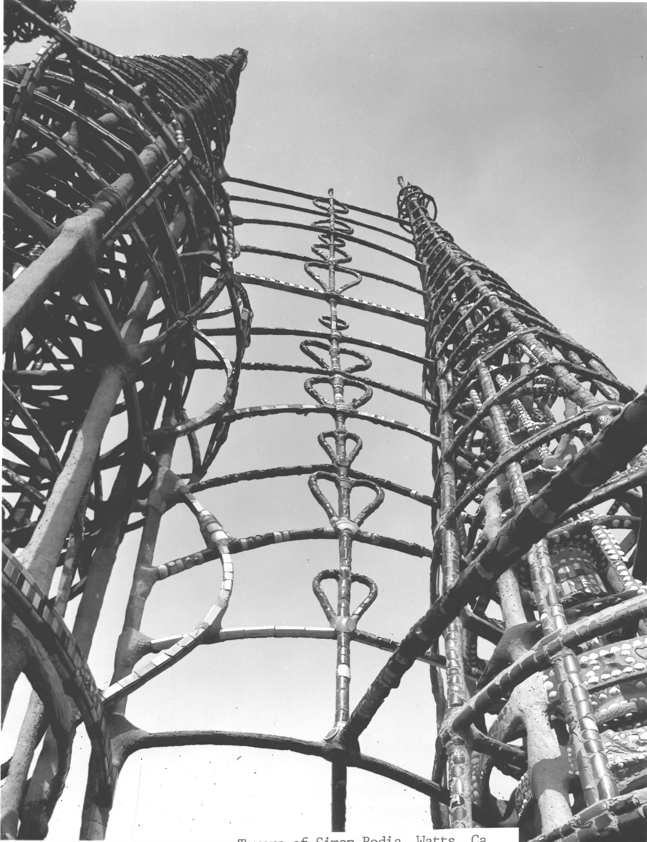
Towers of Simon Rodia, Watts, Ca Detail: Iron buttresses Photo: Marvin Rand, 1989
