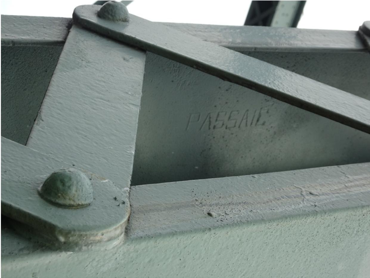
**Photograph 7.** View of Passaic Rolling Mill Company founder's mark on steel beam.
