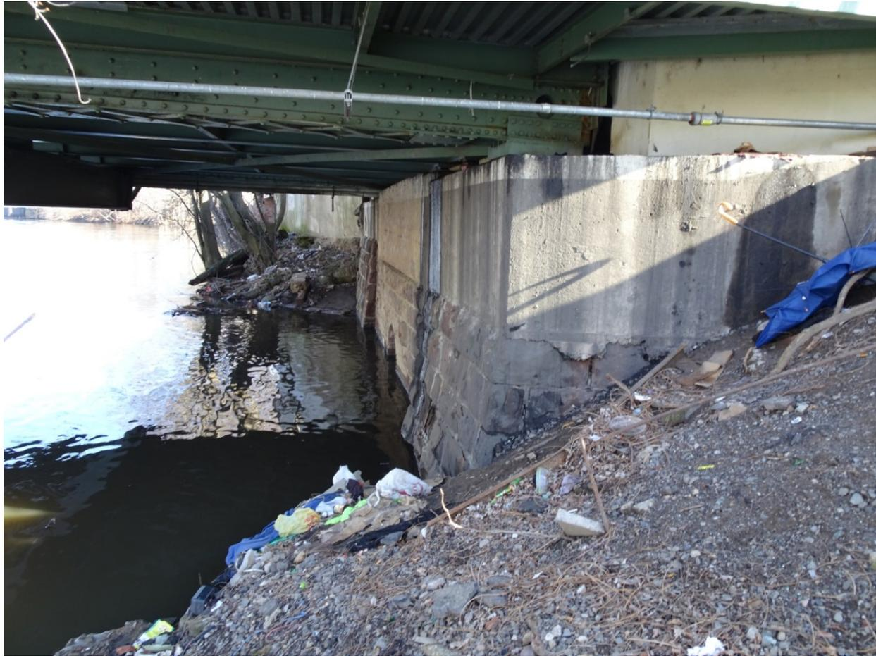
**Photograph 14.** View of south abutment with masonry of earlier span below and reinforced concrete above, looking northeast.
