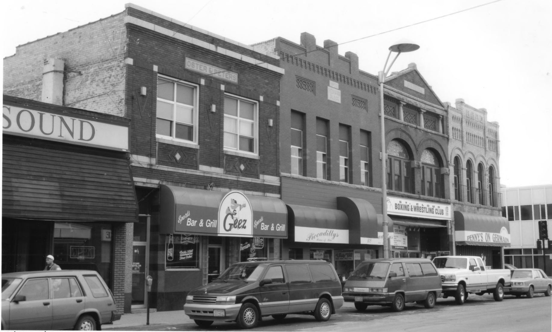
Streetscape, north side of 800 Block of St. Germain Street St. Cloud Commercial Historic District Stearns Co., MN
