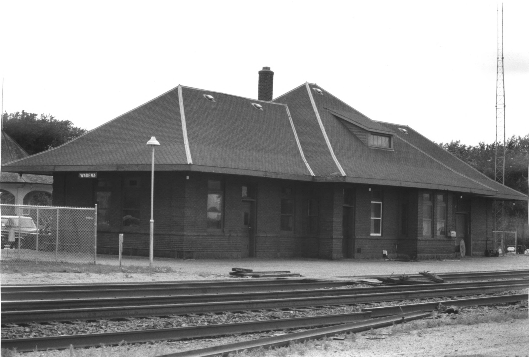
NORTHERN PACIFIC PASSENGER DEPOT WADENA, WADENA CO., MN 09326, #22
