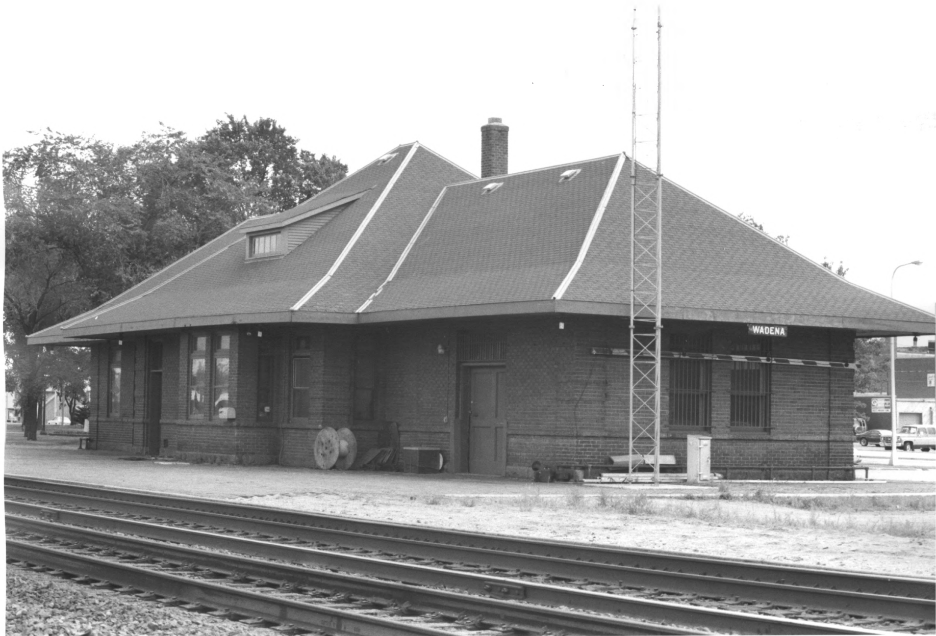
NORTHERN PACIFIC PASSENGER DEPOT WADENA, WADENA CO., MN
