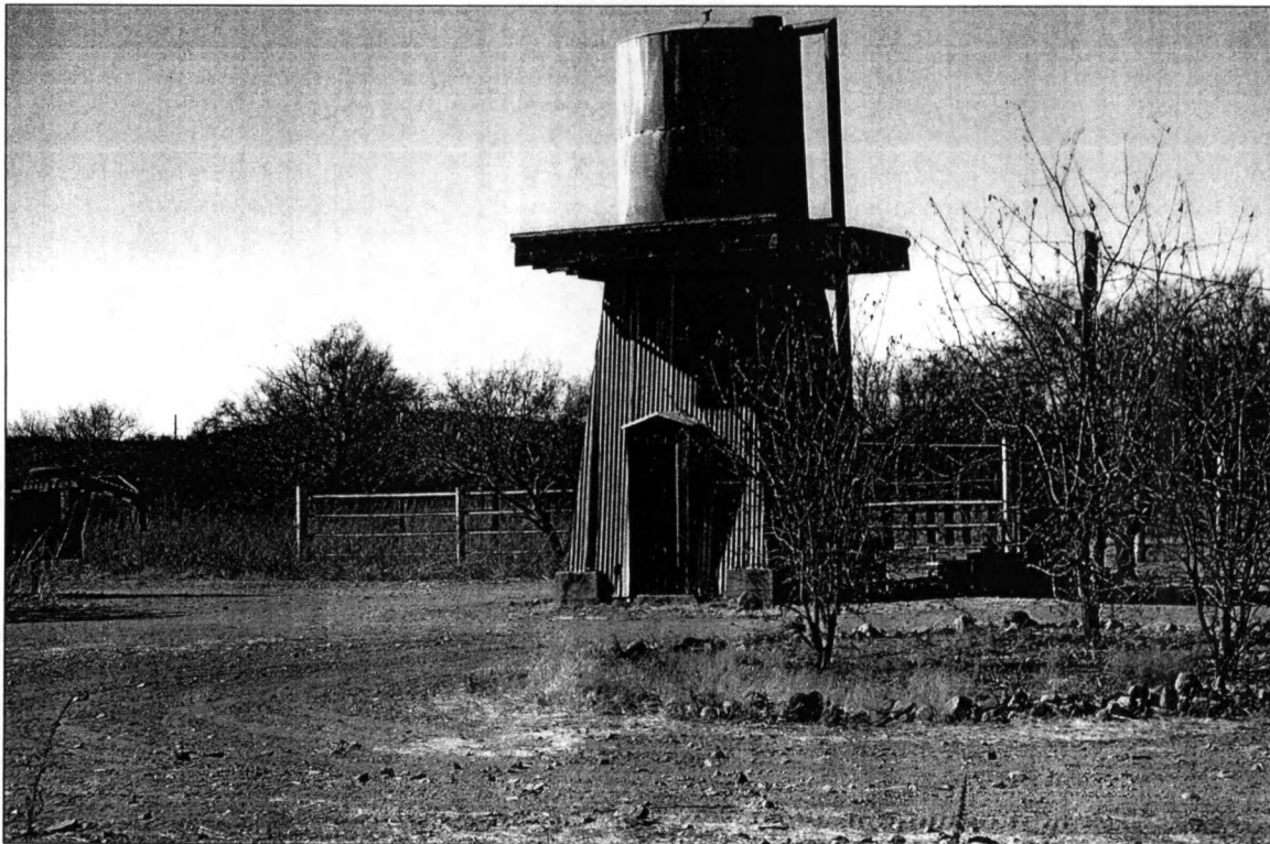
Figure 32. Wash house with rooftop water tank, South Residential Cluster, camera facing west.
