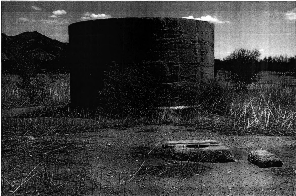
Figure 39. Concrete water-storage tank and well head, located east of Santa Cruz River, near center of agricultural zone, camera facing east.
