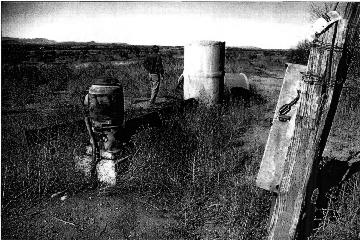
Figure 40. Well head, electric pump, and cylindrical gate box, located east of Santa Cruz River, near center of agricultural zone, camera facing east.
