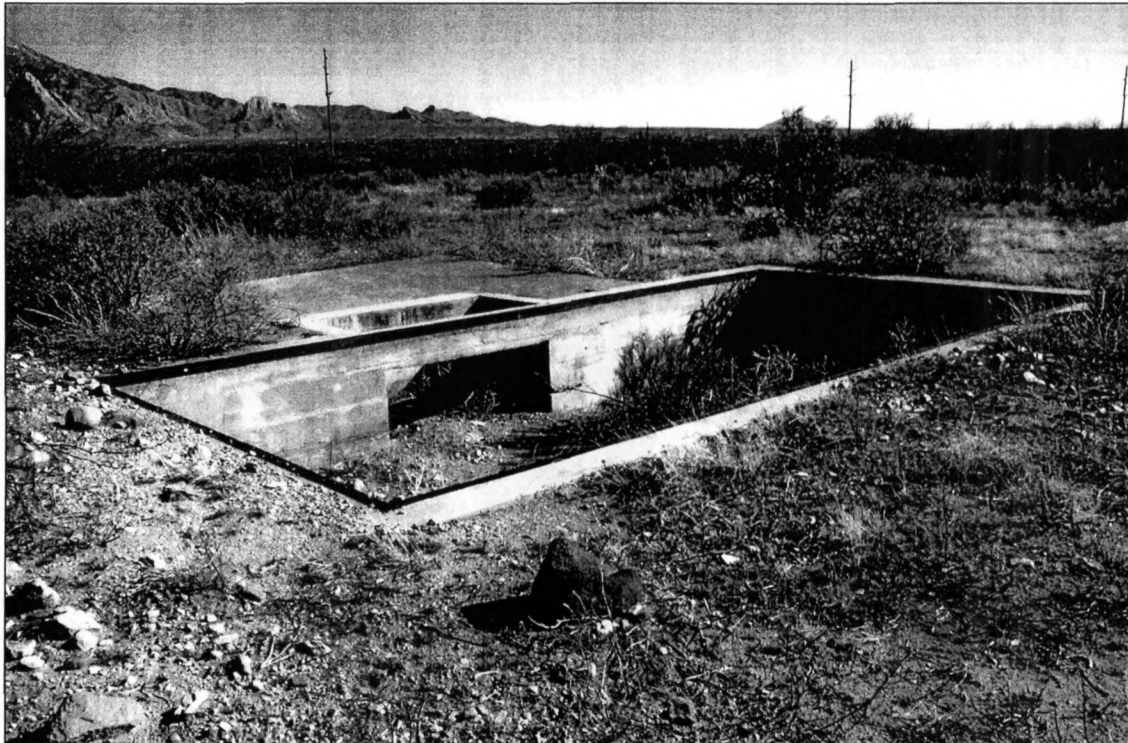
Figure 34. Truck scale foundation, Canal Head Cluster, camera facing southeast.
