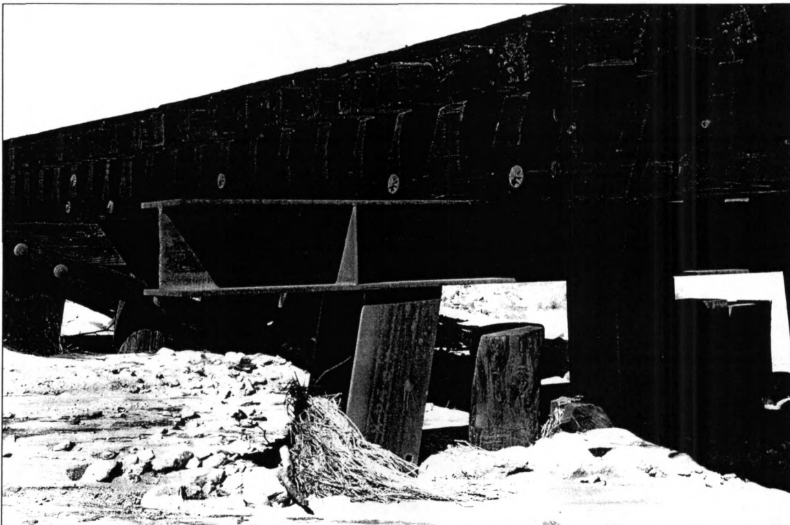
Figure 9. Wooden trestle bridge, with recent steel beam repair, on the Canoa Ranch portion of the Tucson-Nogales Railroad.
