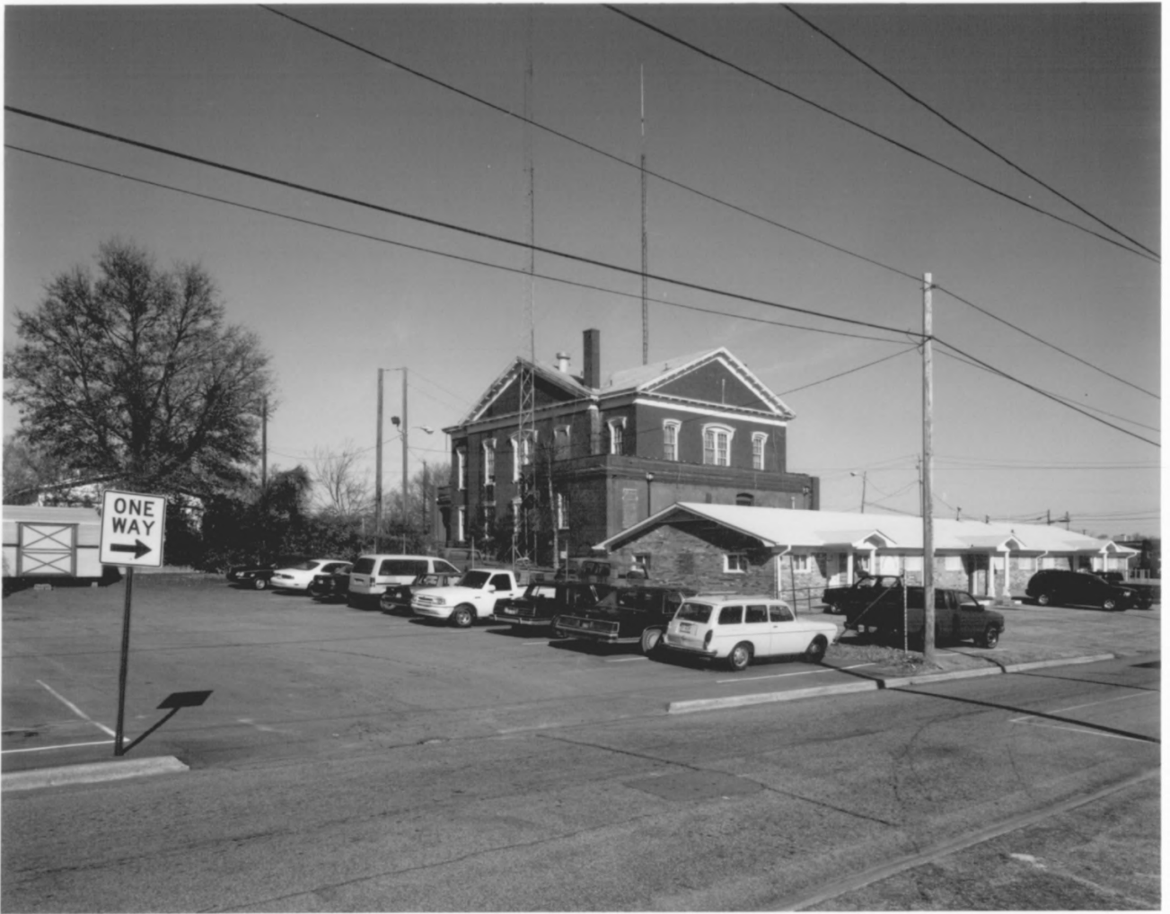
SPALDING COUNTY COURTHOUSE / SPALDING COUNTY JAIL GRIFFIN, SPALDING COUNTY, GEORGIA PHOTOGRAPH 6 OF 17
