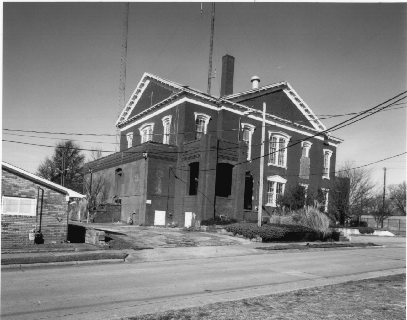
SPALDING COUNTY COURTHOUSE / SPALDING COUNTY JAIL GRIFFIN, SPALDING COUNTY, GEORGIA PHOTOGRAPH 7 OF 17
