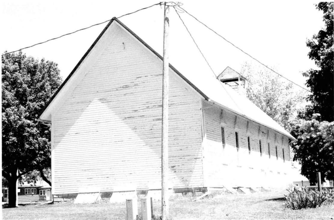
Rear (west) and south elevations looking to the northeast.
