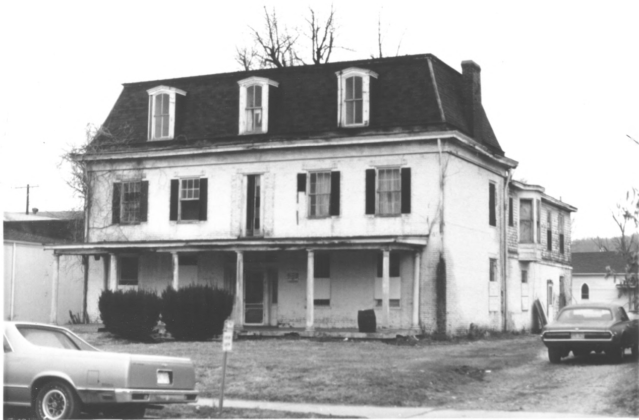
1. Shelburne - Cox House, Taylorsville, Spencer Co., Ky.
