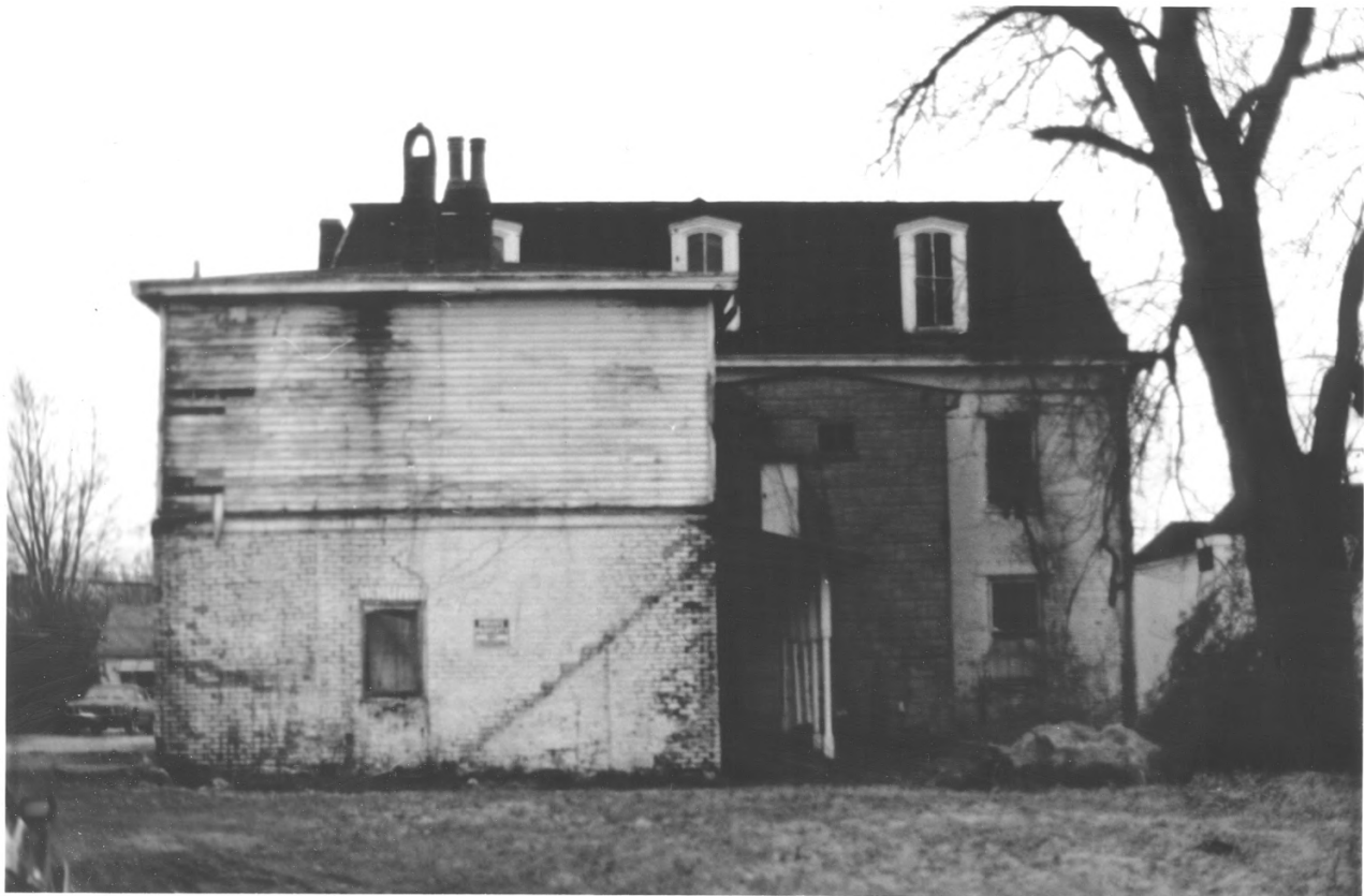
3. Shelburne - Cox House, Taylorsville, Spencer Co., Ky.
