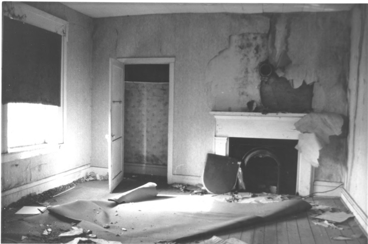
7. Shelburne - Cox House. Taylorsville, Spencer Co., Ky.
