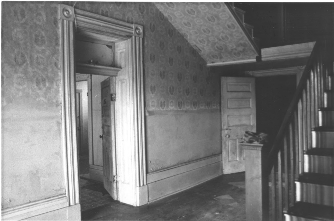
5. Shelburne - Cox House. Taylorsville, Spencer Co., Ky.
