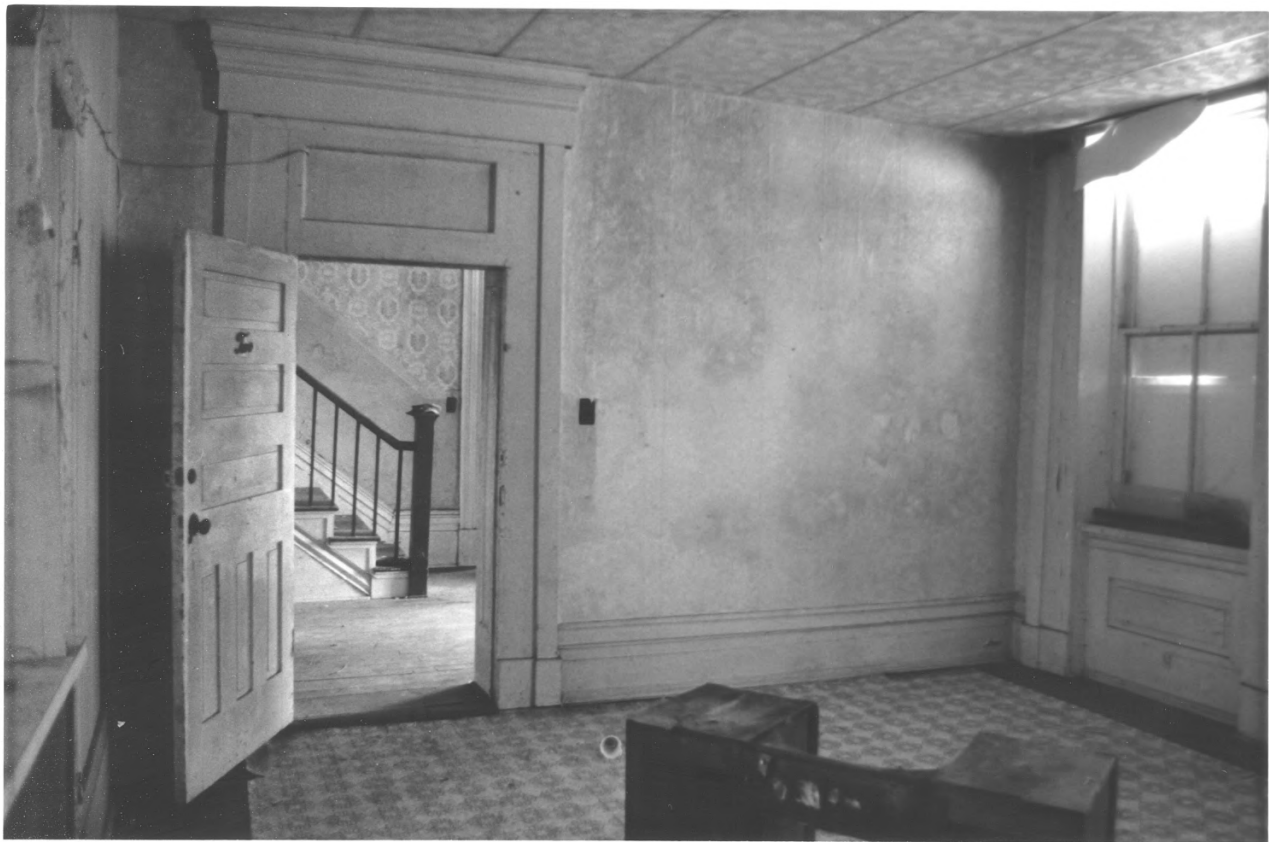
4. Shelburne - Cox House, Taylorsville, Spencer Co., Ky.
