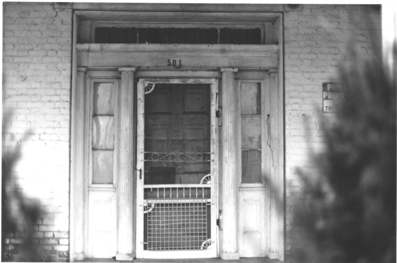
2. Shelburne - Cox House, Taylorsville, Spencer Co., Ky.
