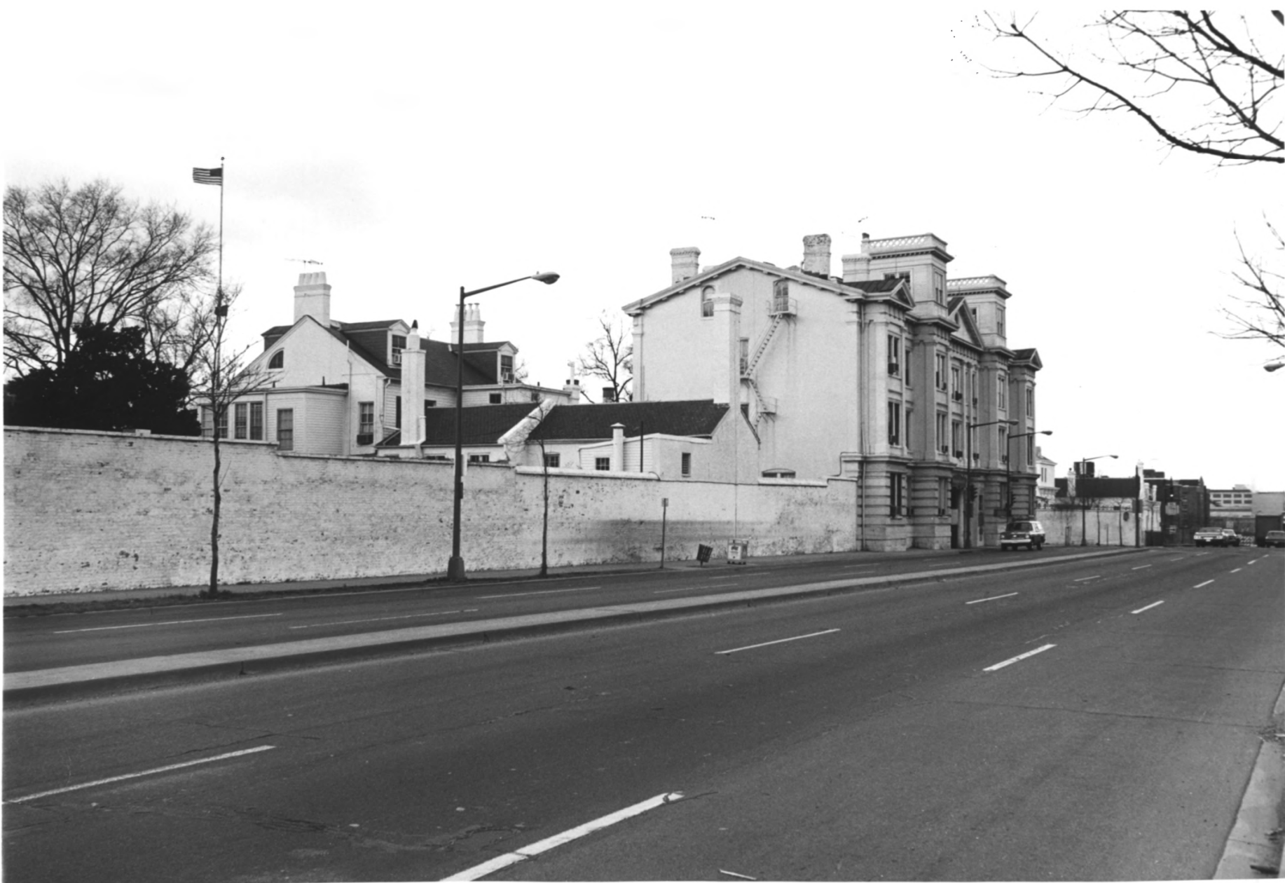
Washington Navy Yard, Washington, D.C. North wall along M Street, S E.
