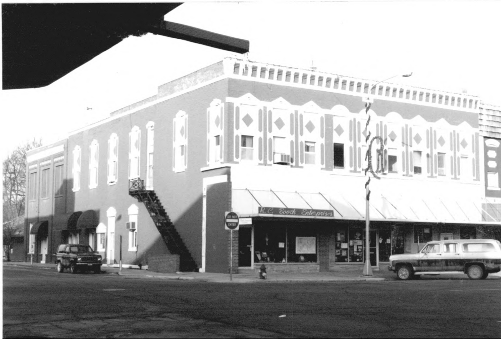
Photograph 7-11. Type III Building, Long Block (#27a-c).
